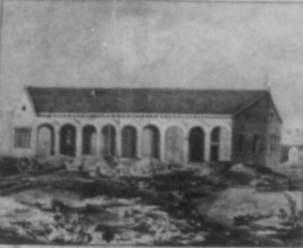
St Louis & Iron Mountain Railroad Work - Shop.
