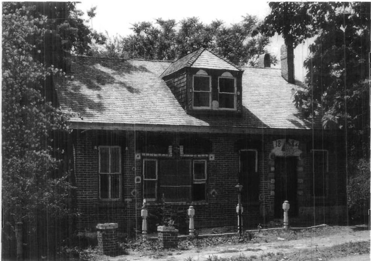
Alois Herbert Double House, May 21, 2006 – WORK IN PROGRESS
