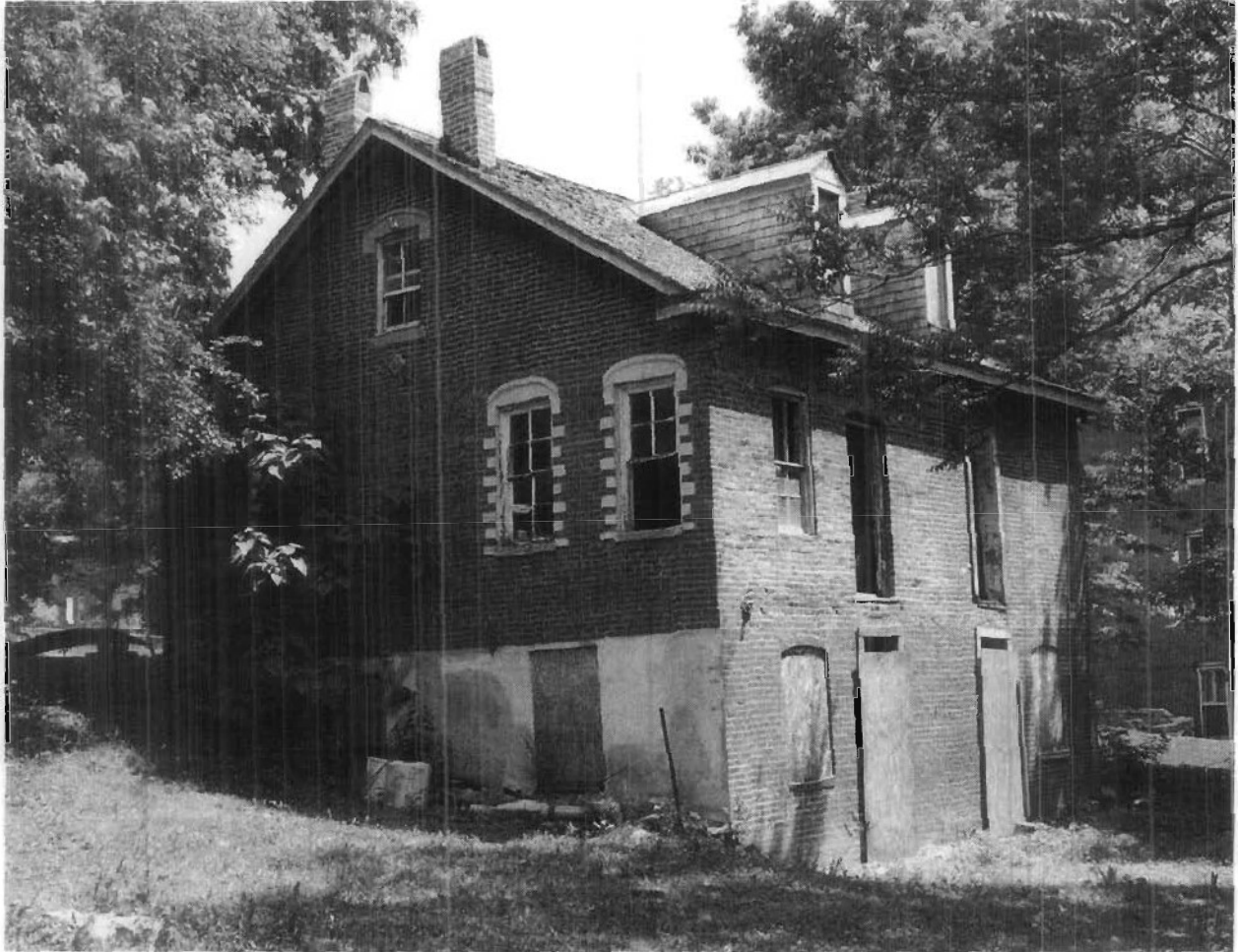
Alois Herbert Double House, May 21, 2006 -- WORK IN PROGRESS
