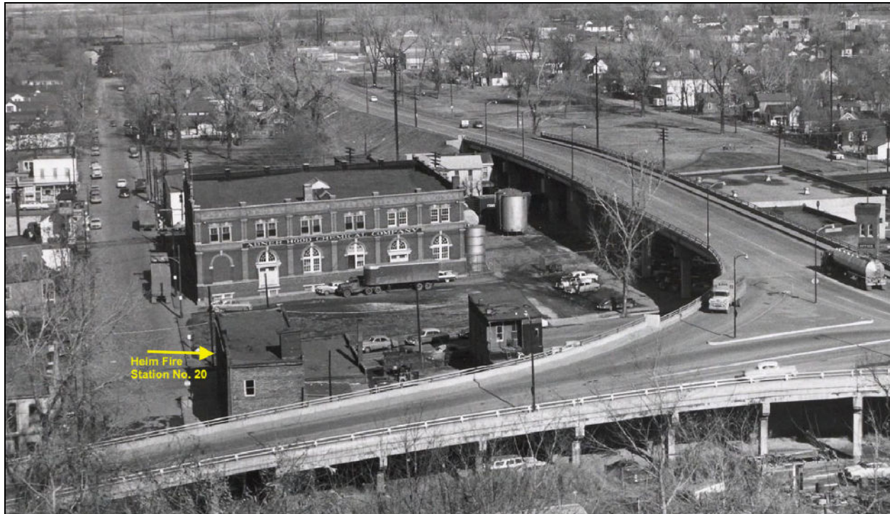
Figure 9: Rear elevation of Heim Fire Station No. 20, as it appeared c. 1960.
