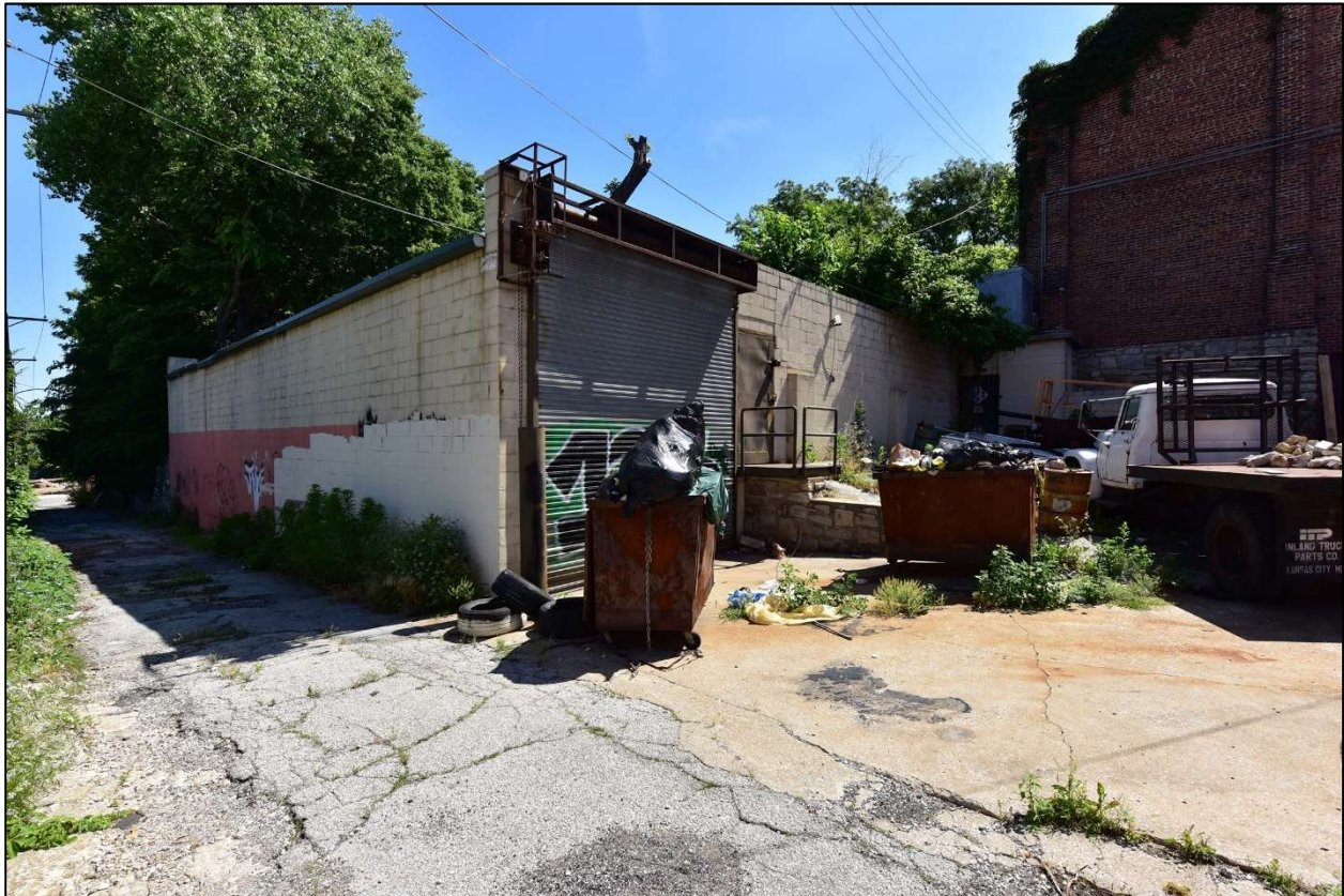
Figure 6. South façade of adjacent garage and CMU retaining wall on property to the north of the Hazelle Building. Source: Brad Finch, June 2020.
