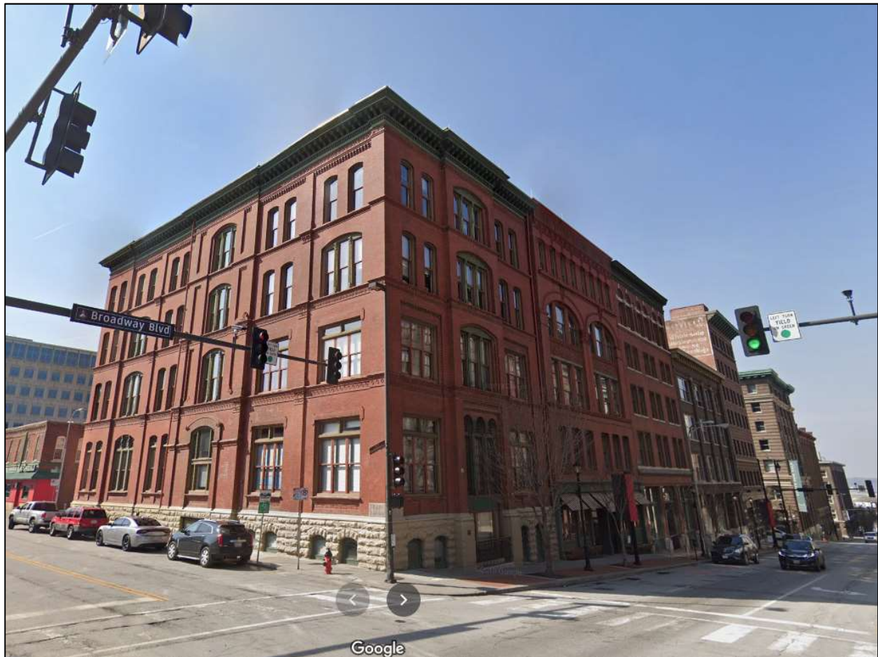
Figure 27. The extant Thayer (Bracken) Building, 820-822 Broadway, looking northwest at its south and east elevations. Source: Google Streetview, image date April 2019.
