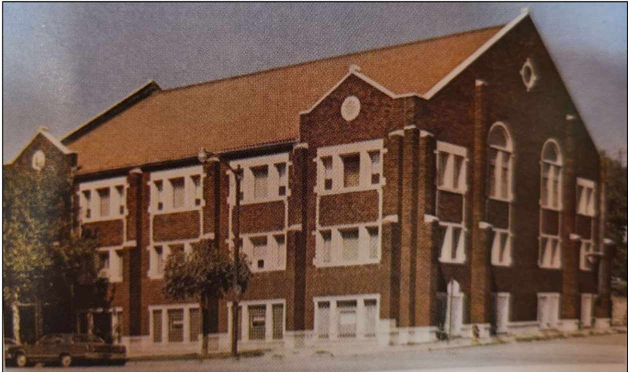
Figure 9. The building at 1224 Admiral Blvd. in 1971 while occupied by Hazelle, Inc. View is to the northwest. Note glass block at ground level of the main façade and center windows of the third story on the east elevation. Source: Joly, Hazelle & Her Marionettes , 89.
