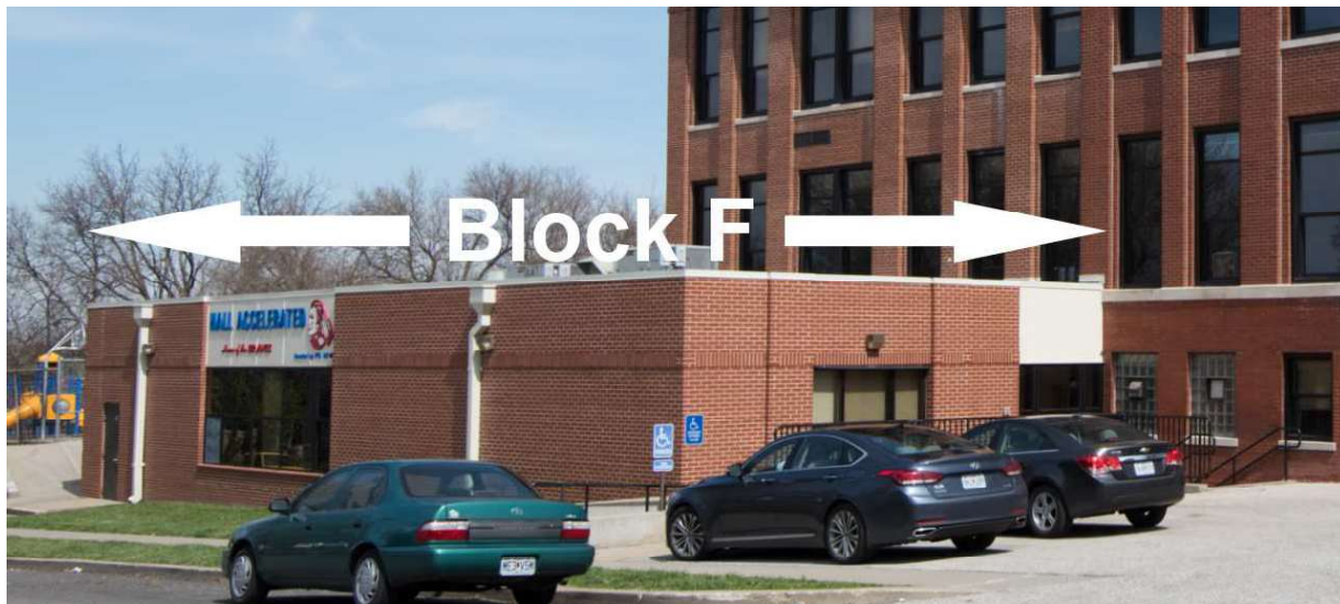
Figure 16. Hall School Block F, south and west elevations. Source: Brad Finch, 2016.
