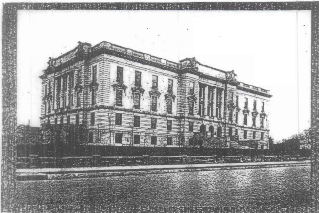
No. 1.—Greene County Court House, Built of Missouri Marble at a cost of $400,000.
