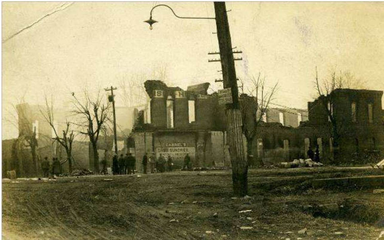
Figure 15. Madison Hotel after the fire of 1911. The hotel re-located to a new building constructed in 1915 on northwest corner of the court square. Photo is courtesy of Vi Thompson. Available online at: http://www.rootsweb.ancestry.com/~momadiso/around_madison/around_madisonco11.html .
