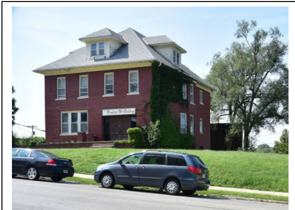
Figure 24. 1002 North 24 th Street 2019.
