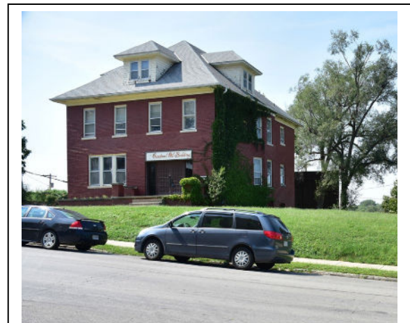
Figure 47. 1002 North 24 th Street, 2019.
