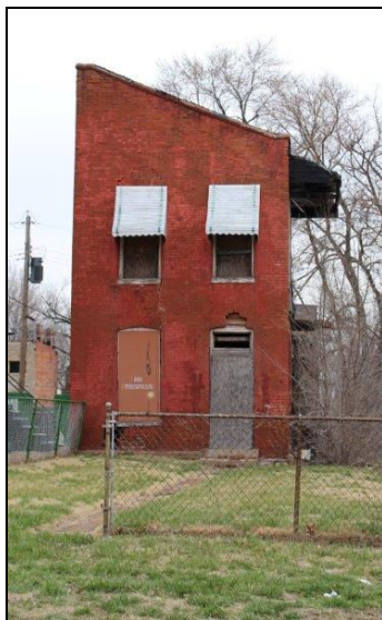
2729 Howard Street The gallery roof remains
