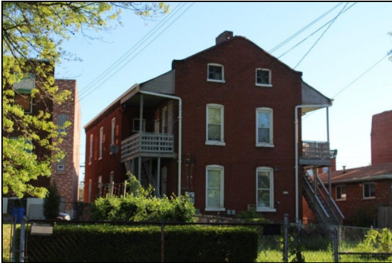
Rear wing galleries at 2814 and 1826 Arsenal Street
