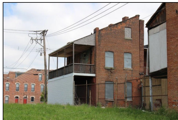
2511 Rear Benton Street
