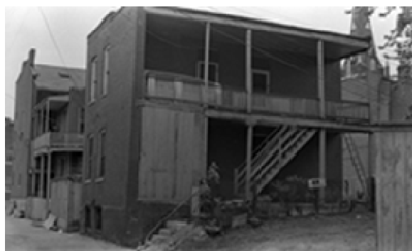
Figure 2. Gallery. This unidentified photograph taken in Soulard ca. 1870 is a Charleston House type with a side gallery (porch with internal steps) with a brick wing wall at the street end of the porch.
