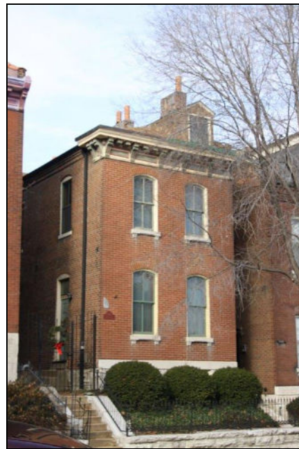
Bracketed wood cornice 2307 S. 11 th Street
