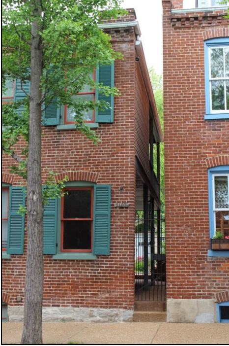
Typical brick wing wall in front of gallery, 2107 Menard Street
