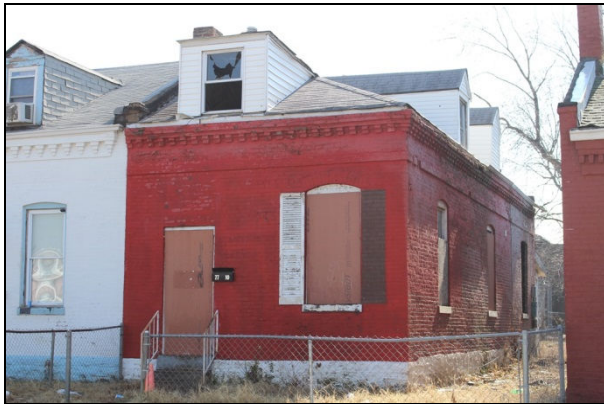
Brick cornice 7710 Water Street
