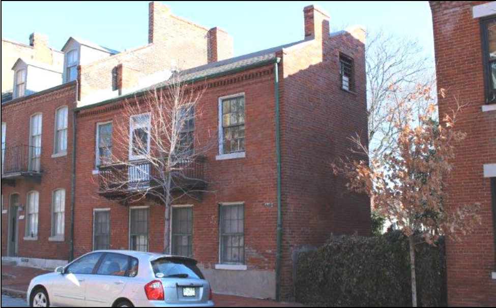
Shed roof only, 1812 S. 8 th Street
