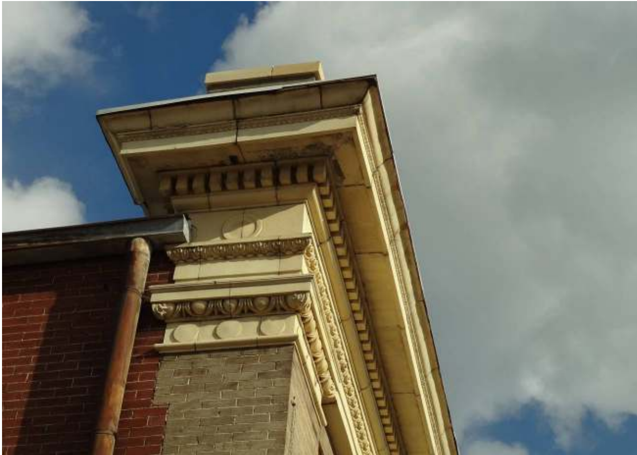
Photo 4. Northwest corner—terra cotta cornice.
