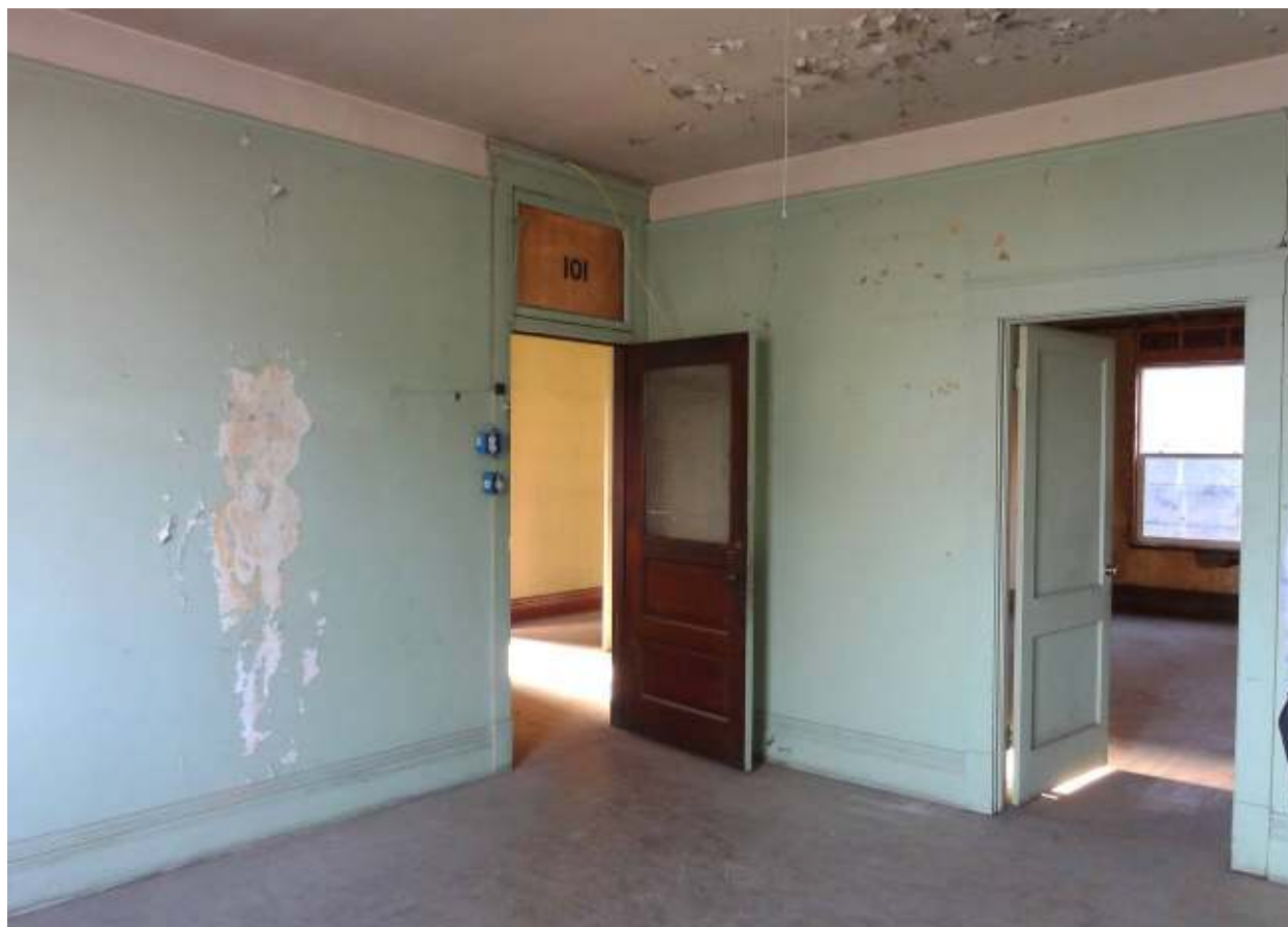
Photo 9. Second floor, front office.
