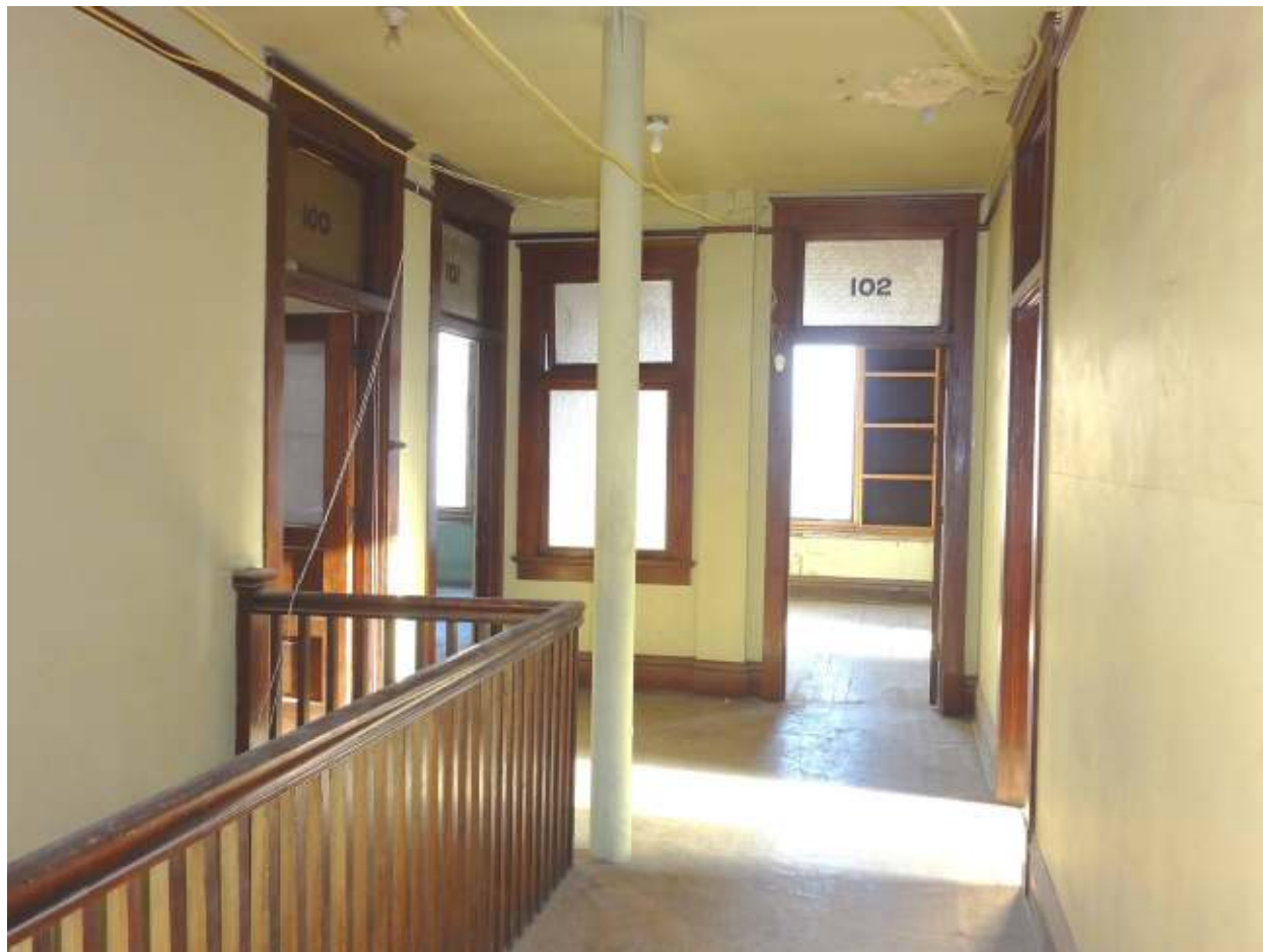
Photo 10. Second floor, south end of hallway.
