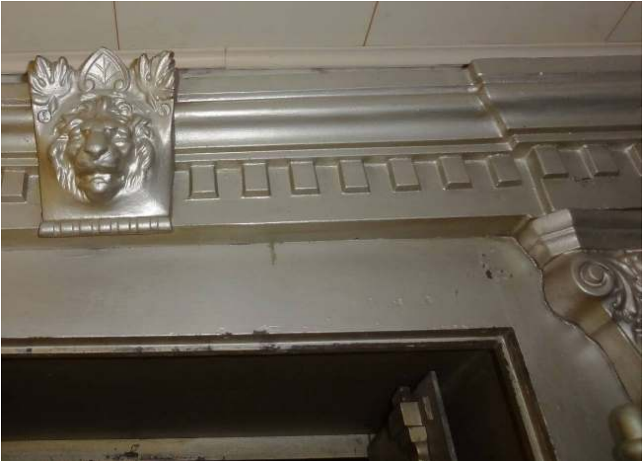
Photo 14. First floor, west side, original bank safe.
