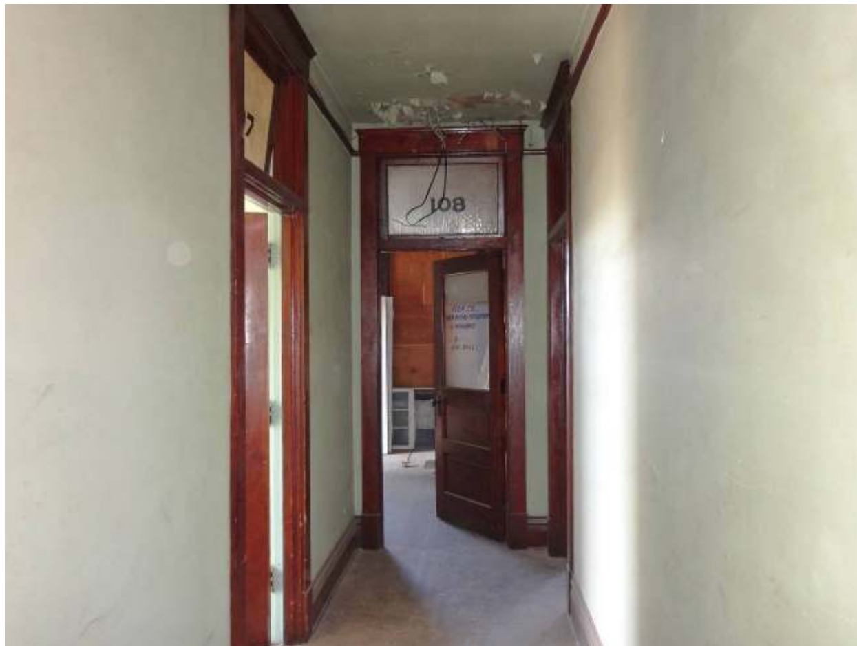
Photo 8. Second floor, north end of hallway.
