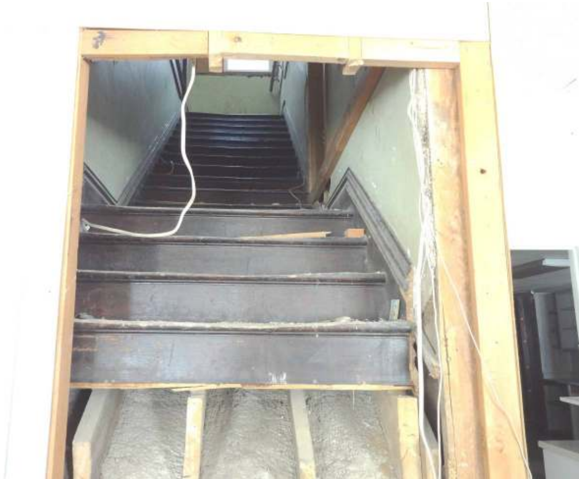
Photo 11. First floor, remaining original stairs to second.
