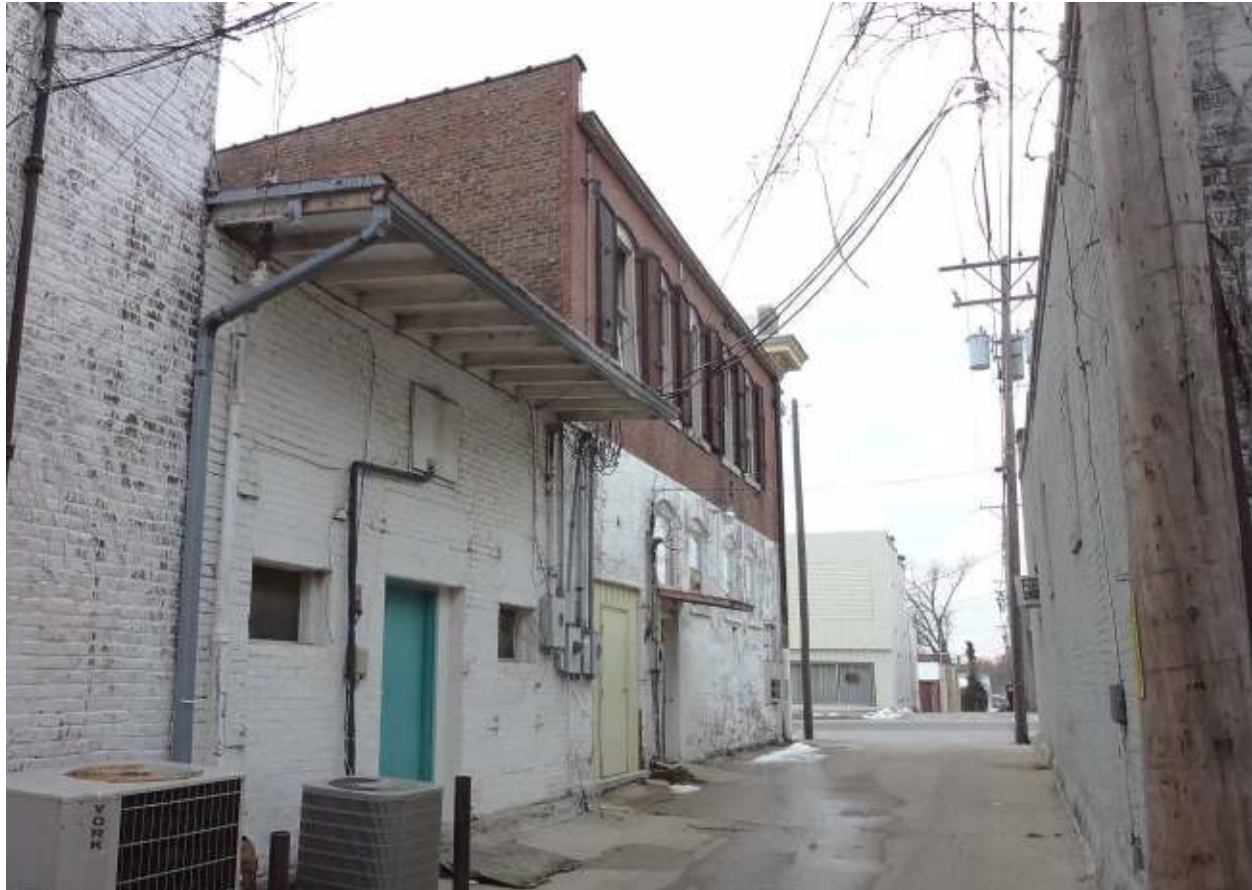
Photo 6. North (back) wall, from the east.
