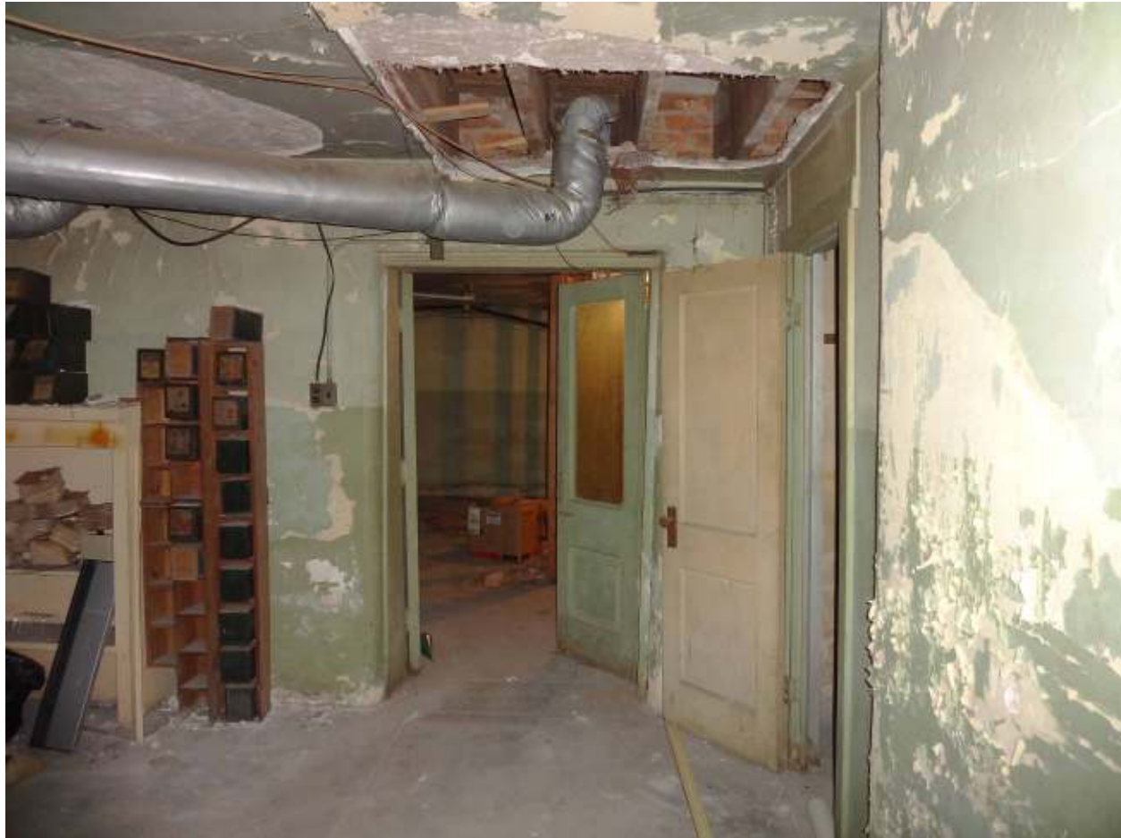
Photo 16. Basement, south end.
