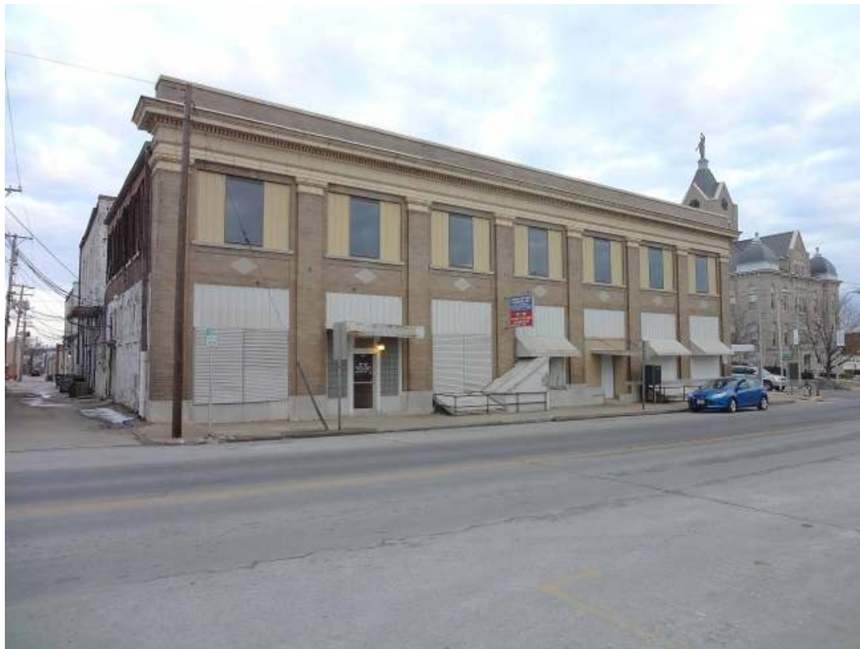
Photo 5. West wall and northwest corner.
