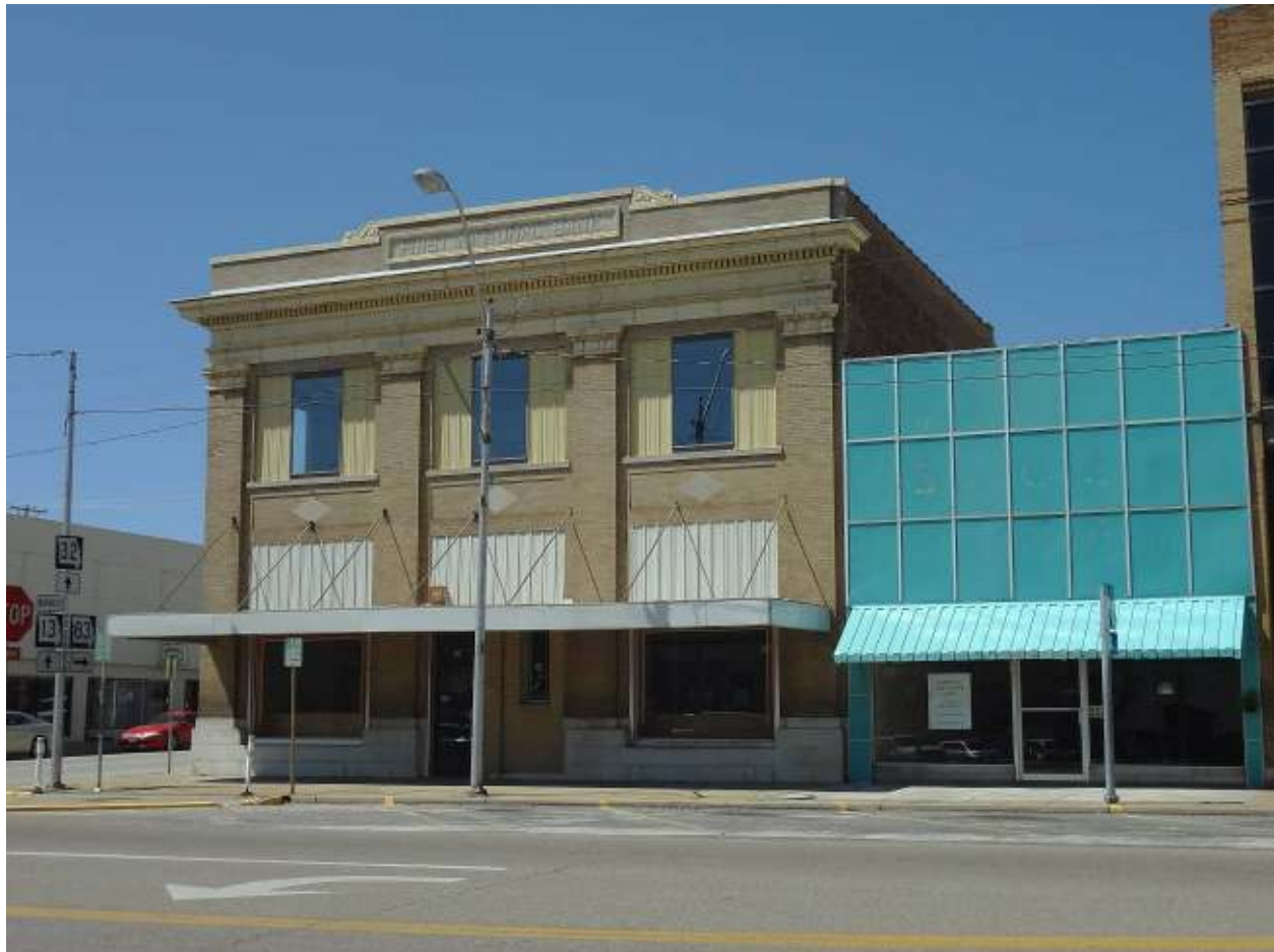
Photo 2. Façade, south wall.
