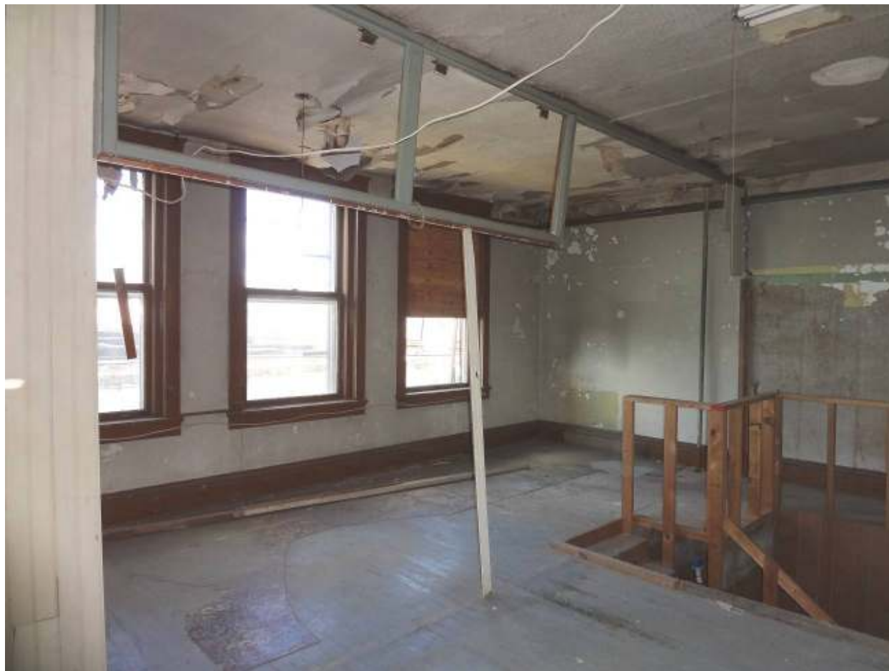
Photo 7. Second floor, back wall.
