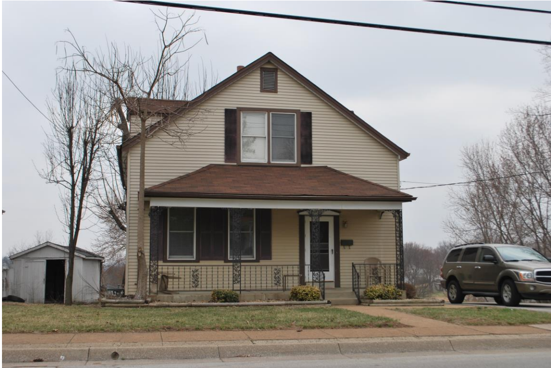
Figure 19. 1013 W. Fifth Street, view is north.
