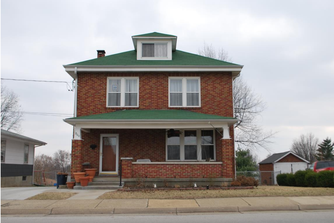
Figure 25. 806 W. Fifth Street, a Foursquare dwelling, view is south.
