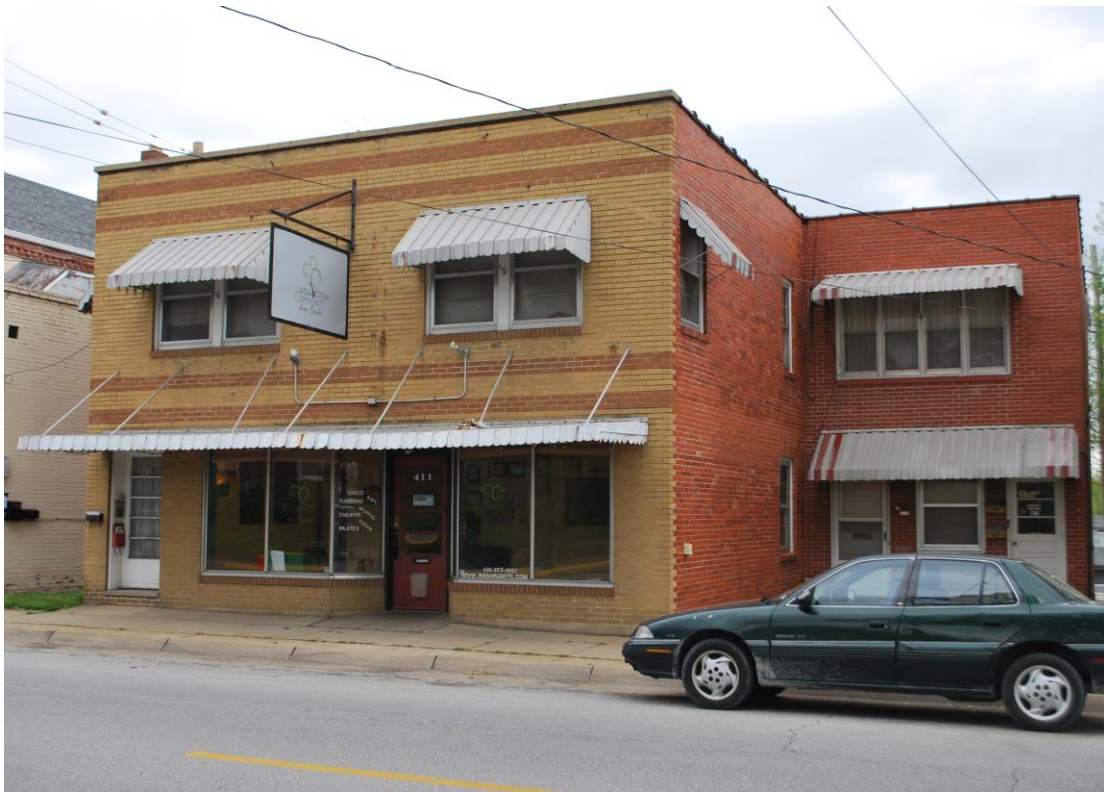
Figure 45. 409-13 W. Fifth Street is a multi-purpose commercial building. View is northwest.
