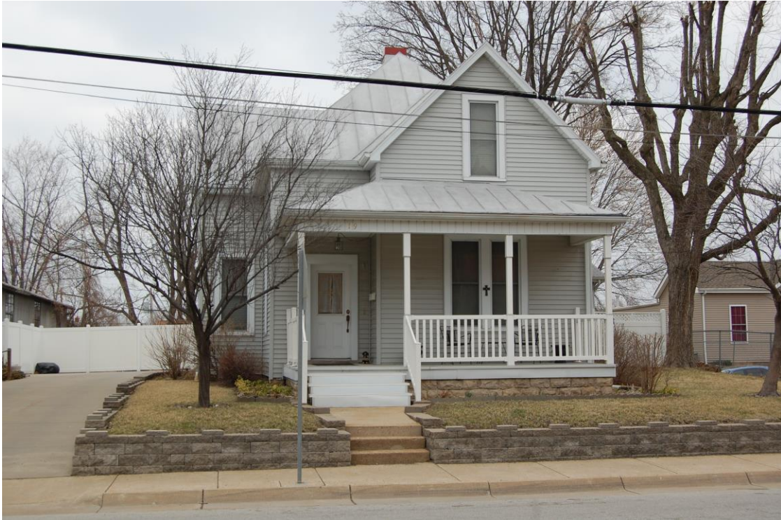
Figure 16. 19 E. Fifth Street, view is northeast.
