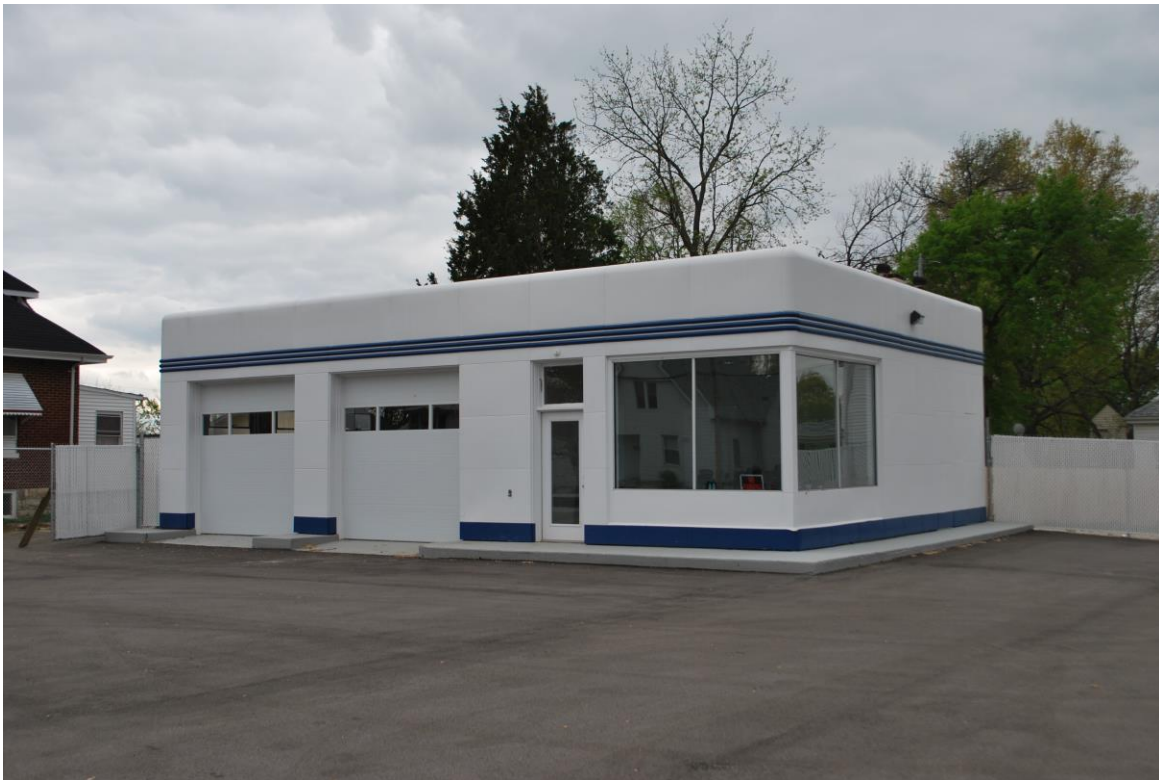
Figure 49. The former Arro Gasoline Station at 300 E. Fifth Street, view is northwest.
