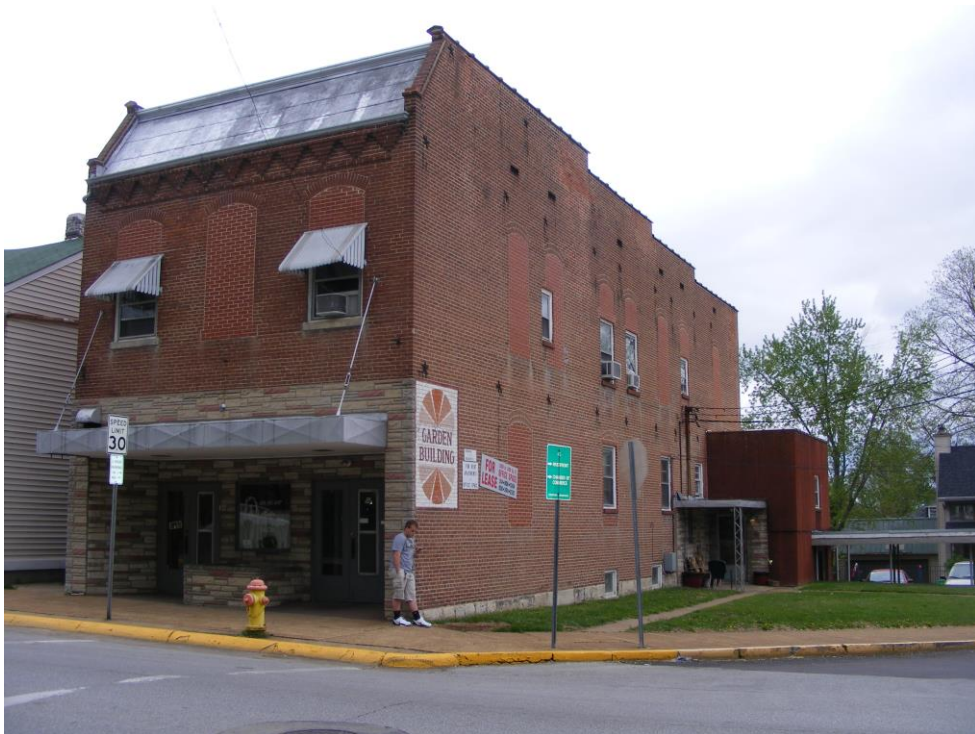
Figure 21. 401-403 W. Fifth Street, view is northwest.
