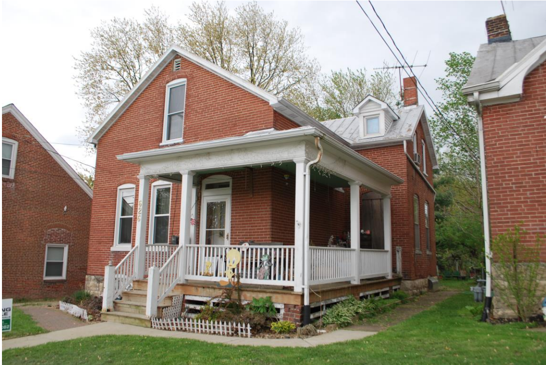
Figure 13. 626 W. Fifth Street, example of a brick Gabled Ell plan dwelling, view is southwest.
