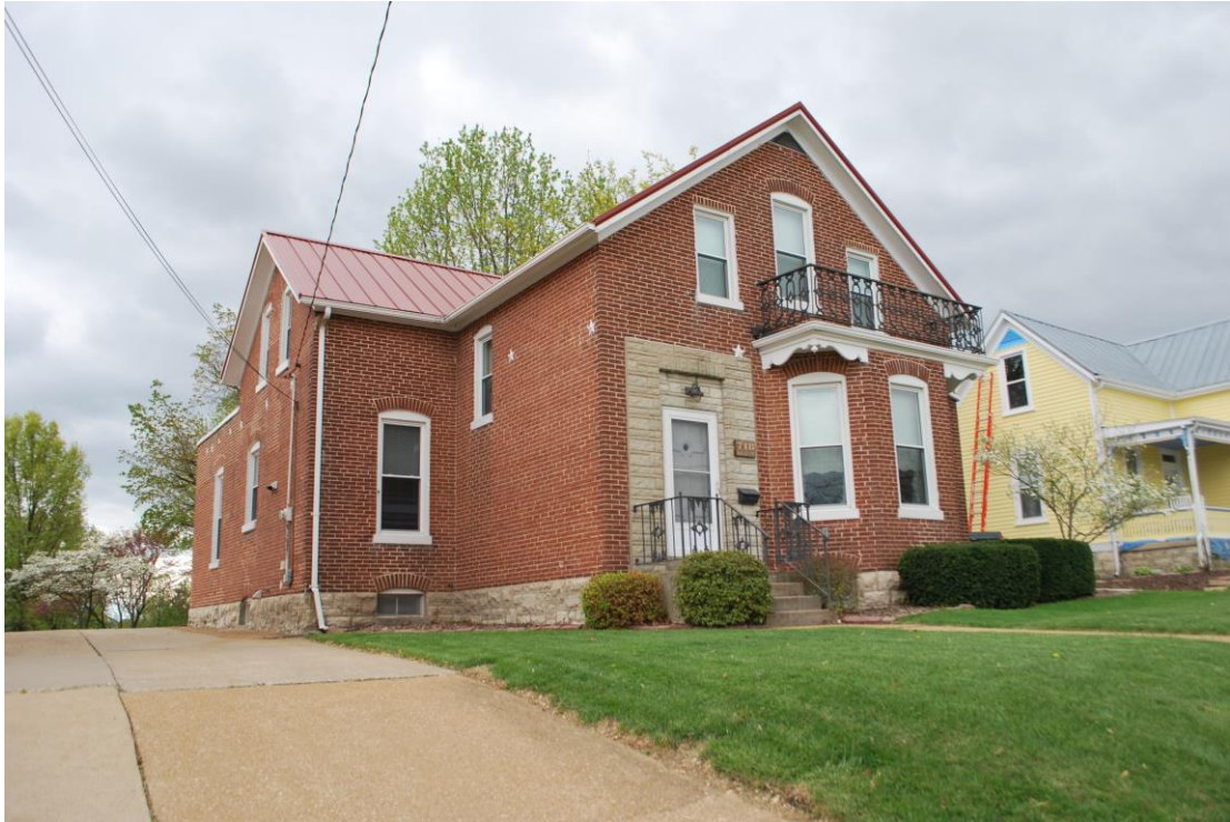
Figure 14. 718 W. Fifth Street, narrow Gabled Ell plan brick dwelling, view is southwest.
