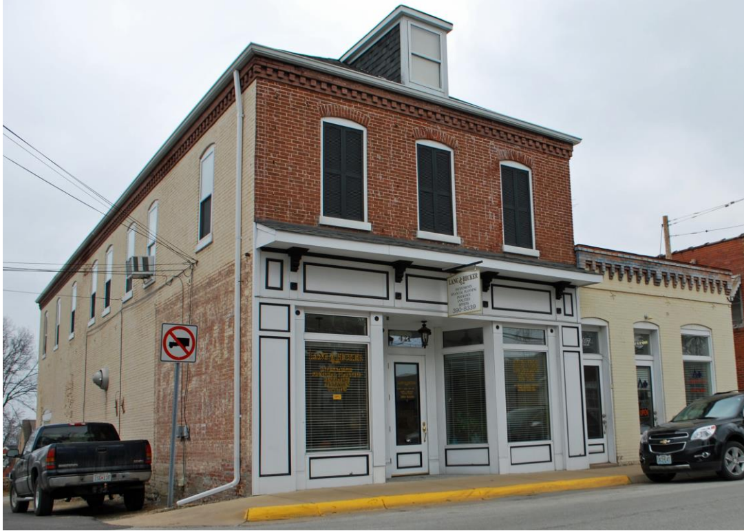
Figure 44. 421 W. Fifth Street, view is northeast.
