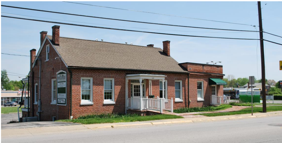
Figure 8. 529 E. Fifth Street, example of a neoclassical federal subtype dwelling, view is northeast.
