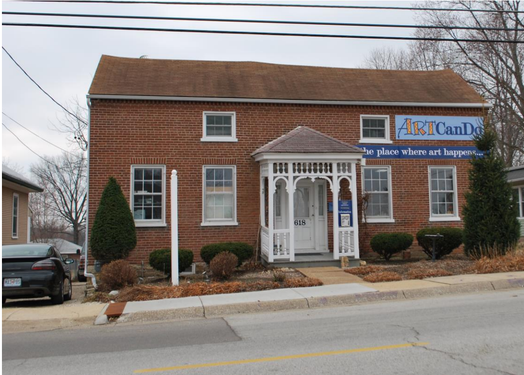
Figure 42. The Menzenworth House, 618 W. Fifth Street, view is southwest.
