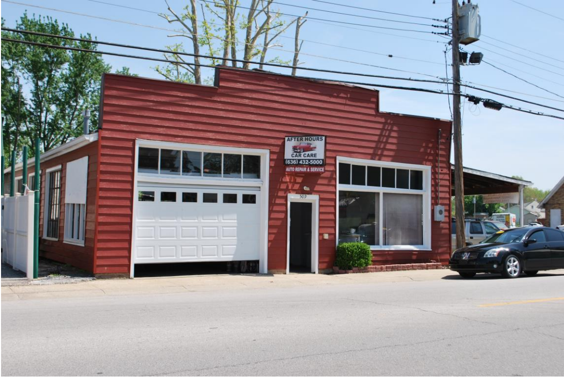
Figure 22. 509 E. Fifth Street, view is northeast.
