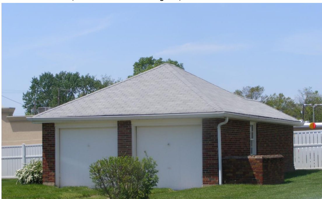
Figure 52. Garage associated with 553 E. Fifth Street. View is southwest.
