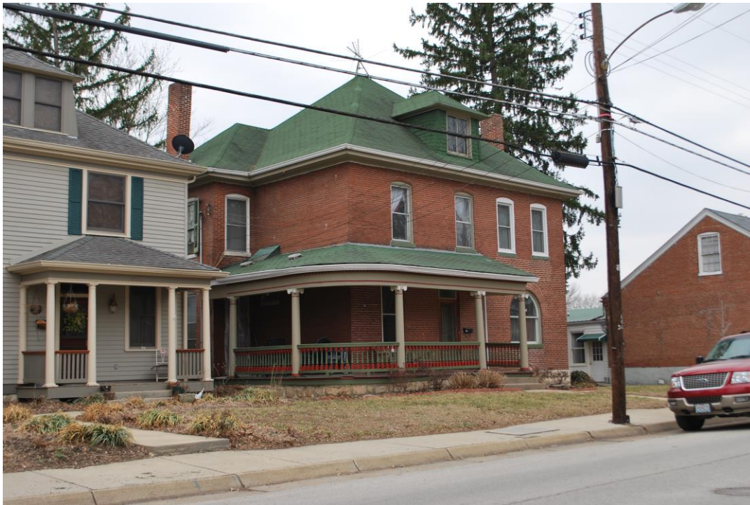
Figure 40. 502 (left) and 504 (right) W. Fifth Street contribute to the Stafford-Olive Historic District. View is southwest. Both dwellings were constructed c. 1910 and reflect the district's foursquare property type.
