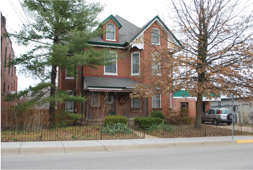
Figure 38. The dwelling at 311 W. Fifth Street is a contributing feature of the Tibbe Historic District. View is northeast.
