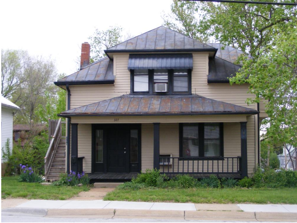
Figure 30. 327 E. Fifth Street, example of a frame hipped Bungalow, view is north.
