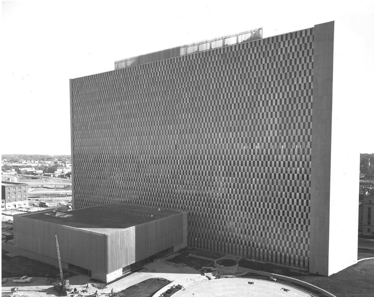
Figure 1. Federal Office Building construction photograph, September 1, 1965, view to the southeast showing the main entry on the west elevation and secondary entry on the north elevation of the low-rise block
