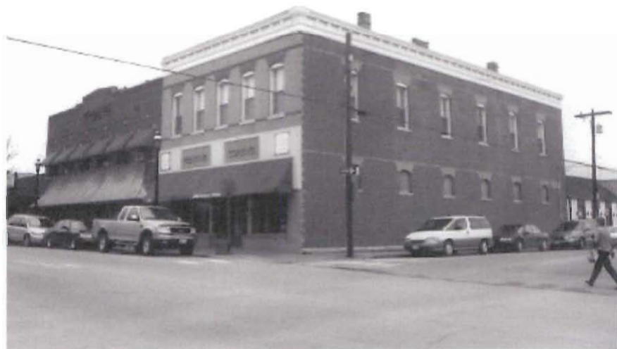
112 East Columbia, the Henry Meyer Building, ca. 1899.
