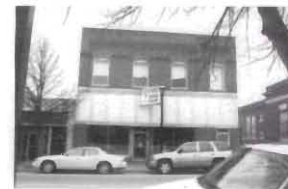
114 E. Columbia (Facade being restored.)
