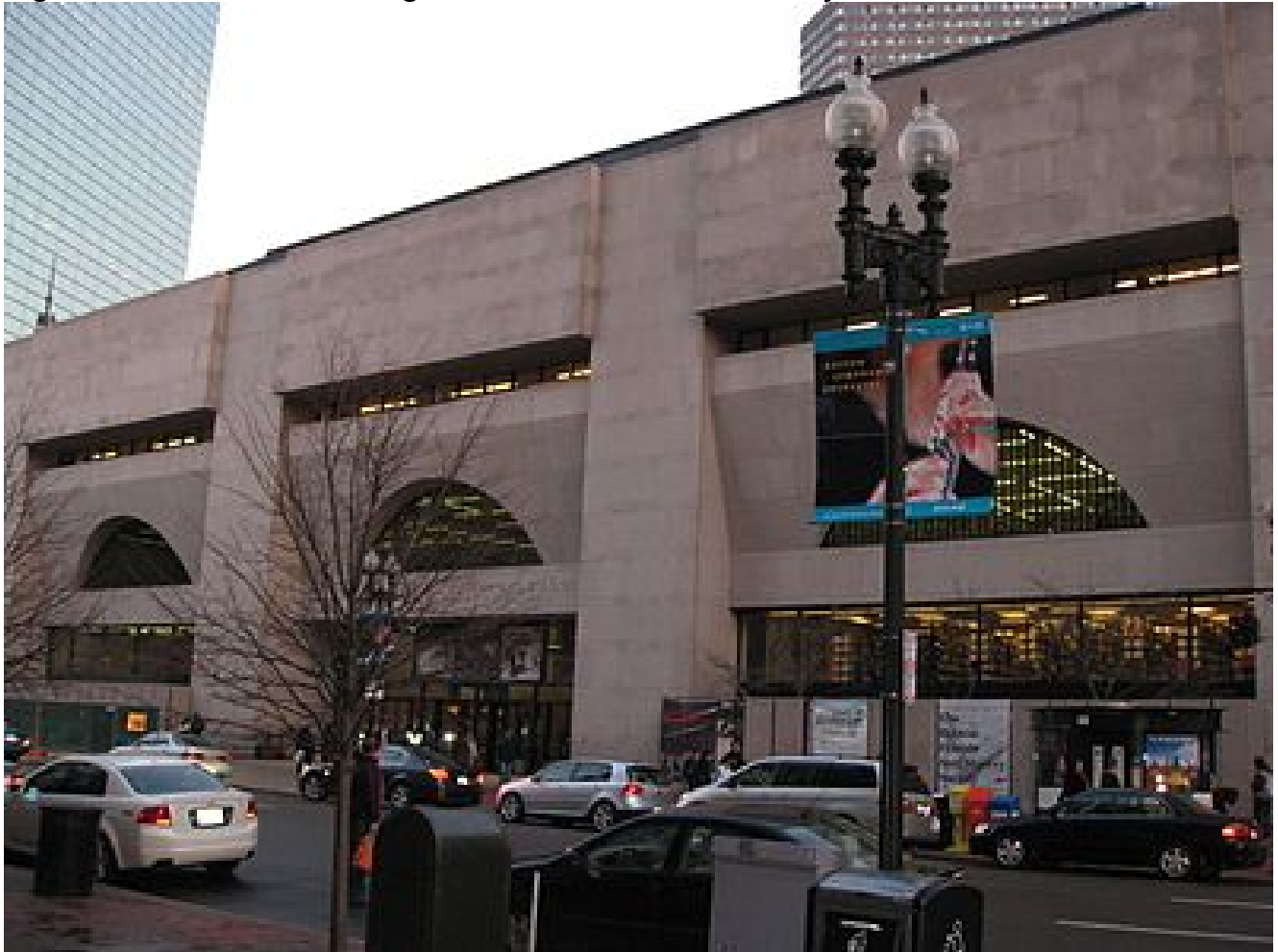
Figure 12: Johnson Building at the Boston Public Library 61
