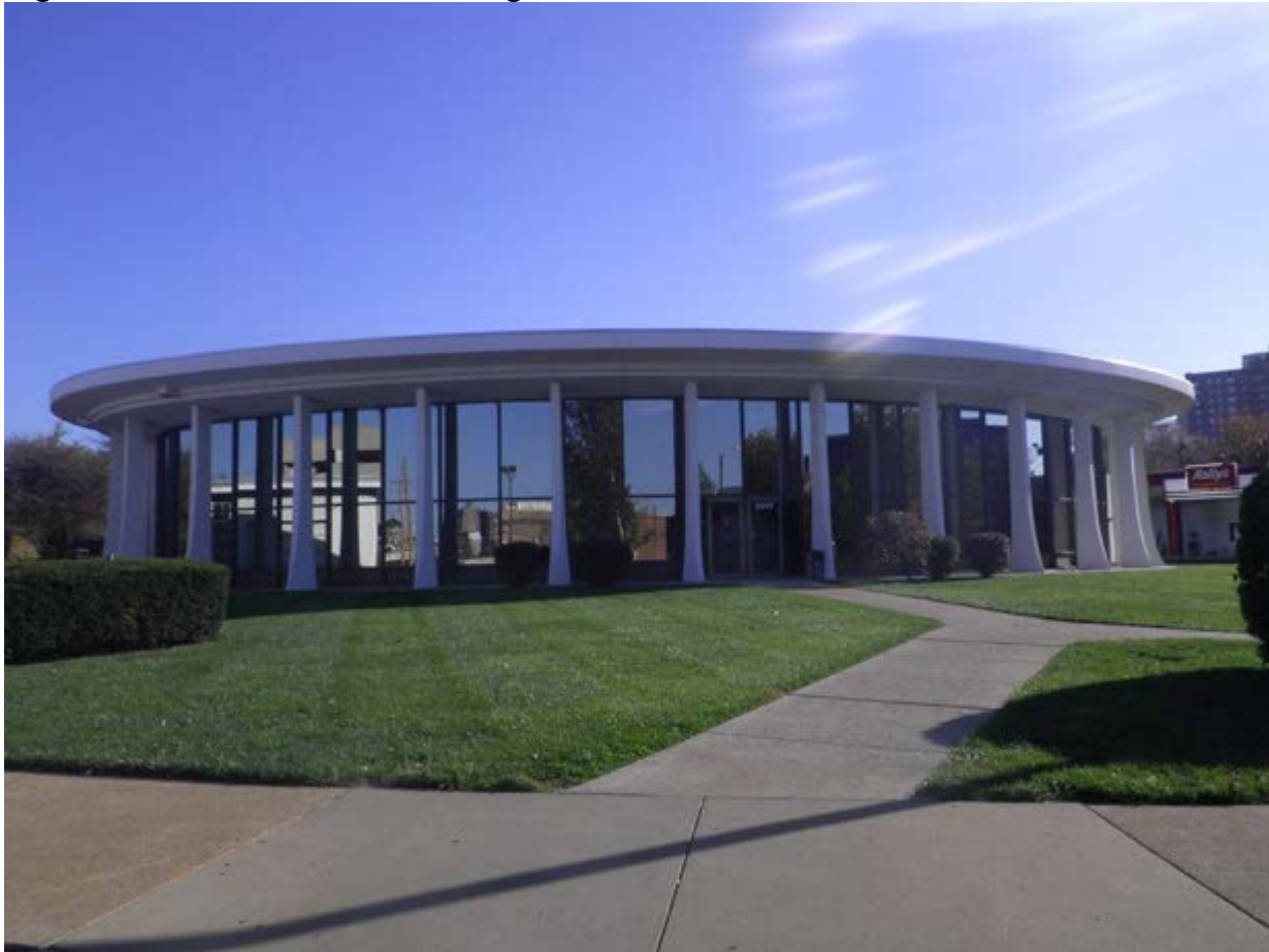
Figure 15: Photo of AAA Building 64
