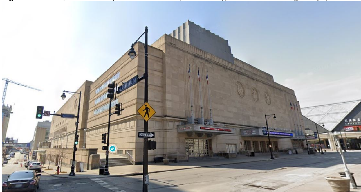
Figure 27. Municipal Auditorium, 301 W. 13 th Street, Kansas City, 2020. Source: Google Maps, 2019.
