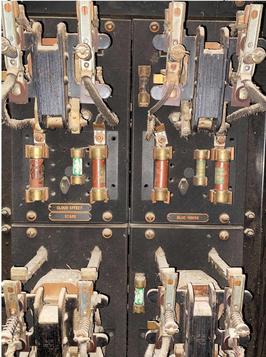
Figure 13. Detail of Cloud Effect control mechanism. Source: Rachel Consolloy, 2021.
