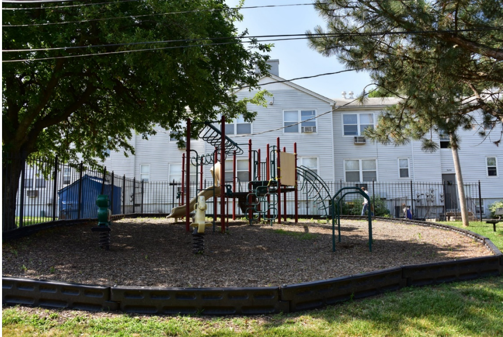
Figure 4. Playground and trash enclosure (typical). (Photographs by Brad Finch, f-Stop Photography, June 2021.)
