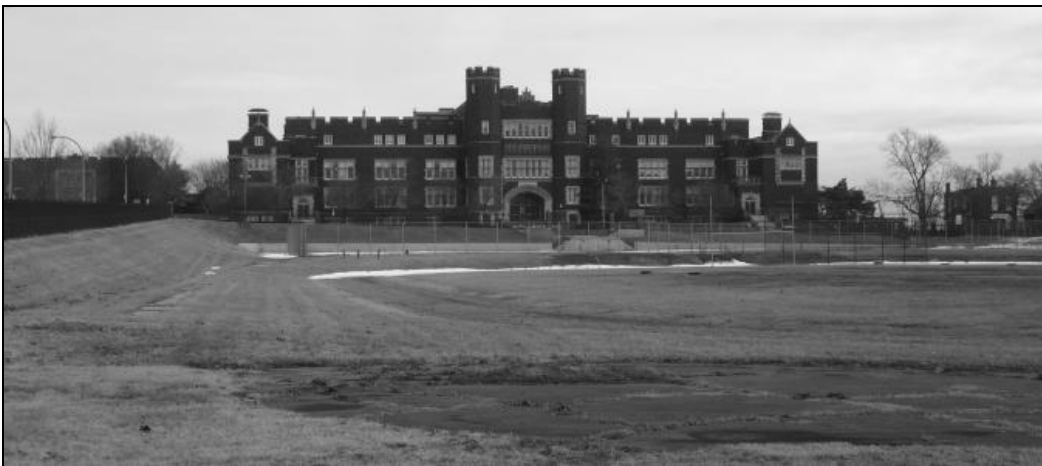
Grover Cleveland High School, 4352 Louisiana (tennis/track/football field, 4352 S. Grand)
