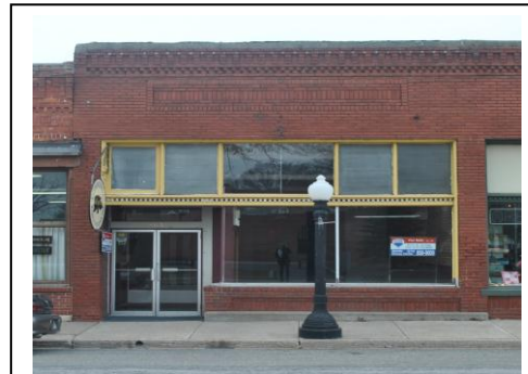
Figure 15. 103 E. Main Street – One Part Commercial Block
