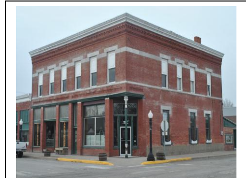
Figure 8. 104 S. Bridge Street – Financial Institution
