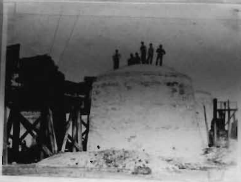
Wood being unloaded from the flat cars of the Sligo & Eastern Railroad, filling one of the huge kilns for the making of charcoal for the furnace.
