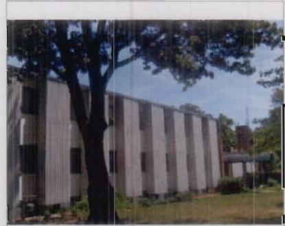
Front façade looking southeast from Forest
