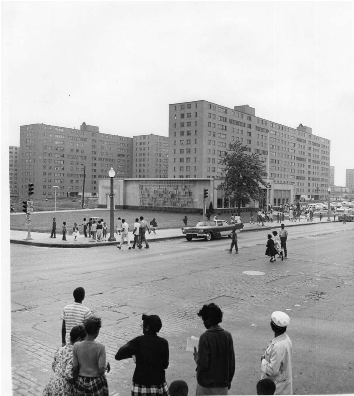
Figure 6. Crunden Library and Igoe Apartments, c. 1962. View is southeast. Photo courtesy of St. Louis Public Library, Archives (Central Branch).
