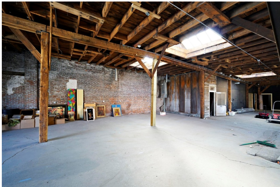
Figure 24: One-story wing, interior view facing east-southeast.
