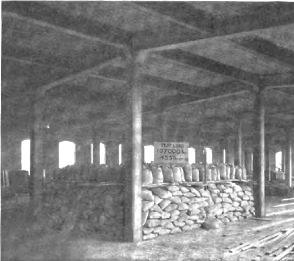
Floor Test. Showing Load of 107,000 Pounds. or 455 Pounds per Square Foot
