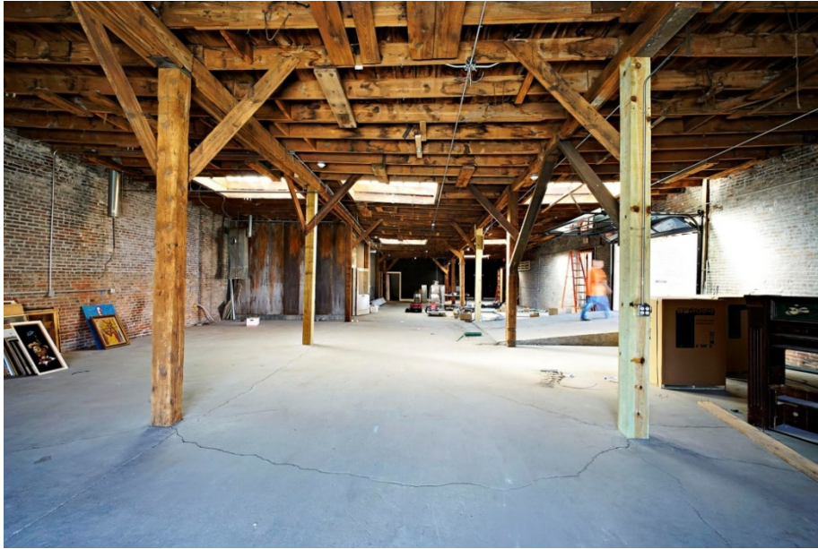
Figure 23: One-story wing, interior view facing south.
