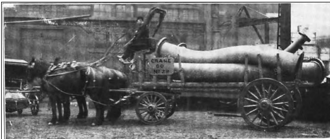
Crane Co. Wagon Loaded with Pipe Bends
