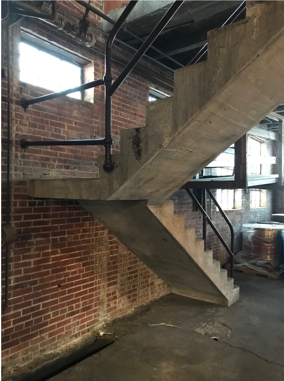
Figure 9: View of staircase landing. Source: Preservation Research Office photograph, 2018.
