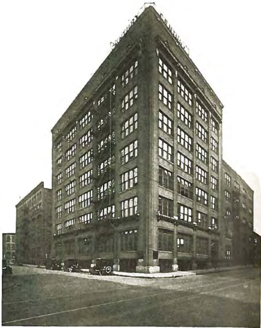
Main plant of the Century Electric Company, the largest manufacturer of single phase motors in St. Louis.
