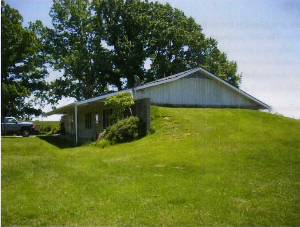
Structure 80a (House), view E
