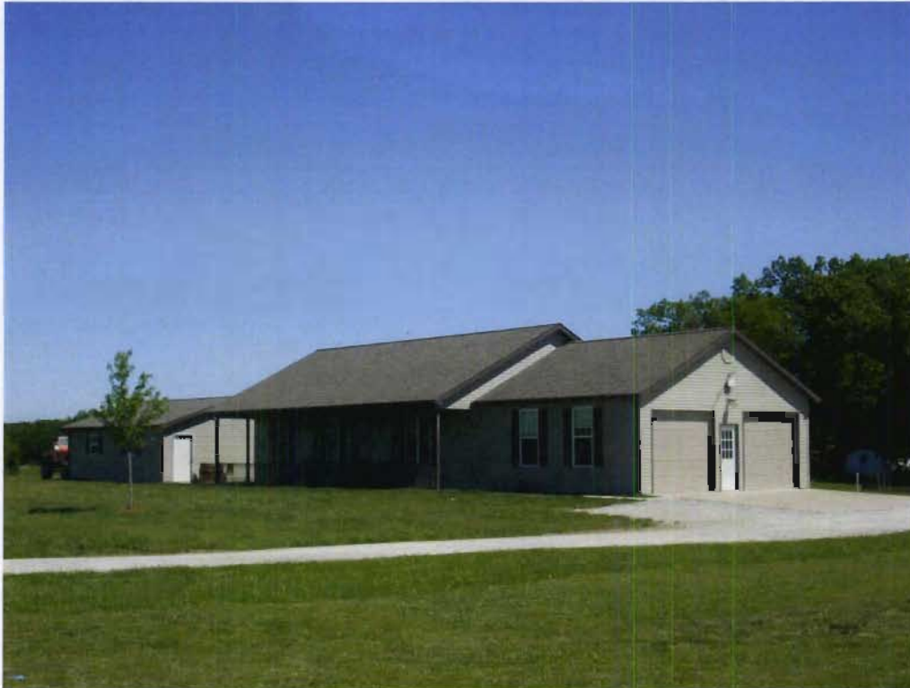
Structures 95e (Detached shed/workshop), 95c (House), and 95d (Small shed behind house), pictured from left to right, view SW
