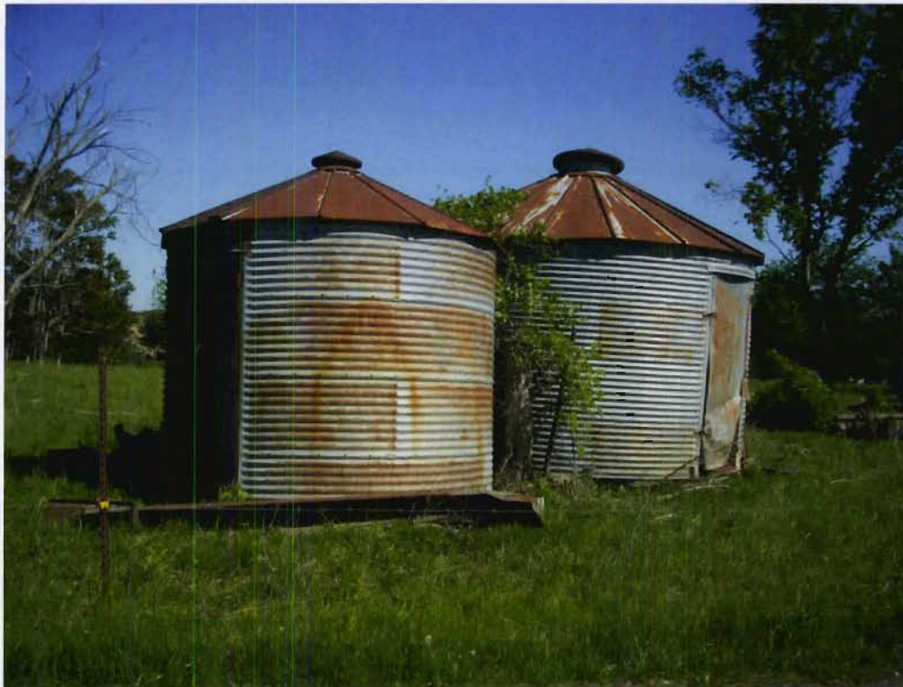
Structure 75h (Pair of small silos), view E
