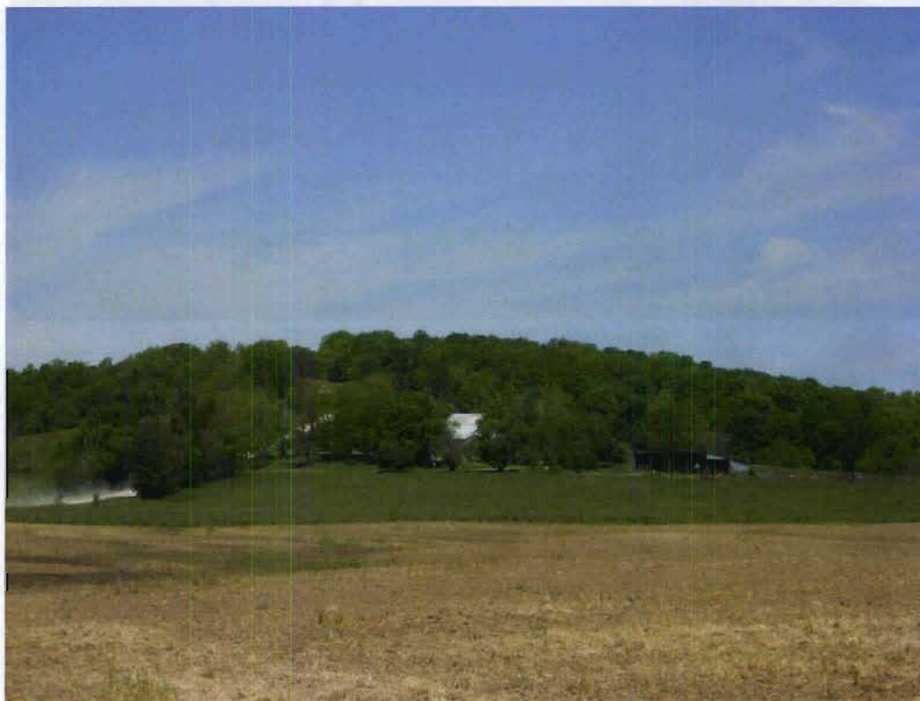
Property 124/128, view N, visible structures are top of Structure 128c (Barn), pictured center, and Structure 128b (Pole barn), pictured right
