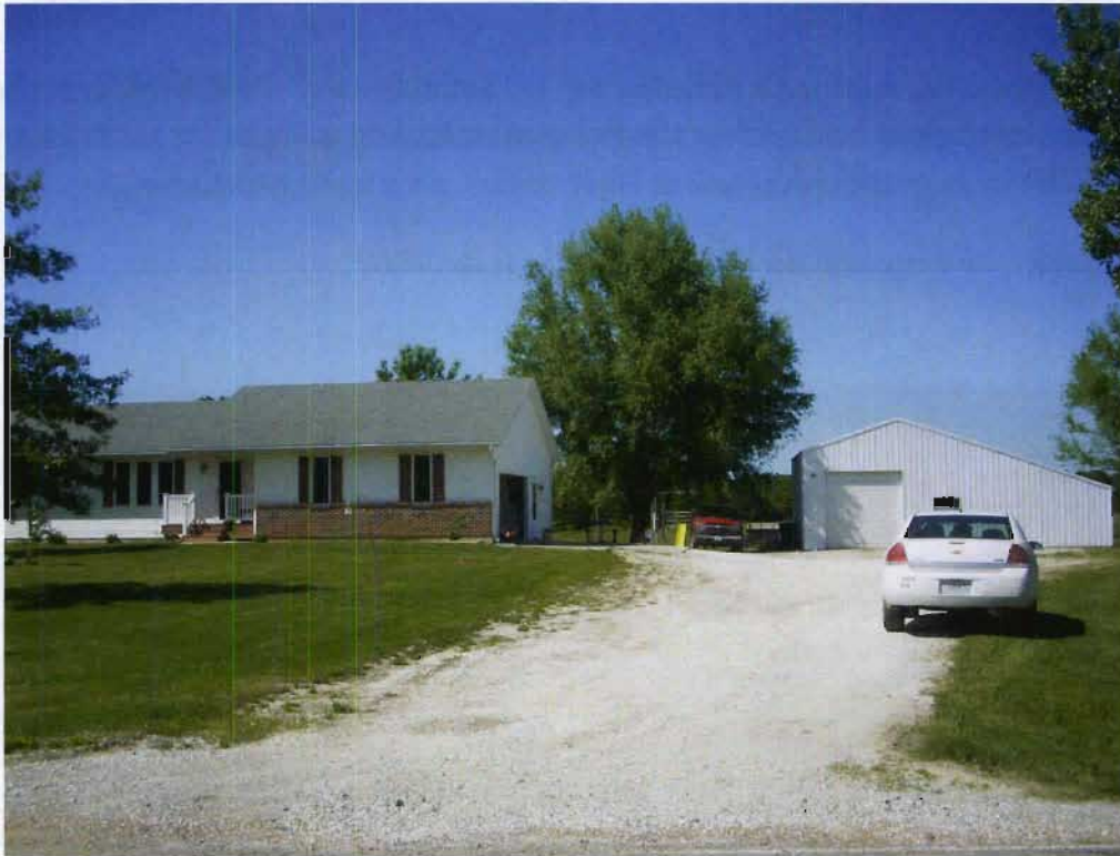
Structures 98b (House) and 98c (Barn/shed), pictured from left to right, view NNW
