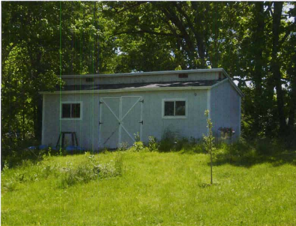
Structure 33b (Small shed), view SE
