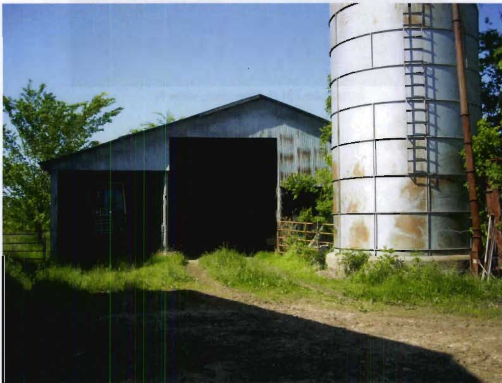
Structure 75e (Equipment barn), view N
