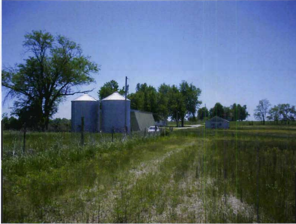
Structure 40d (Silo pair behind metal shed), view SSE
