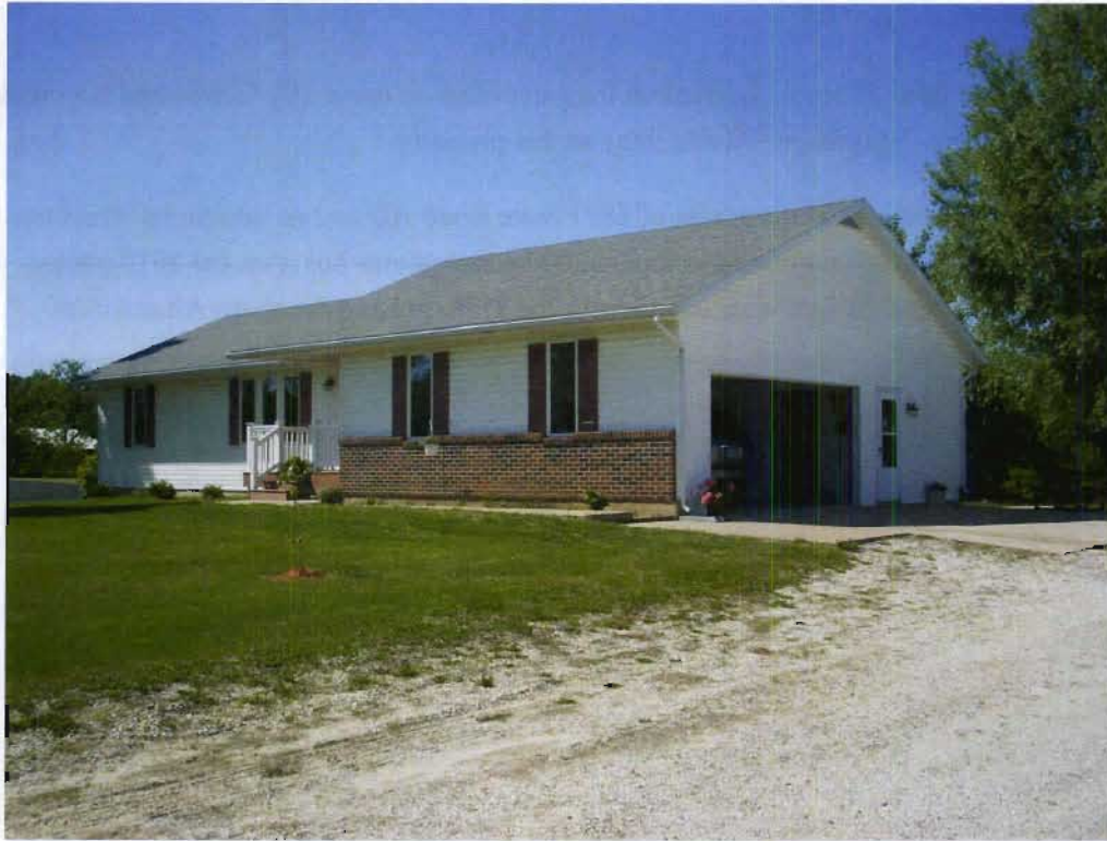
Structure 98b (House), view NNW
