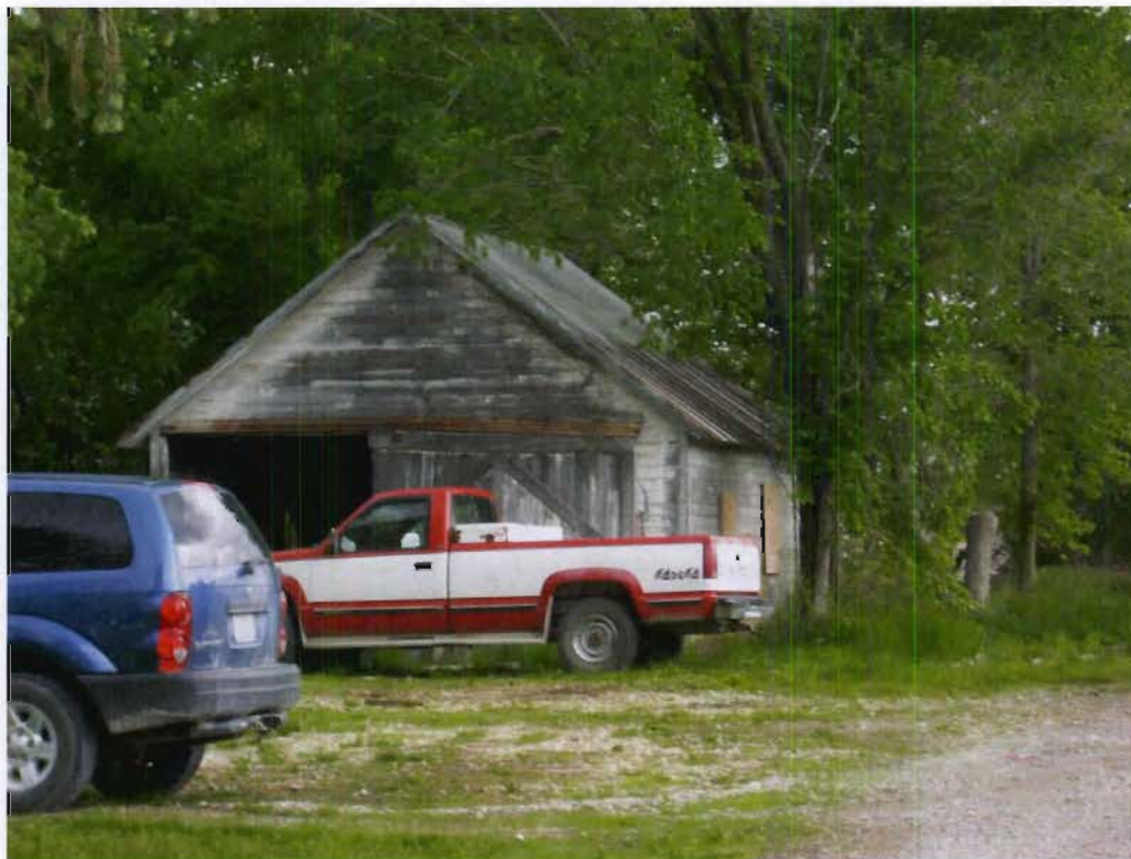
Structure 17c (Outbuilding), view SW
