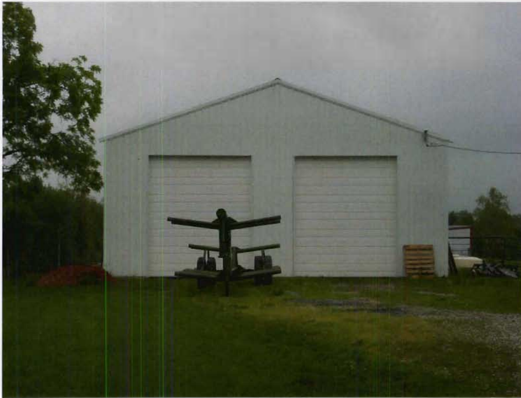
Structure 19b (Outbuilding), view N
