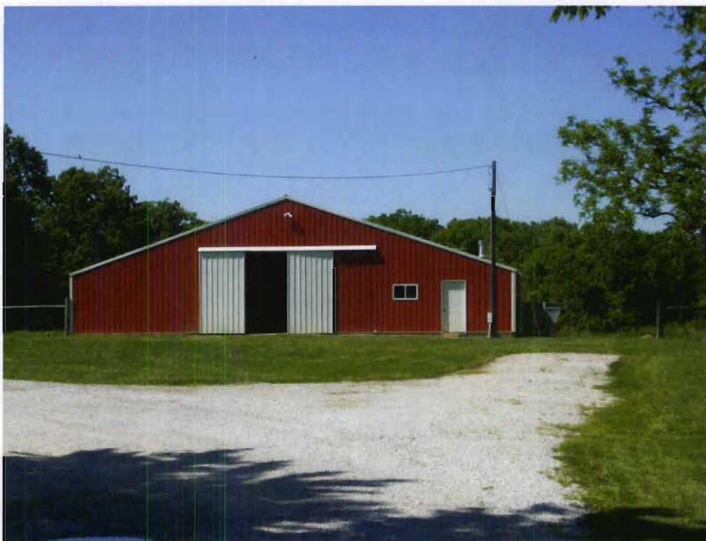
Structure 97c (Barn), view N
