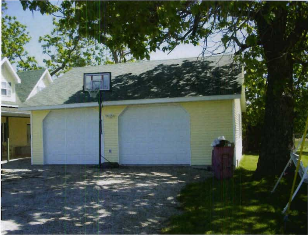
Structure 91b (Garage), view SE
