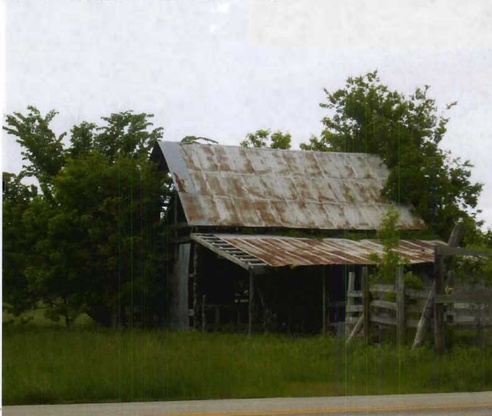
Structure 142a (Barn), view NNE
