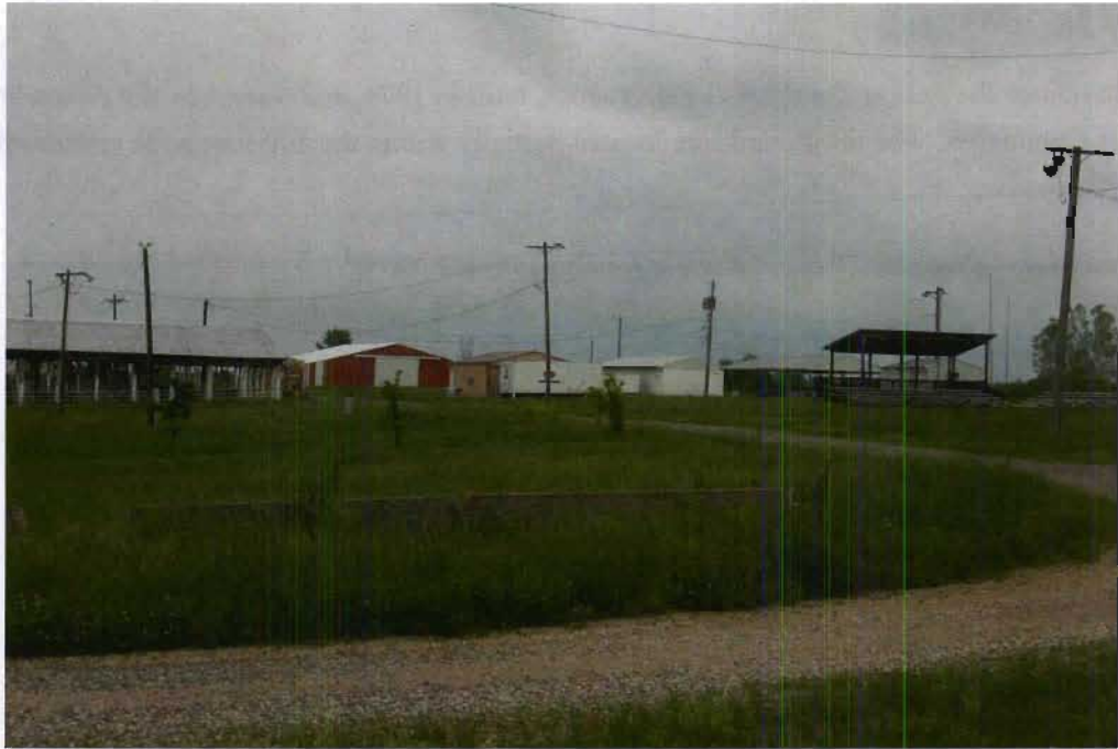
Structures on the 4-H Fairgrounds, view NNW
