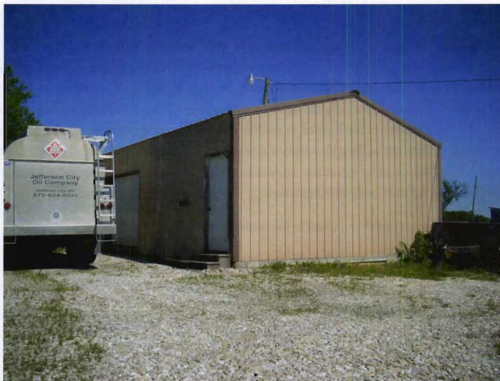
Structure 68b (Modern metal shed), view SE
