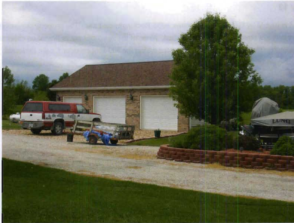
Structure 13b (Garage), view NNW
