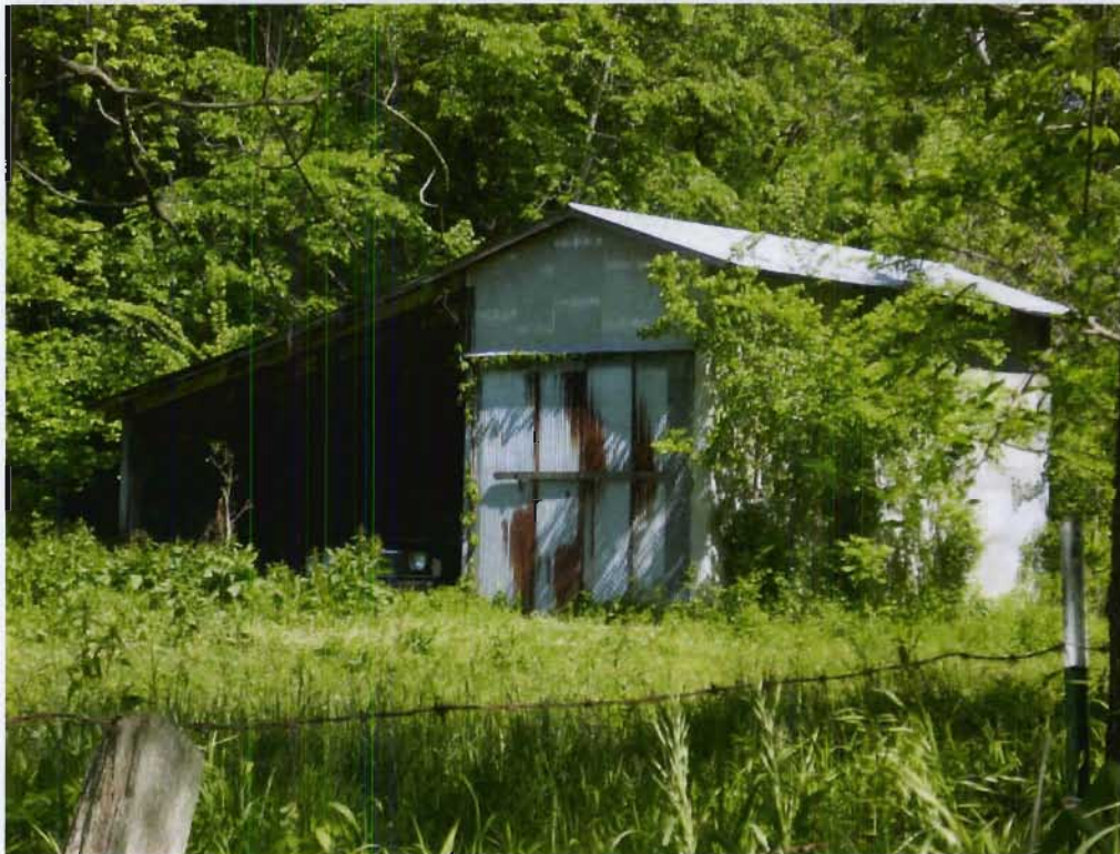
Structure 60a (Metal Shed/Barn), view NW
