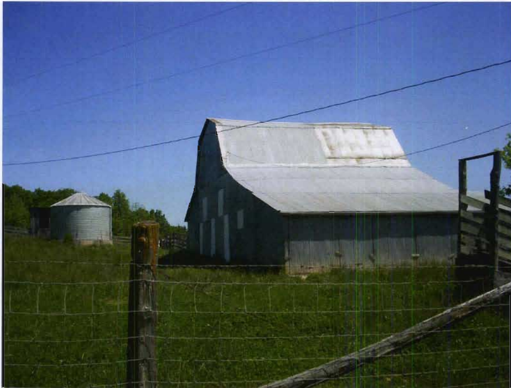
Structures 128e (Shed), 128d (Silo), and 128c (Barn), pictured from left to right, view NE
