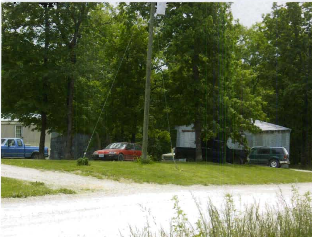
Structures 165c and 165d (Metal sheds), view SW
