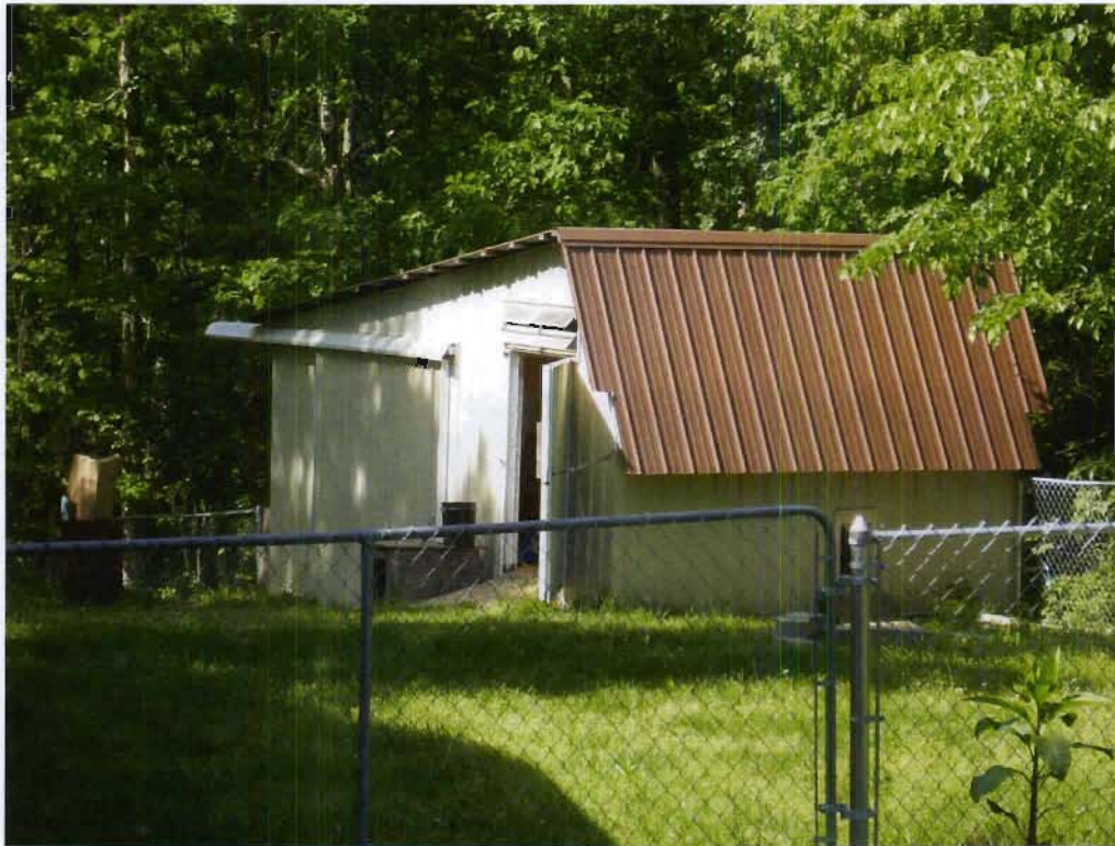
Structure 107b (Shed), view SW
