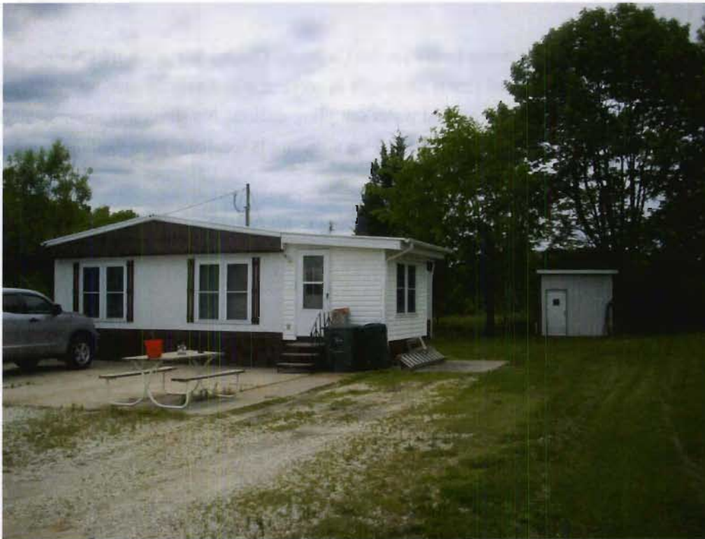
Structures 154a (House) and 154d (Shed #2), view W
