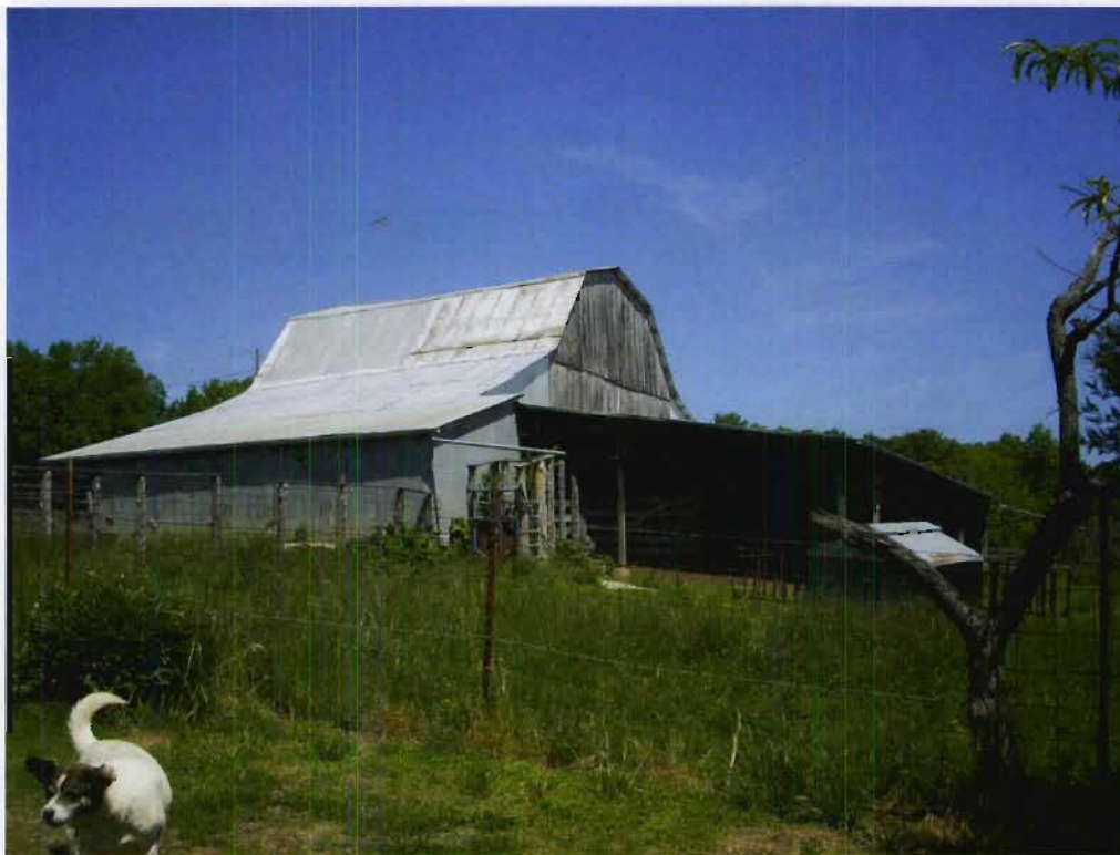
Structure 128c (Barn), view NW
