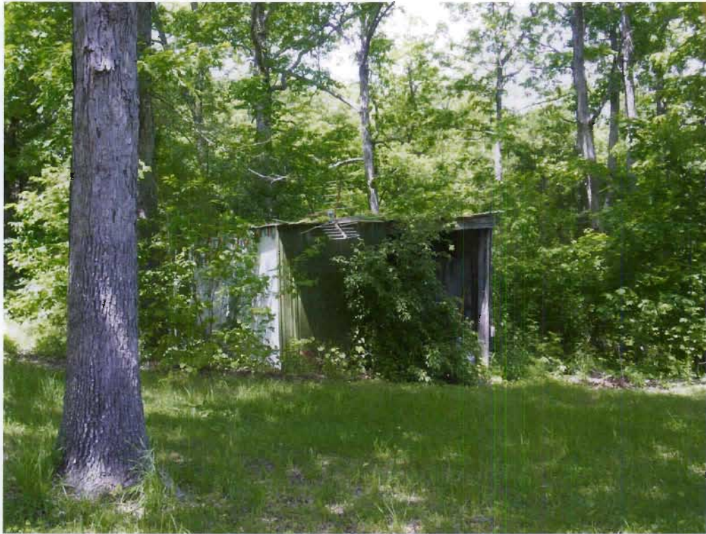
Structure 170b (Shed), view N
