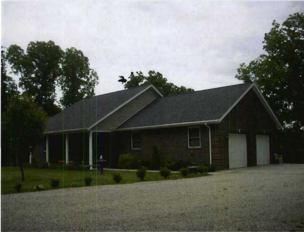
Structure 139a (House), view E
