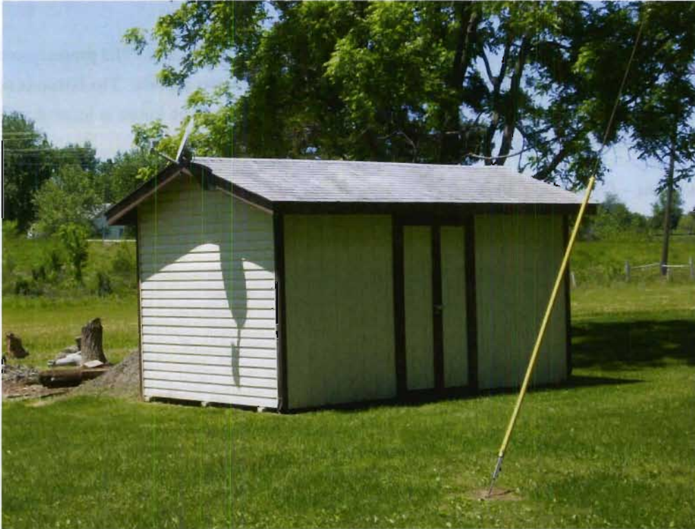
Structure 55b (Shed), view SW
