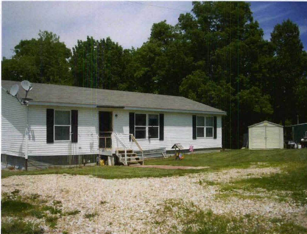
Structures 173a (House), 173b and 173c (Small sheds), view NNW
