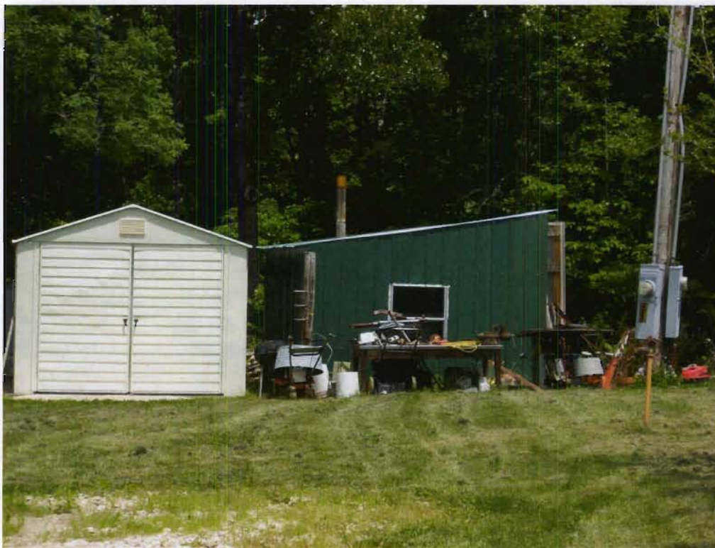
Structures 173b and 173c (Small sheds), view N
