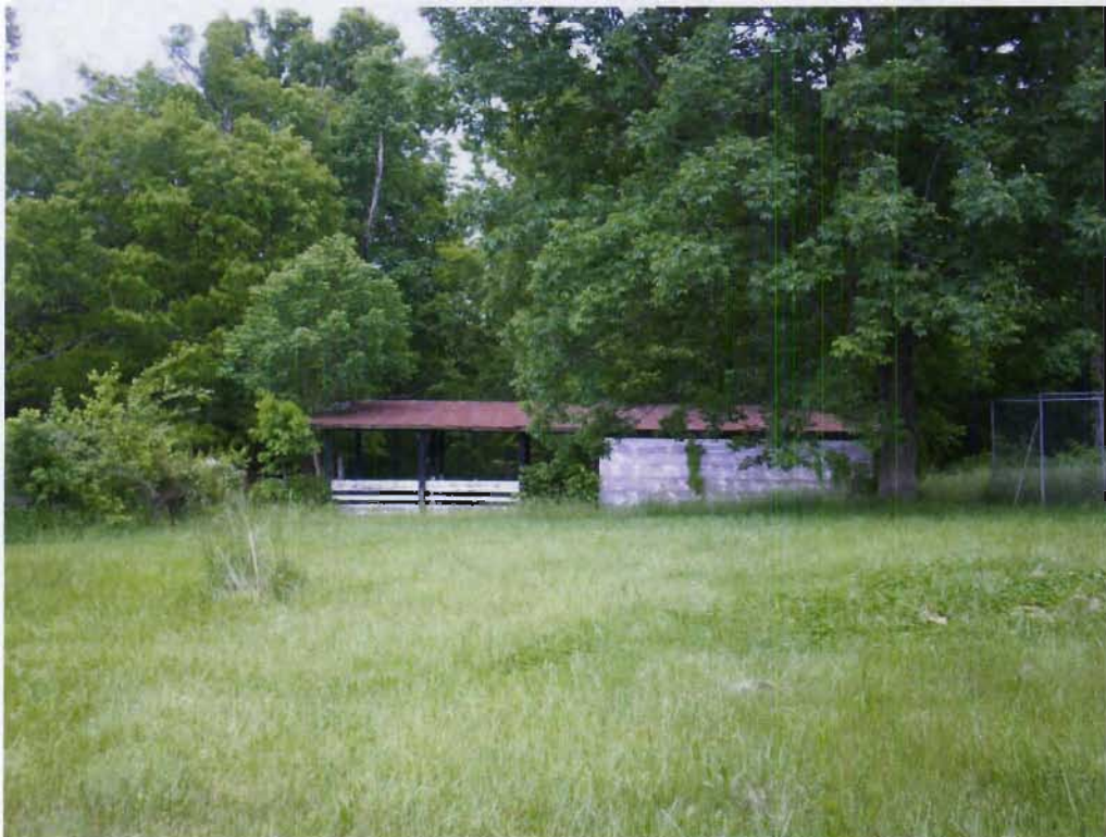
Structure 138b (Shed), view S
