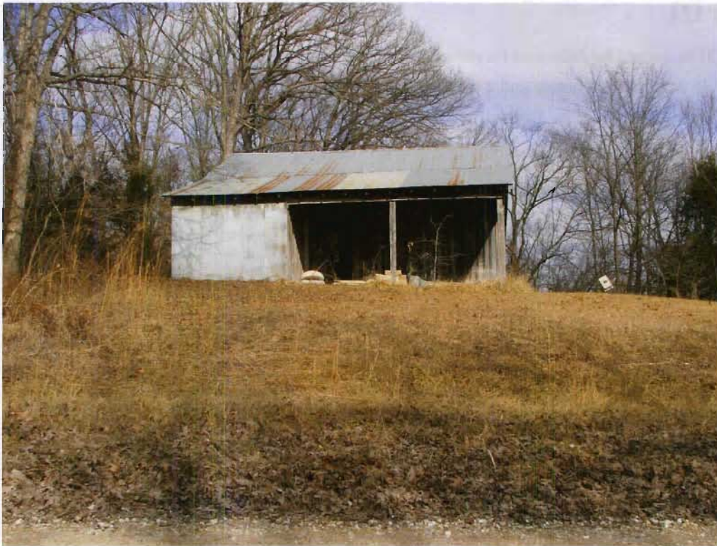
Structure 170c (Barn), view N (2010)
