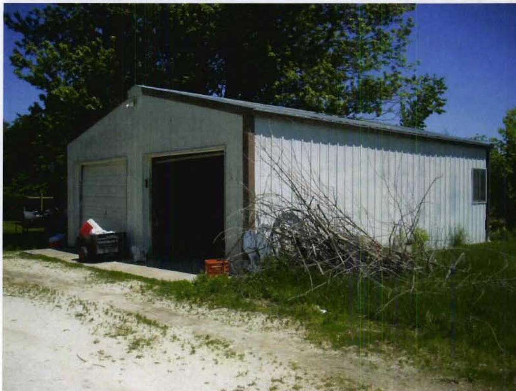
Structure 85b (Garage), view NE
