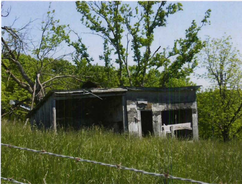
Structure 128h (Outbuilding), view N
