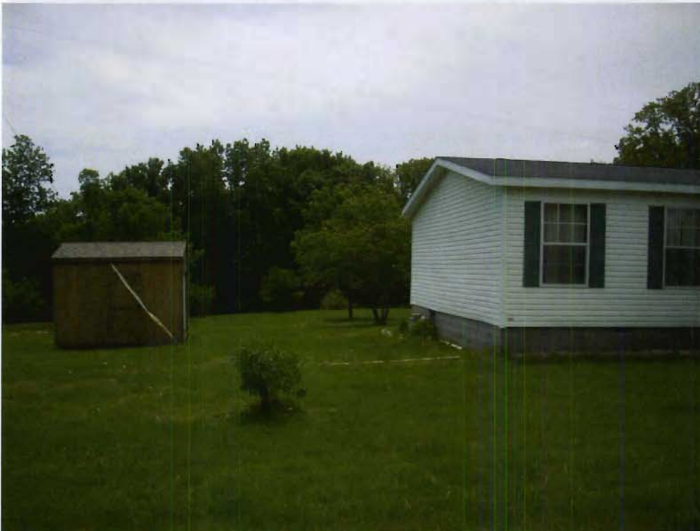
Structures 174a (House) and 174c (Shed #2), view S
