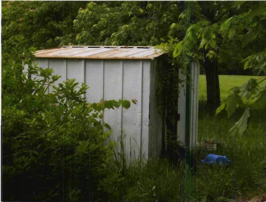
Structure 178f (Small metal shed), view SW
