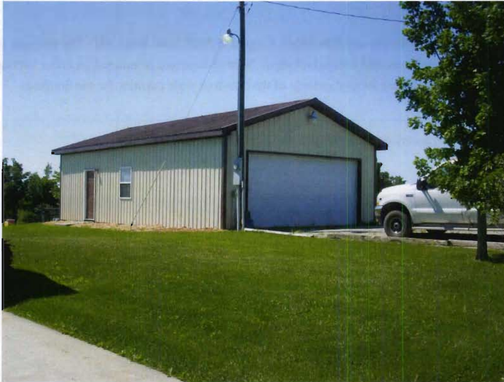
Structure 66b (Shed), view N
