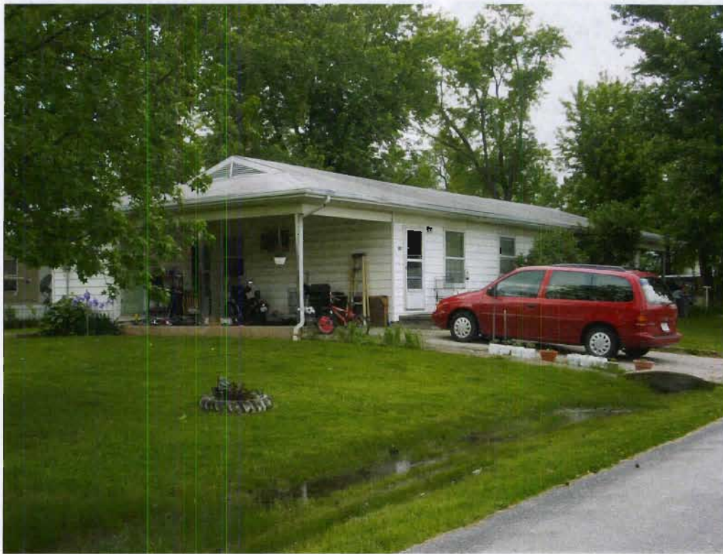
Structure 9e (Duplex), view W
