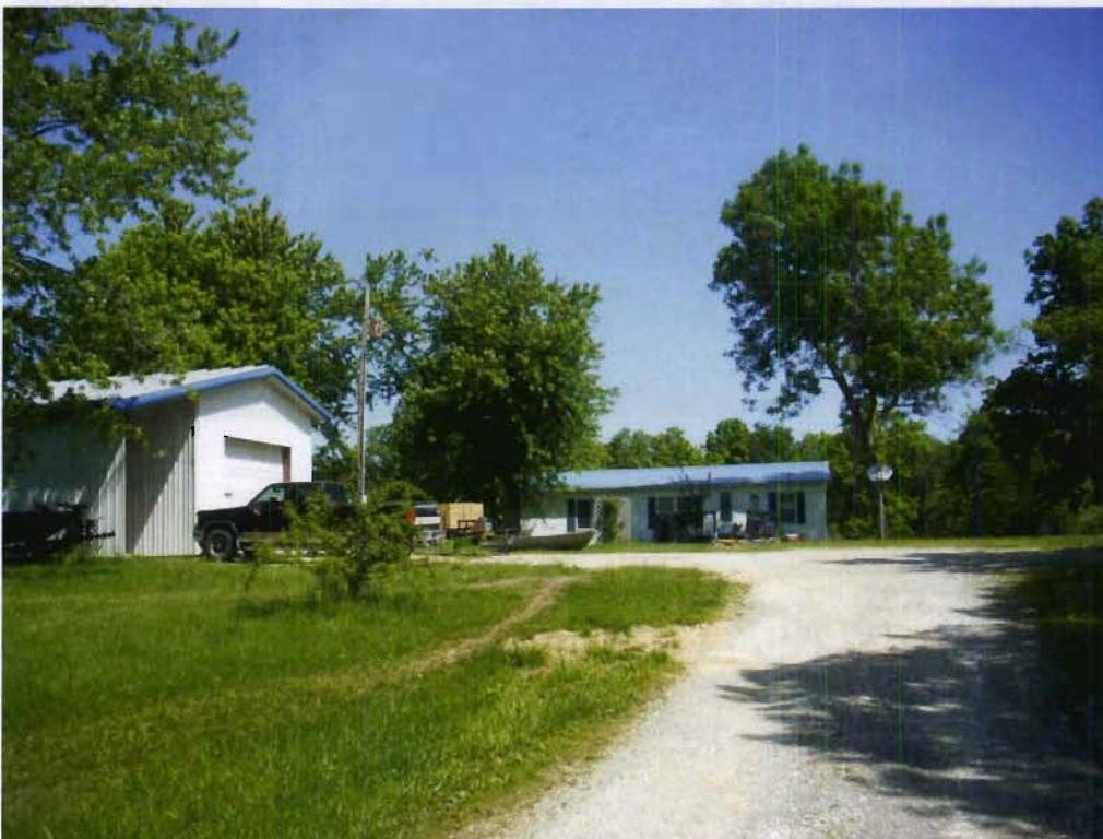
Structures 112b (Garage) and 112a (House), pictured from left to right, view N
