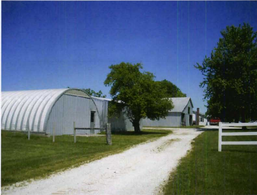
Structure 43e (Metal shed and Quonset building), with 43d (Large metal barn) pictured in center and 43a (House) pictured right of center, view NE
