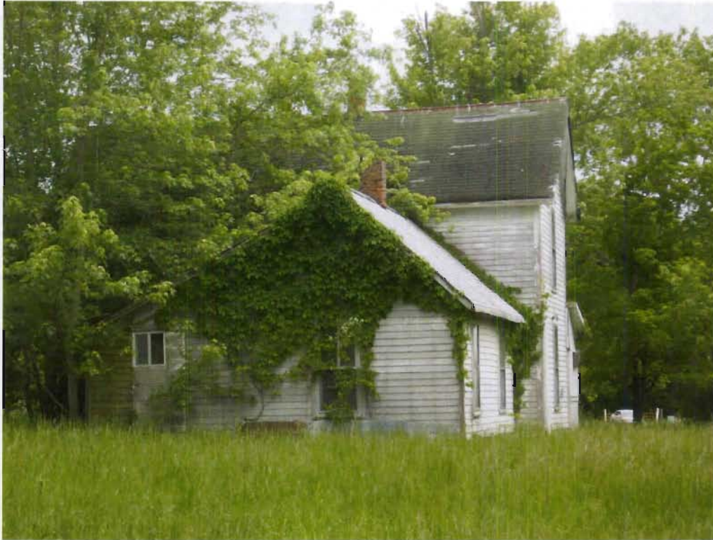
Structure 152a (House), view S
