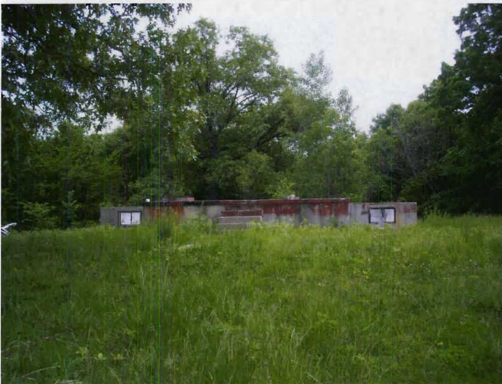
Structure 182c (Foundation), view S
