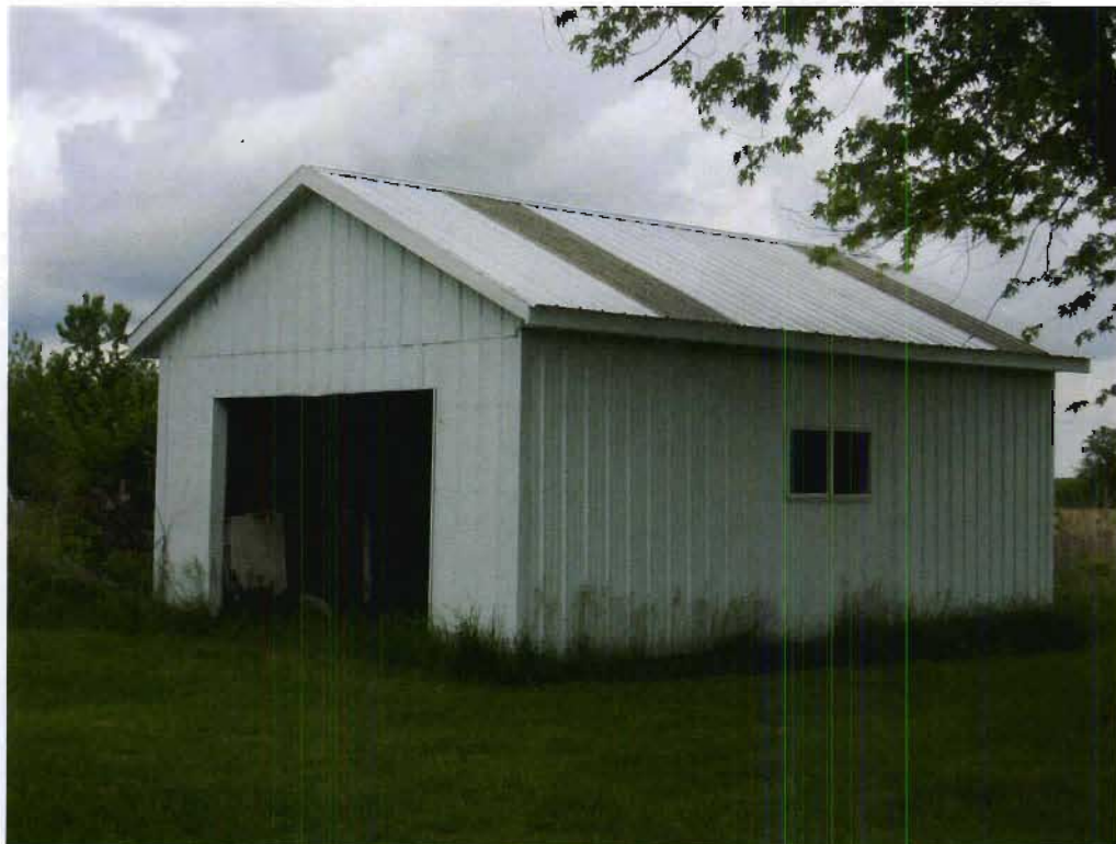
Structure 9h (Garage), view NE
