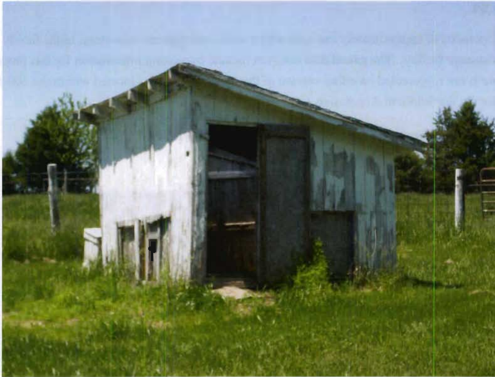
Structure 48f (Shed), view NW
