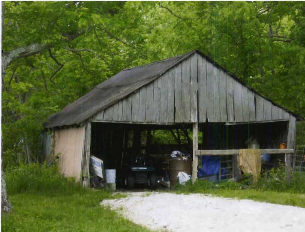
Structure 136b (Shed), view S
