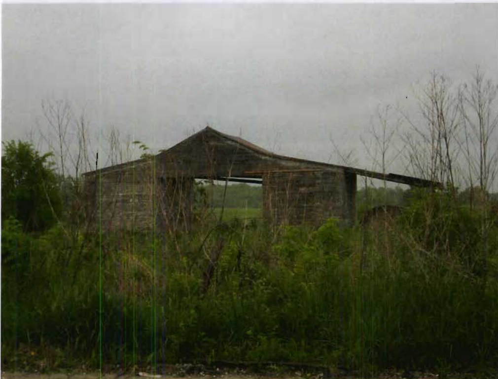
Structure 18b (Outbuilding), view NE
