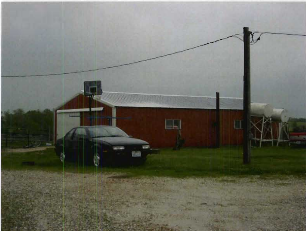
Structure 19c (Outbuilding), view NW
