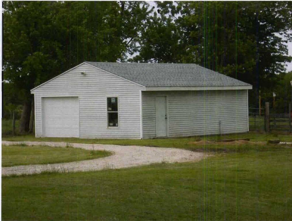
Structure 151b (Garage), view NW
