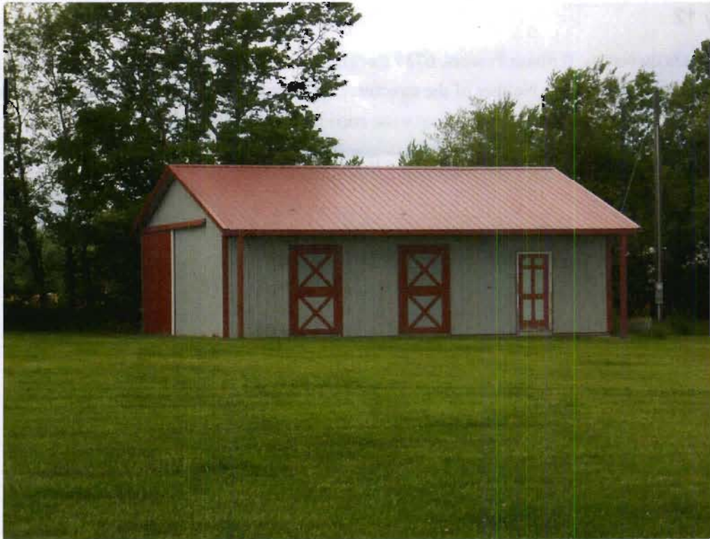
Structure 12b (Shed), view W
