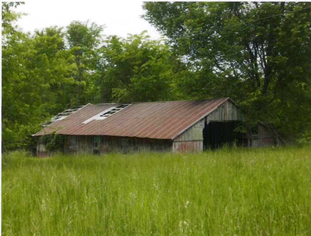
Structure 152c (Barn #2), view NW
