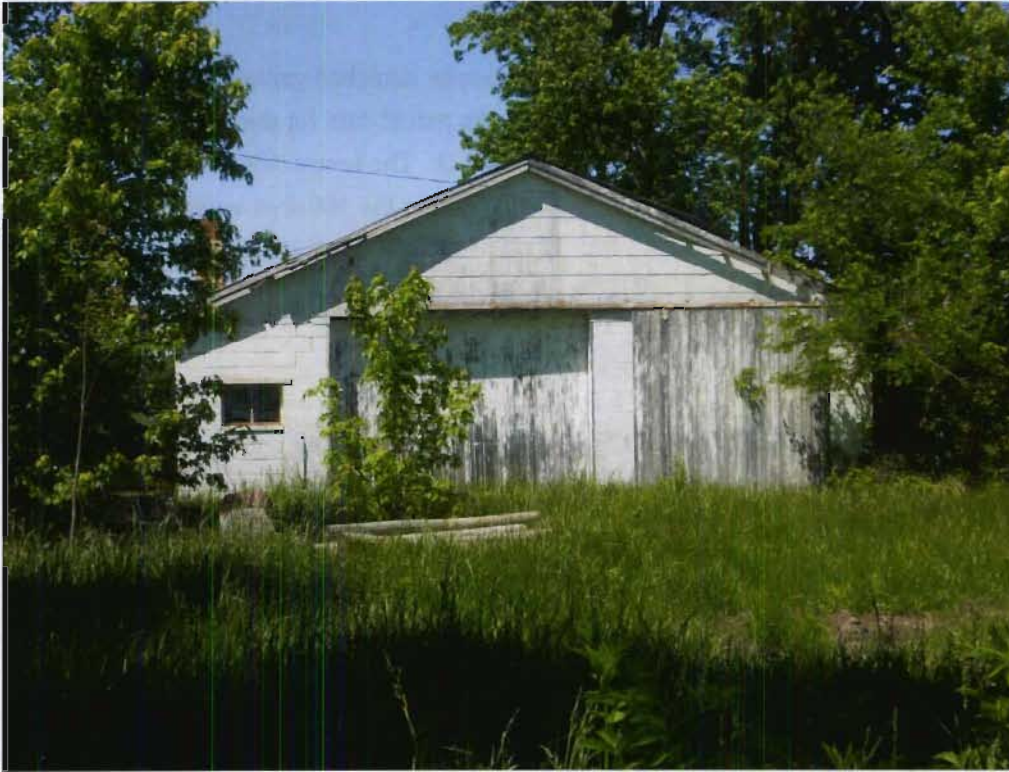
Structure 88c (Smaller structure), view N
