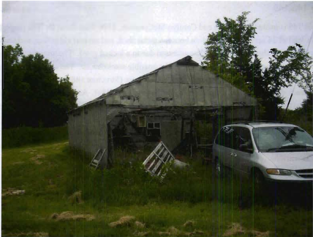
Structure 149a (Metal shed), view NE
