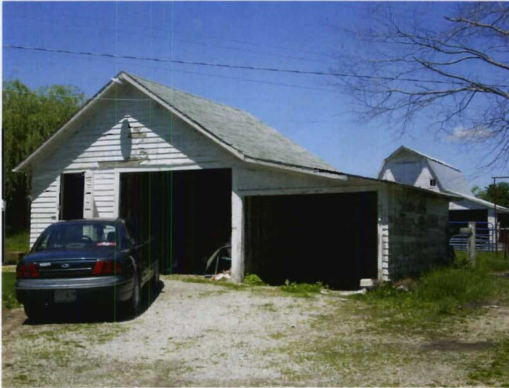
Structure 48b (Garage), view NW
