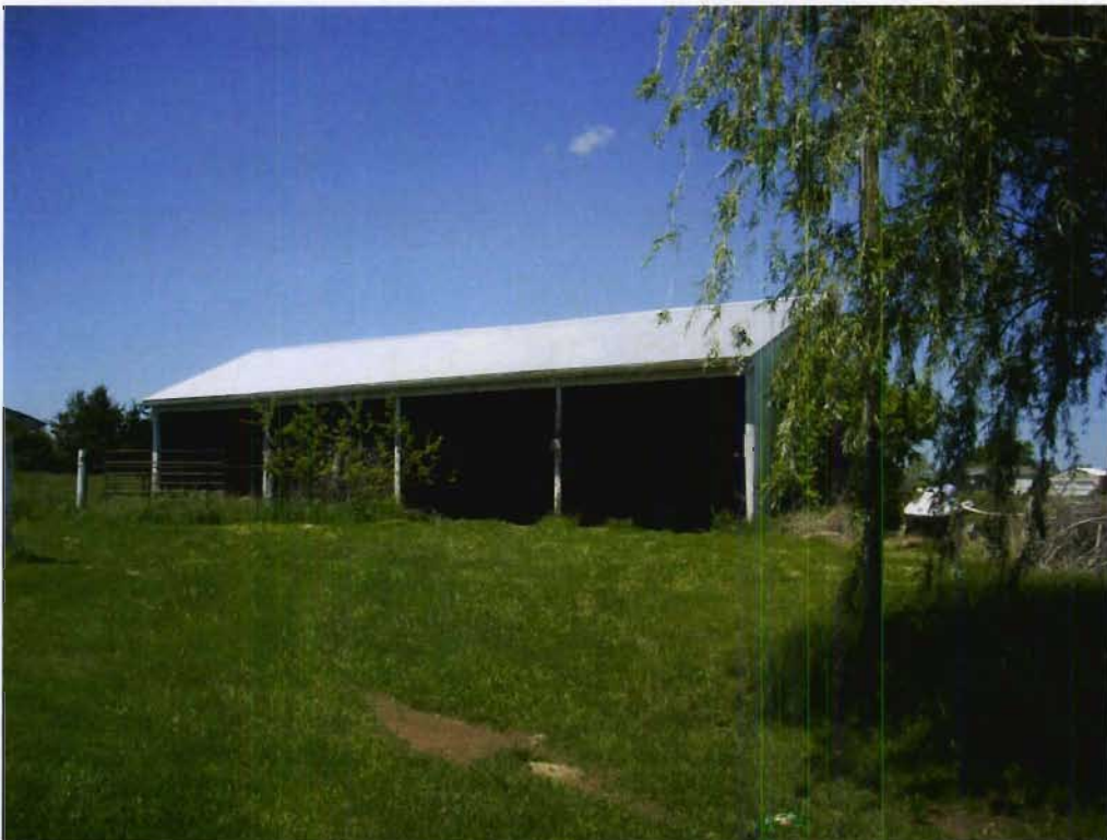
Structure 48e (Pole Barn), view NW
