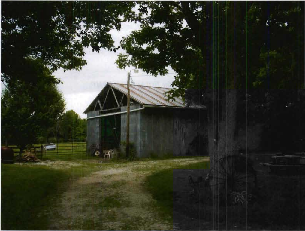
Structure 143b (Barn), view SW
