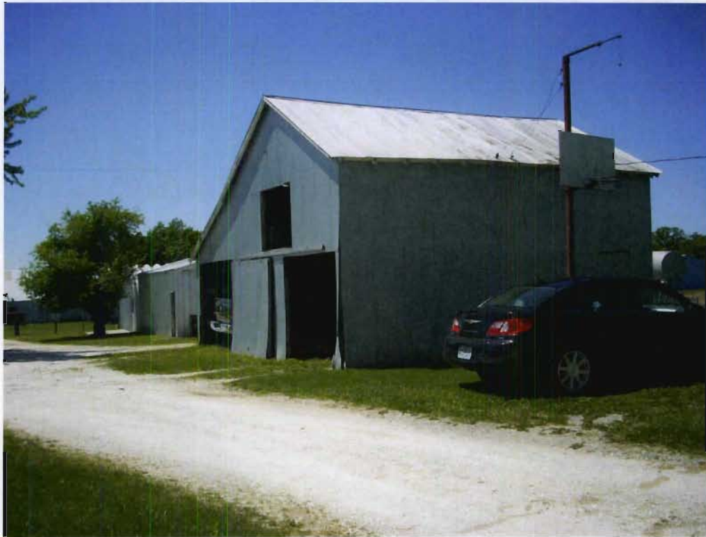
Structure 43d (Large metal barn), view NW
