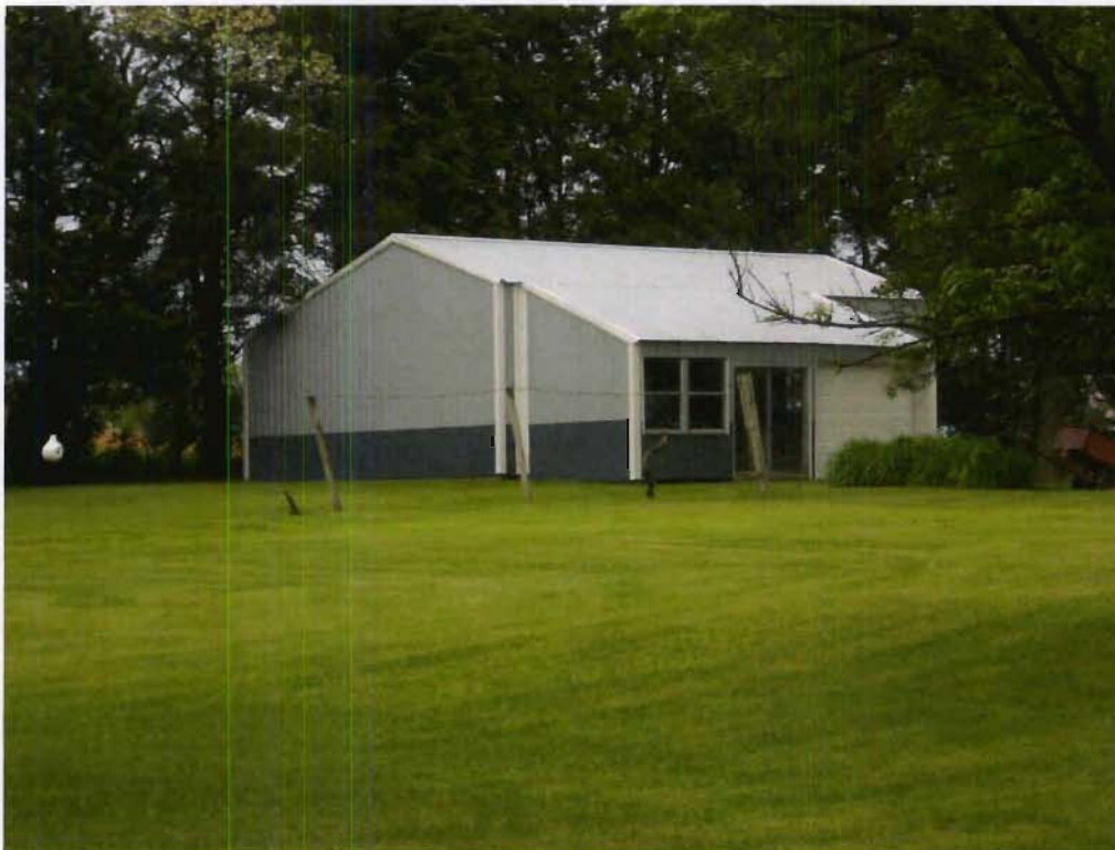
Structure 24c (Metal building), view NE
