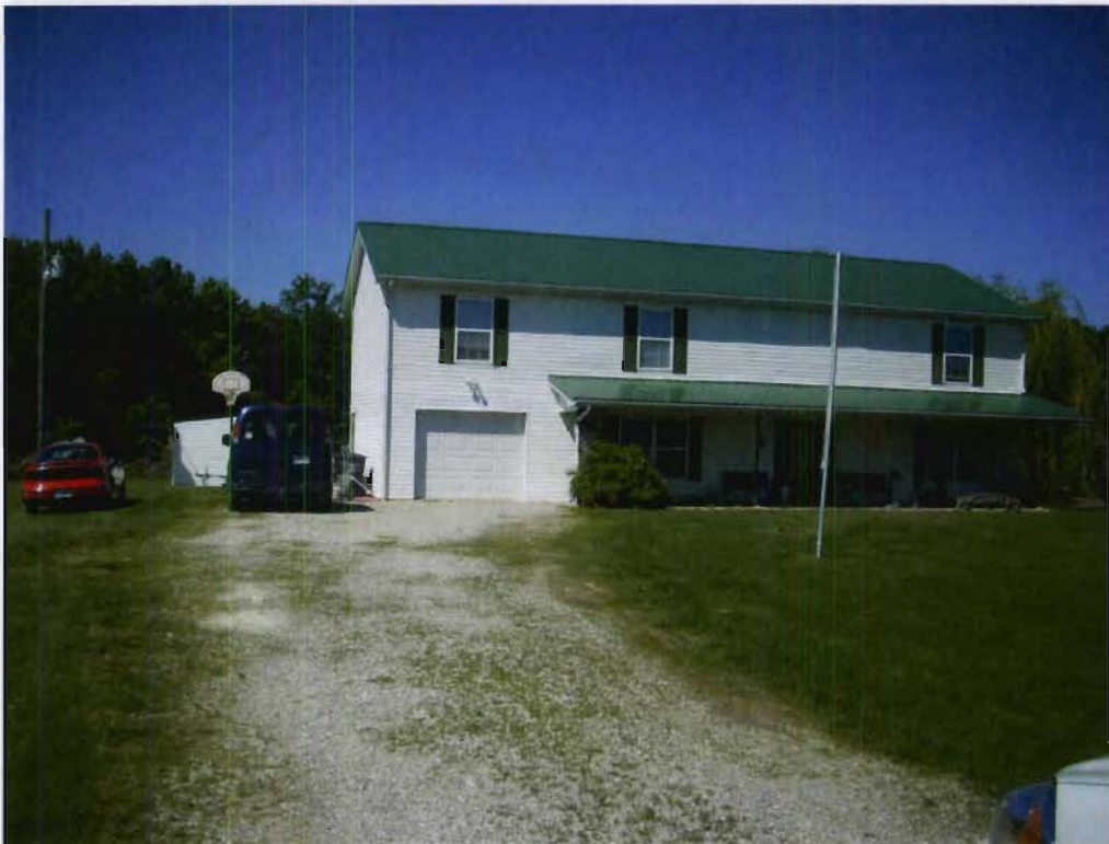
Structures 96b (Shed) and 96a (House), pictured from left to right, view N
