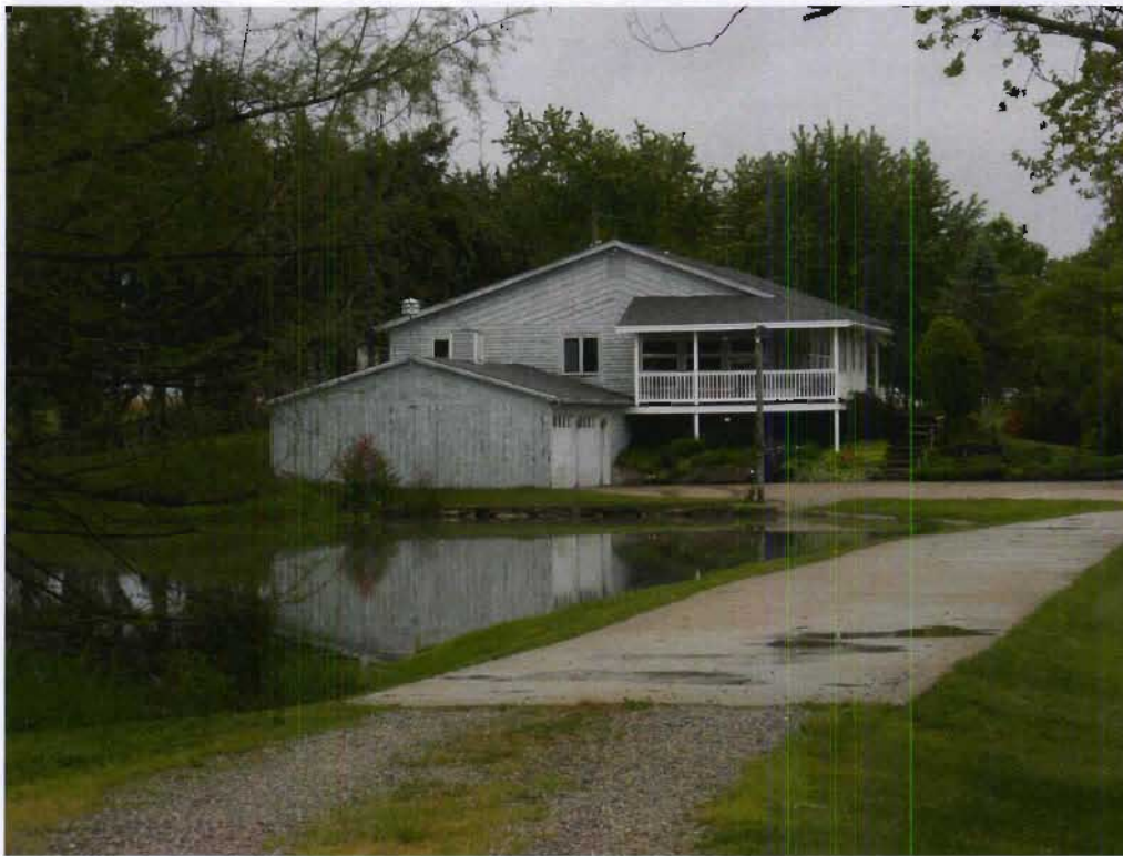
Structure 24a (House), view E
