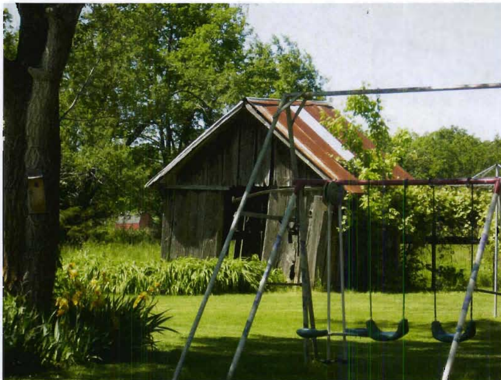
Structure 94i (Smokehouse), view NW
