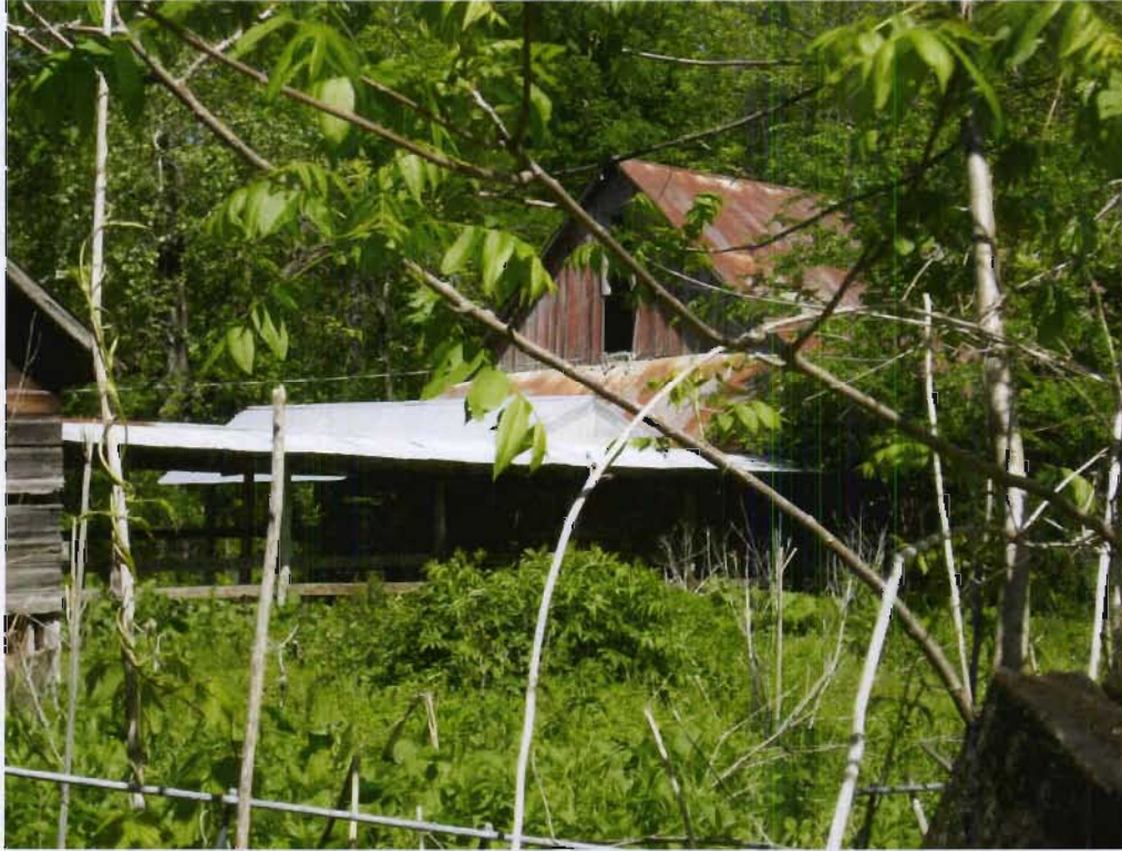
Structure 60b (Red wooden barn), front view, view NW
