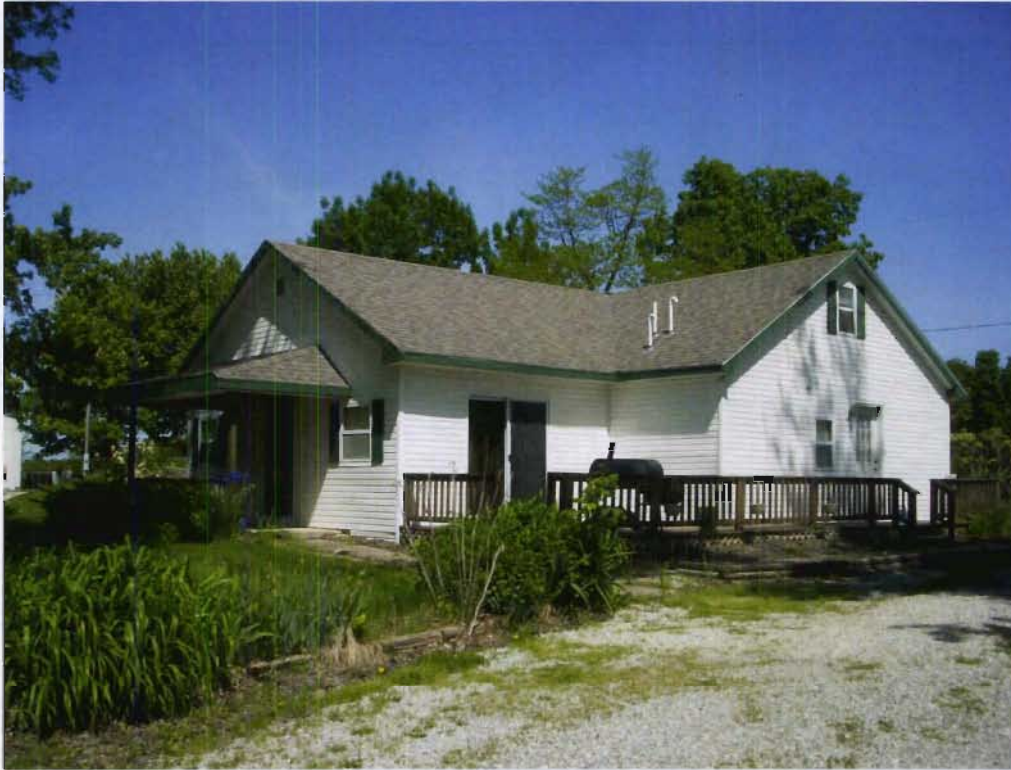
Structure 112c (House), view NW
