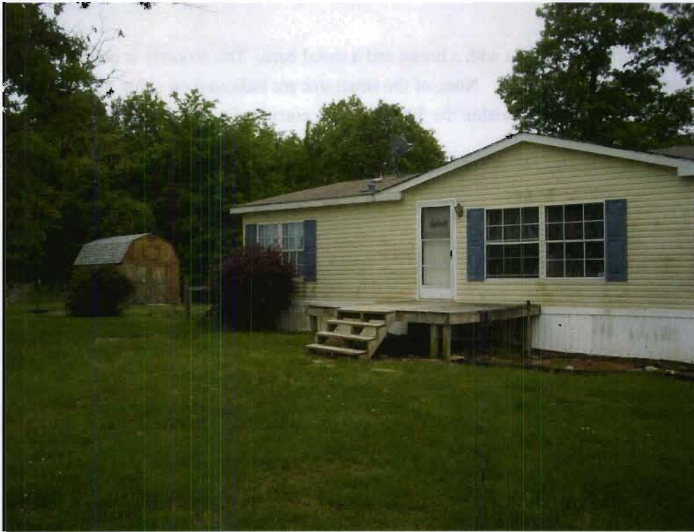
Structure 182b (Shed), view ESE
