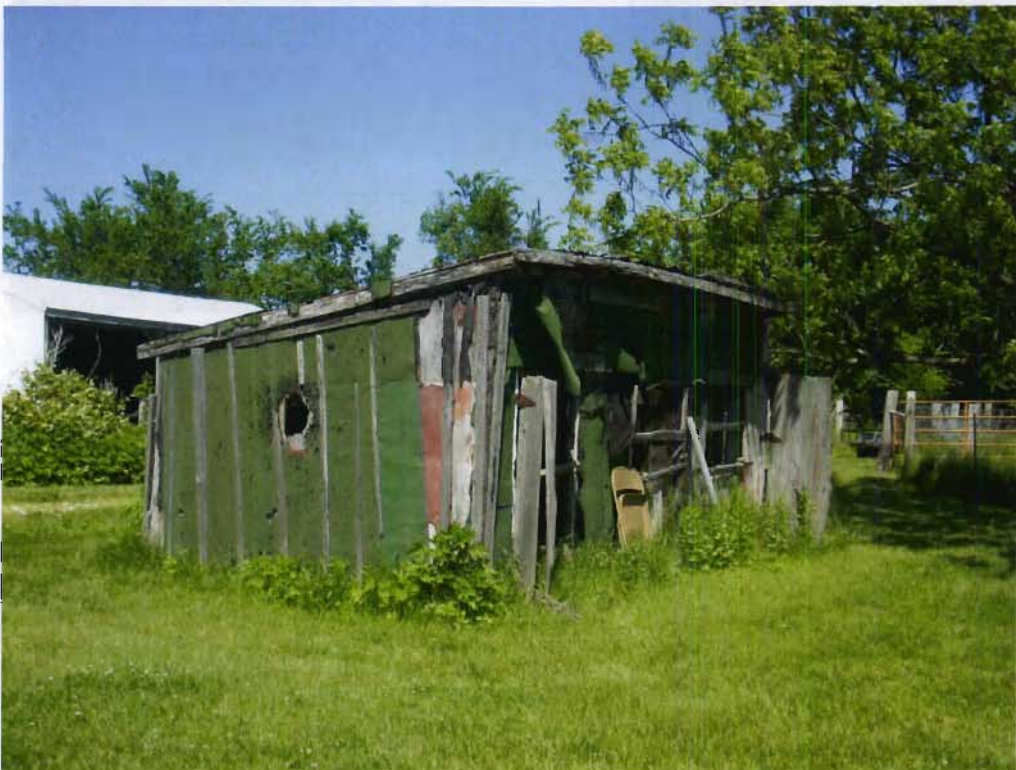
Structure 64c (Shed), view NE
