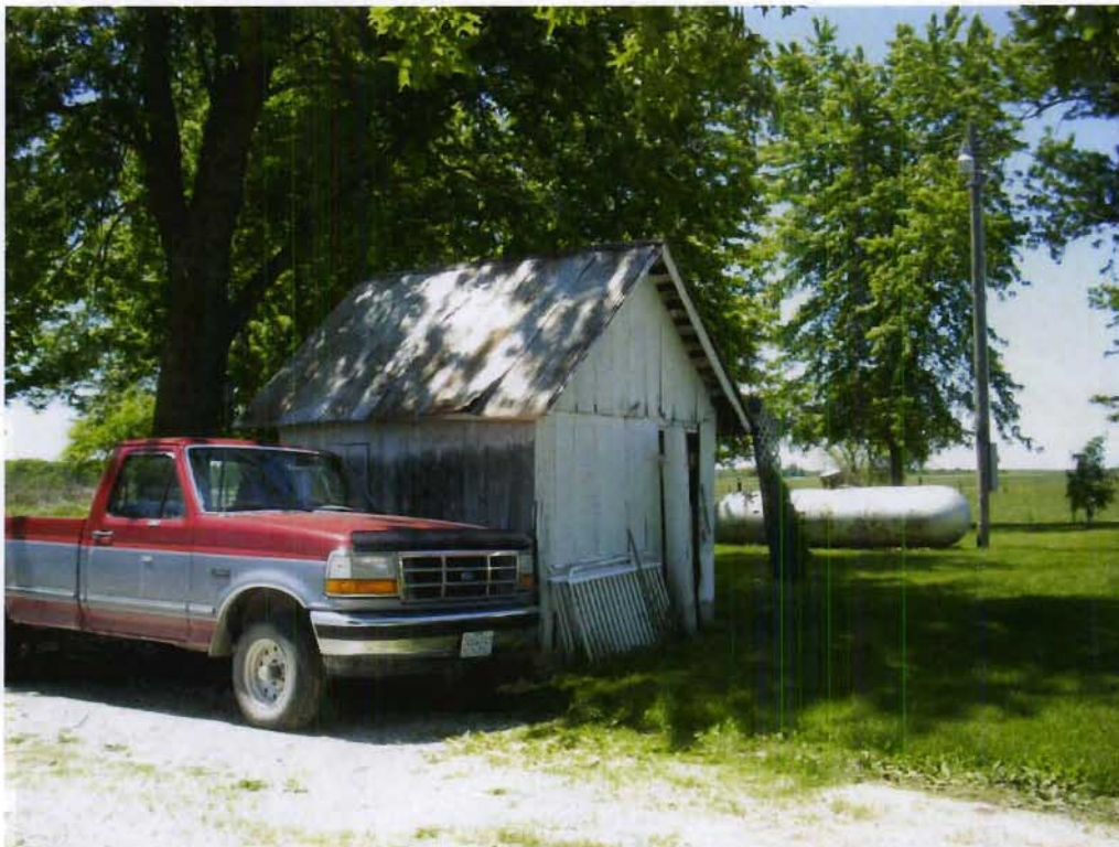
Structure 86d (Shed), view SW
