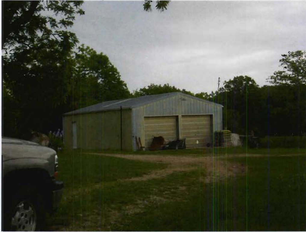
Structure 130b (Garage), view SE
