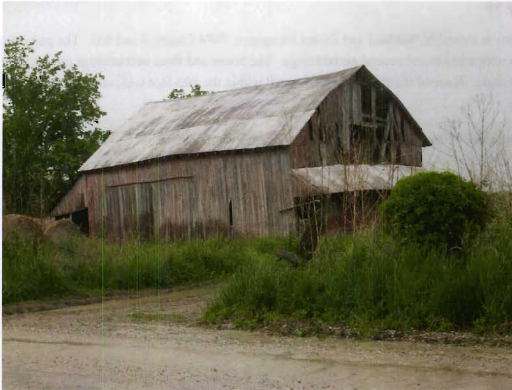
Structure 18a (Barn), view ENE
