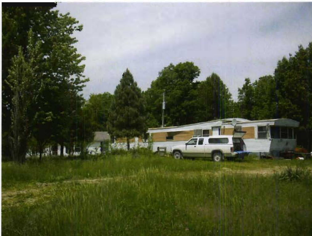
Structures 173a (House) and 173d (Mobile home), view WNW
