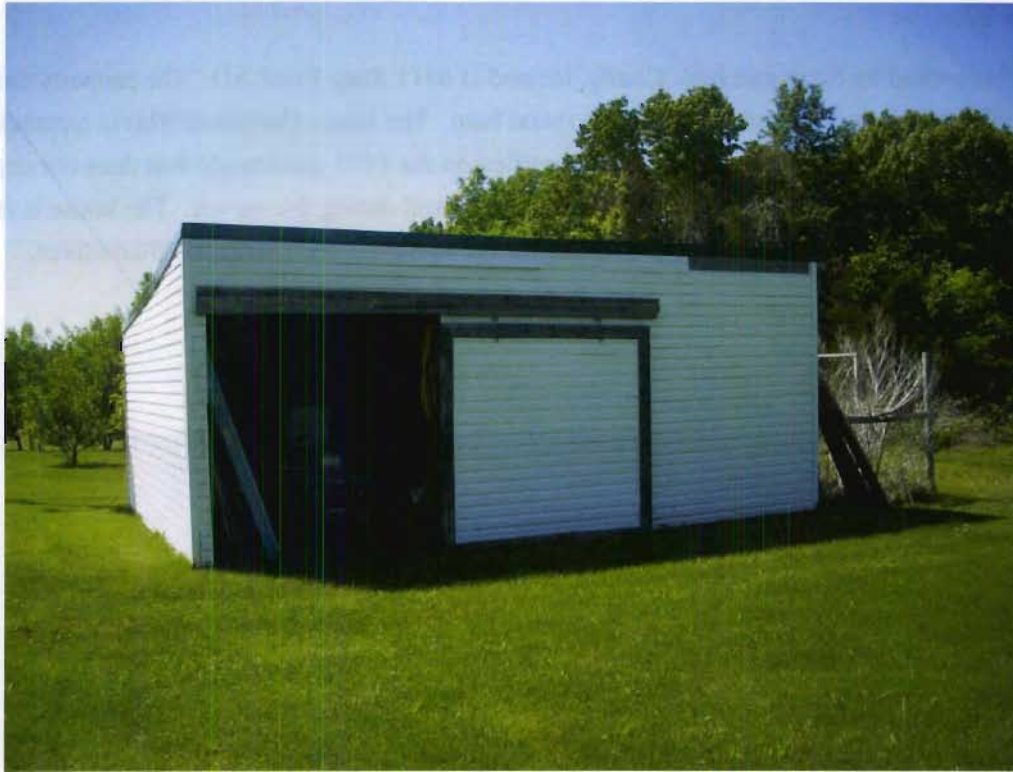
Structure 96b (Shed), view W
