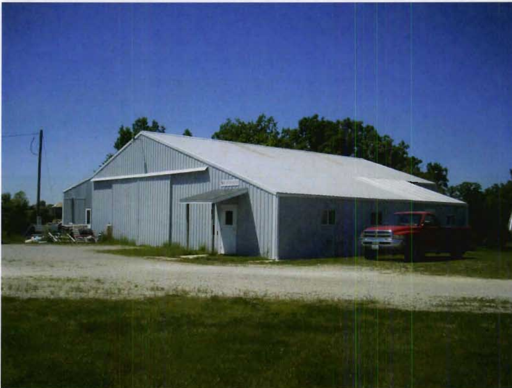
Structure 43f (Hay barn warehouse), view NW
