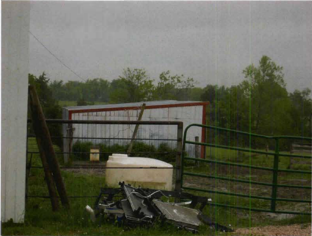
Structure 19d (Outbuilding), view N
