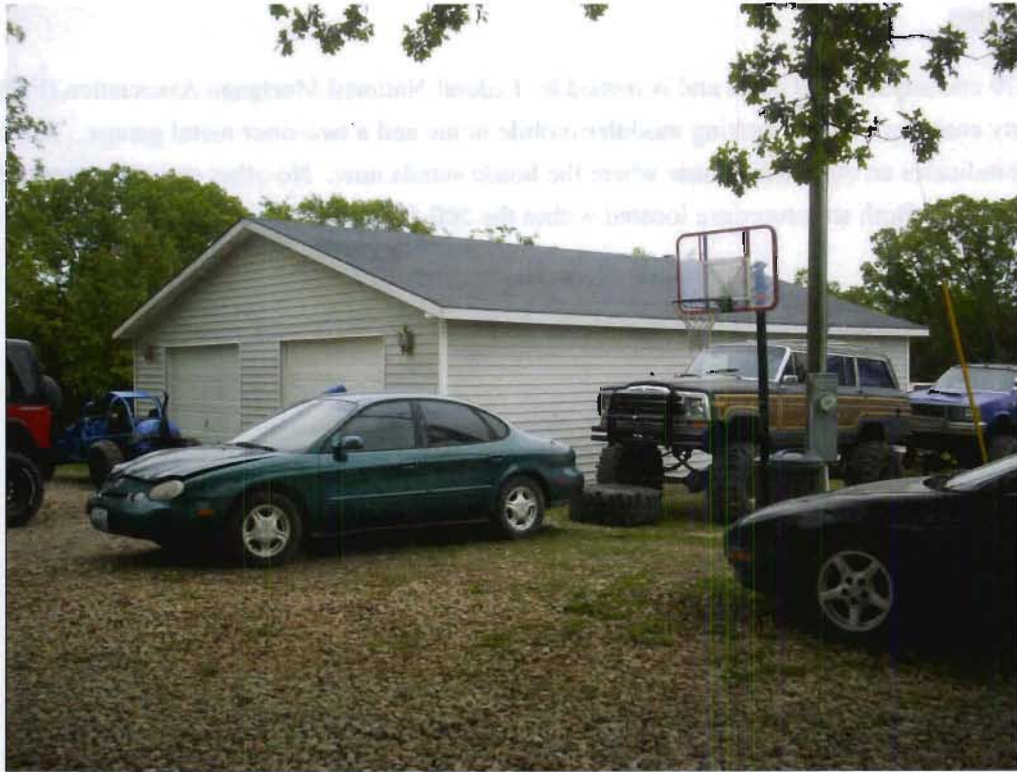
Structure 179b (Garage), view SE
