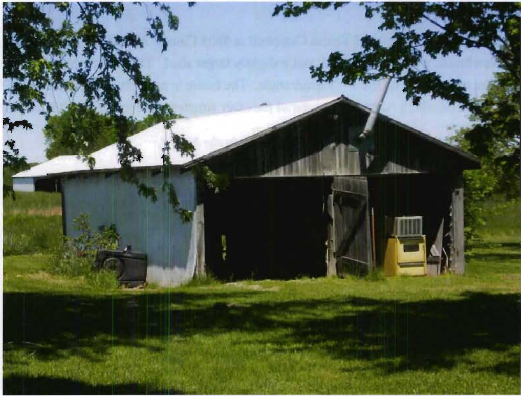
Structure 80c (Shed), view NW
