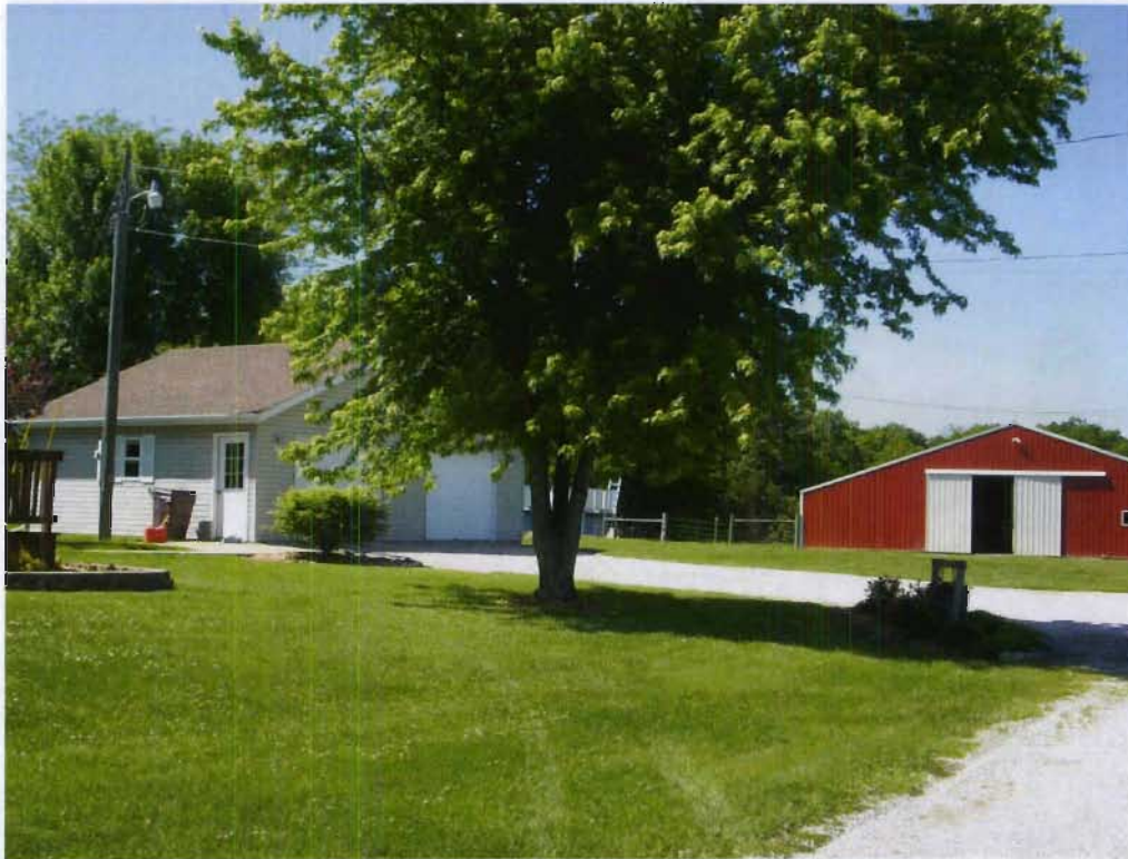
Structures 97b (Garage) and 97c (Barn), pictured from left to right, view NW
