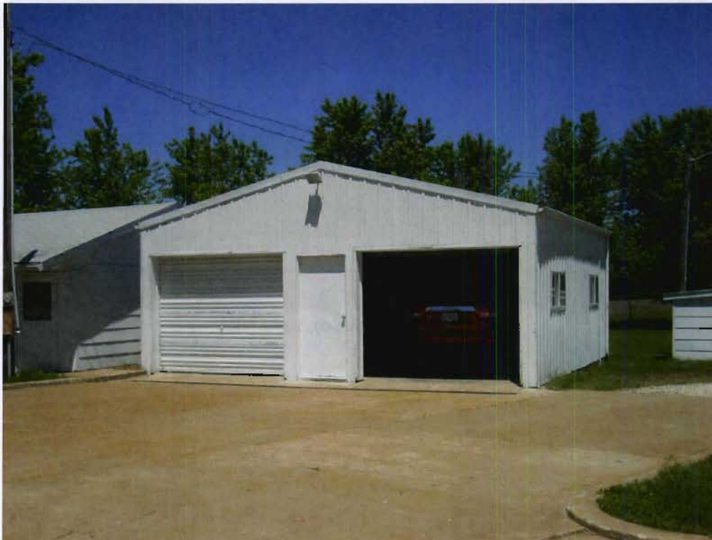
Structure 84c (Garage), view NW
