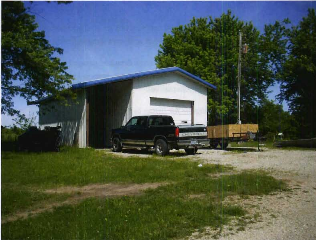
Structure 112b (Garage), view WNW
