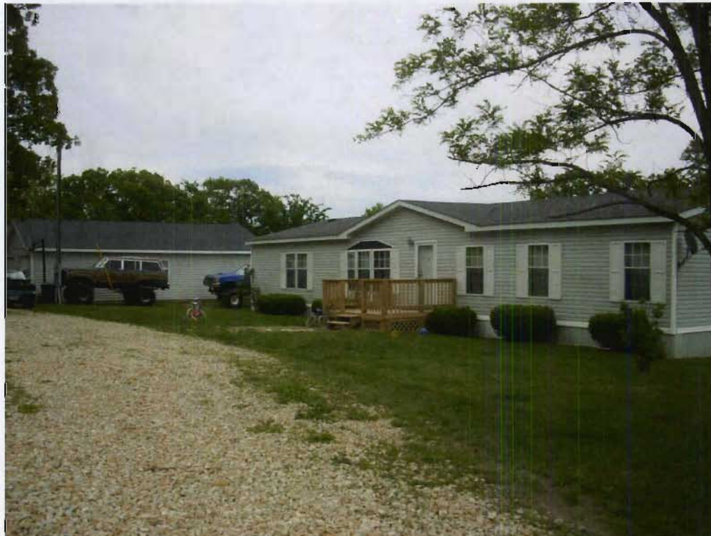
Structures 179a (House) and 179b (Garage), view SE
