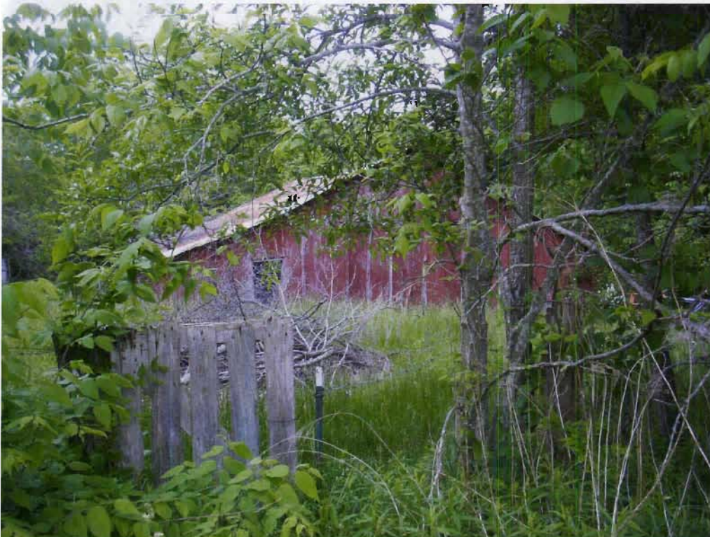
Structure 148b (Barn), view E
