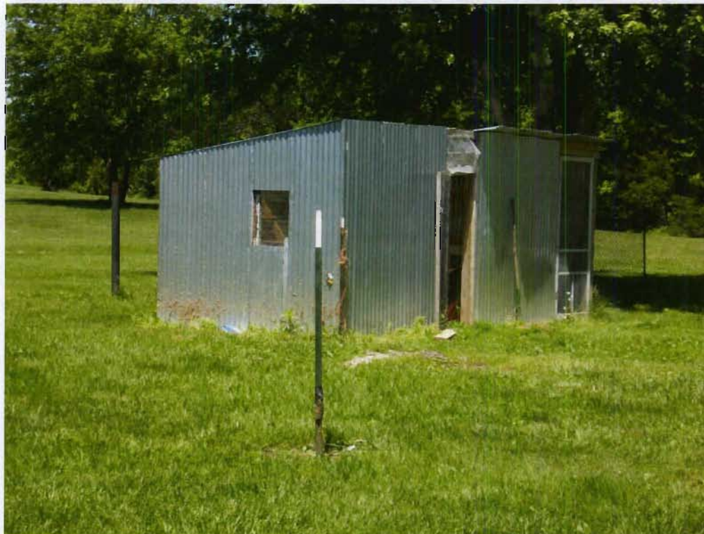
Structure 53c (Shed), view N
