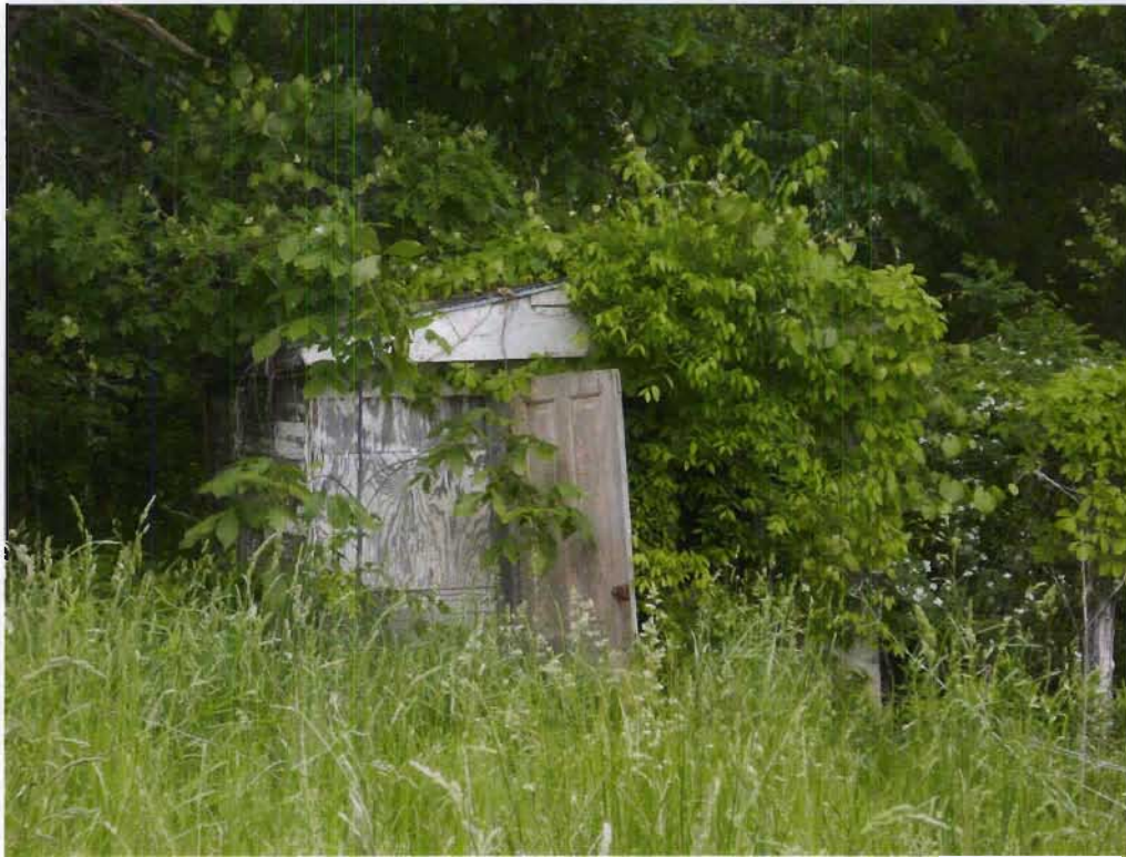
Structure 178h (Wooden shed), view W
