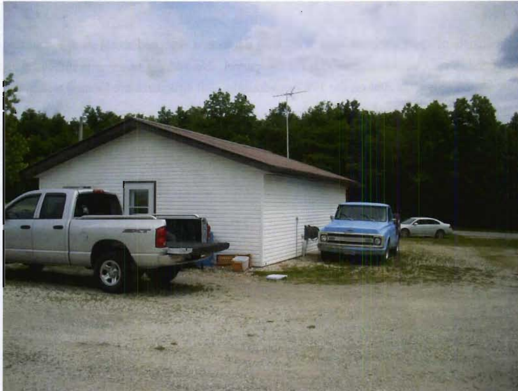
Structure 154b (Garage), view SE
