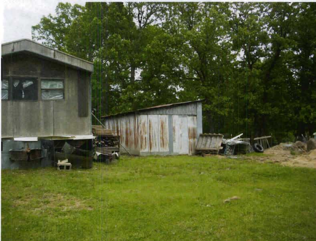
Structures 185a (Mobile home) and 185c (Detached metal shed), view SE
