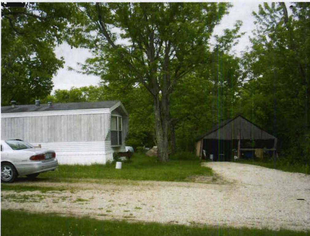
Structures 136a (Mobile home) and 136b (Shed), pictured from left to right, view S
