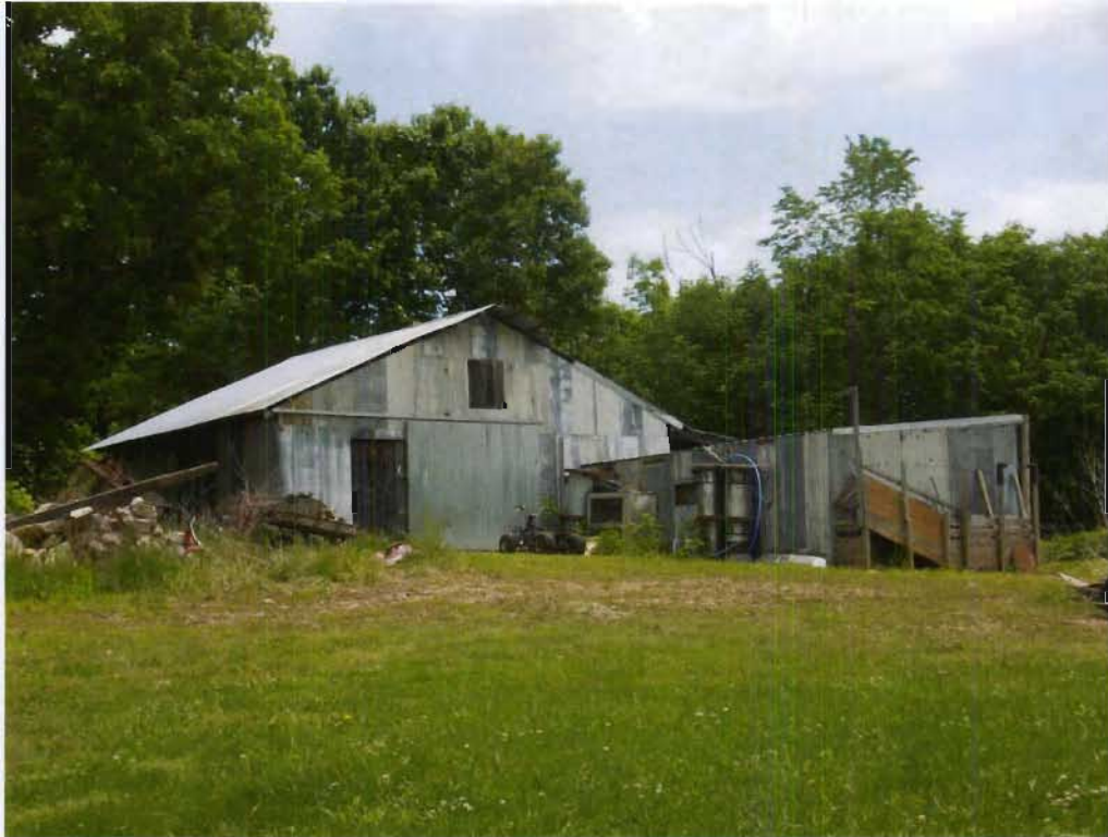
Structure 177a (Barn), view SE
