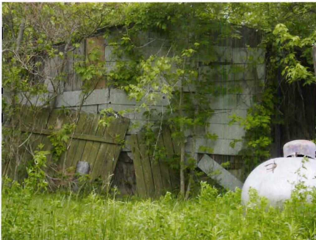
Structure 178g (Barn), view E
