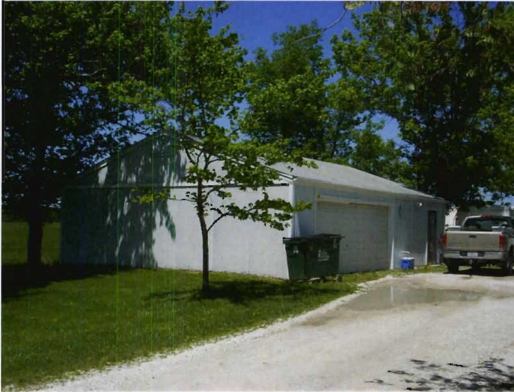
Structure 47b (One-door garage), view NW
