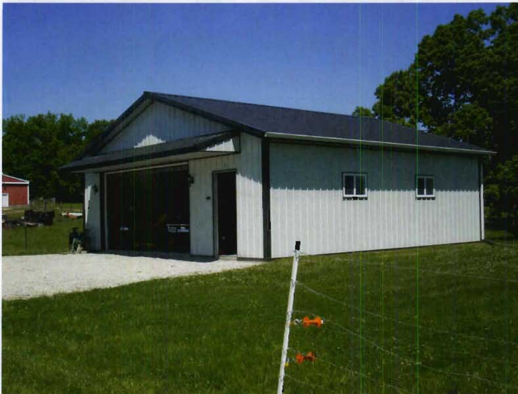
Structure 79c (Garage), view NW
