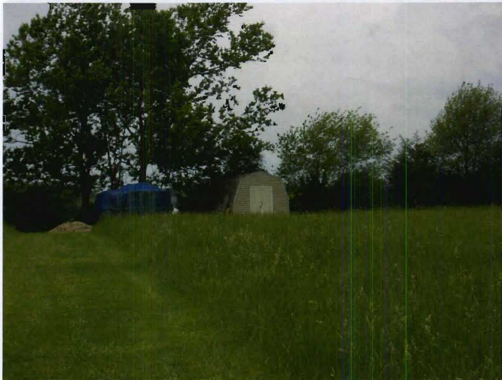
Structure 13c (Shed), view W
