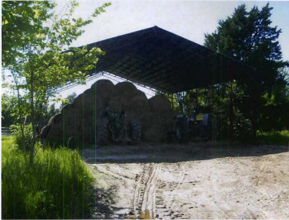
Structure 75d (Hay barn), view W
