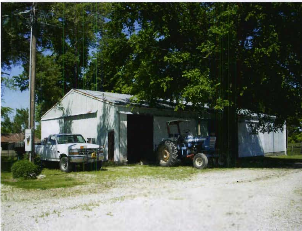
Structure 94g (Older Metal Barn), view NE
