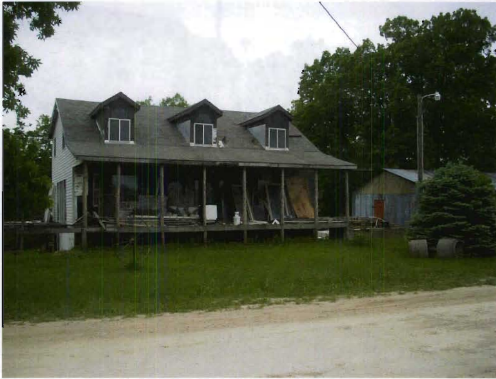
Structure 185f (House), view SW
