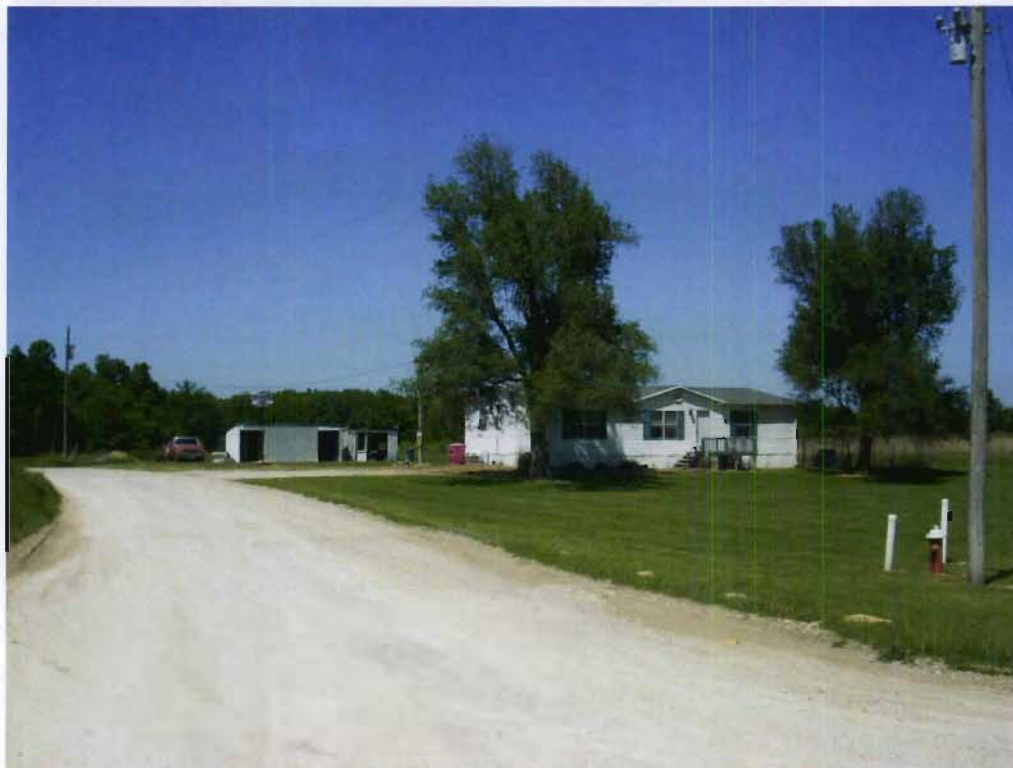
Structures 94b (Metal shed), 94c (metal shed), and 94a (mobile home), pictured from left to right, view NNW
