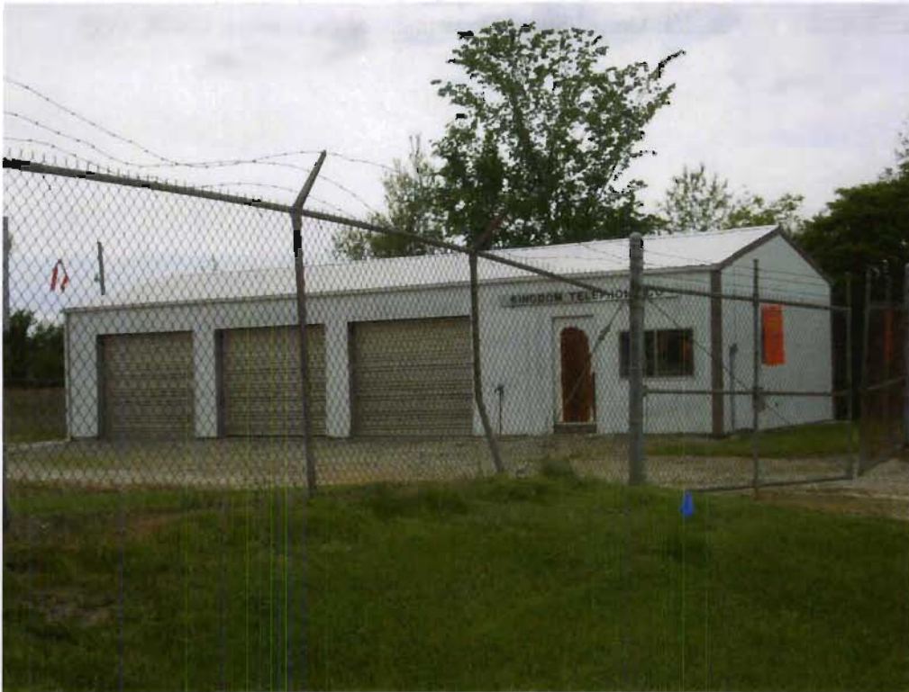
Structure 190a (Kingdom Telephone Company Garage), view SW
