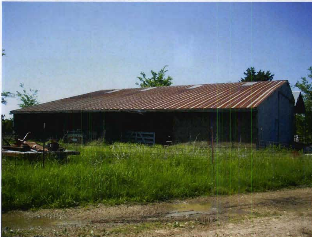
Structure 75c (Partially open barn), view NW
