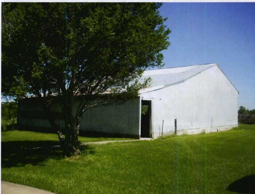
Structure 68c (Older metal shed), view SE
