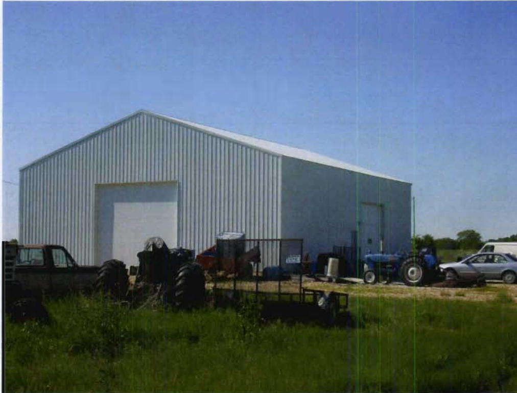
Structure 75i (Metal building), view NW
