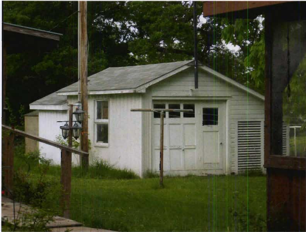
Structure 9d (Small wooden shed), view NE
