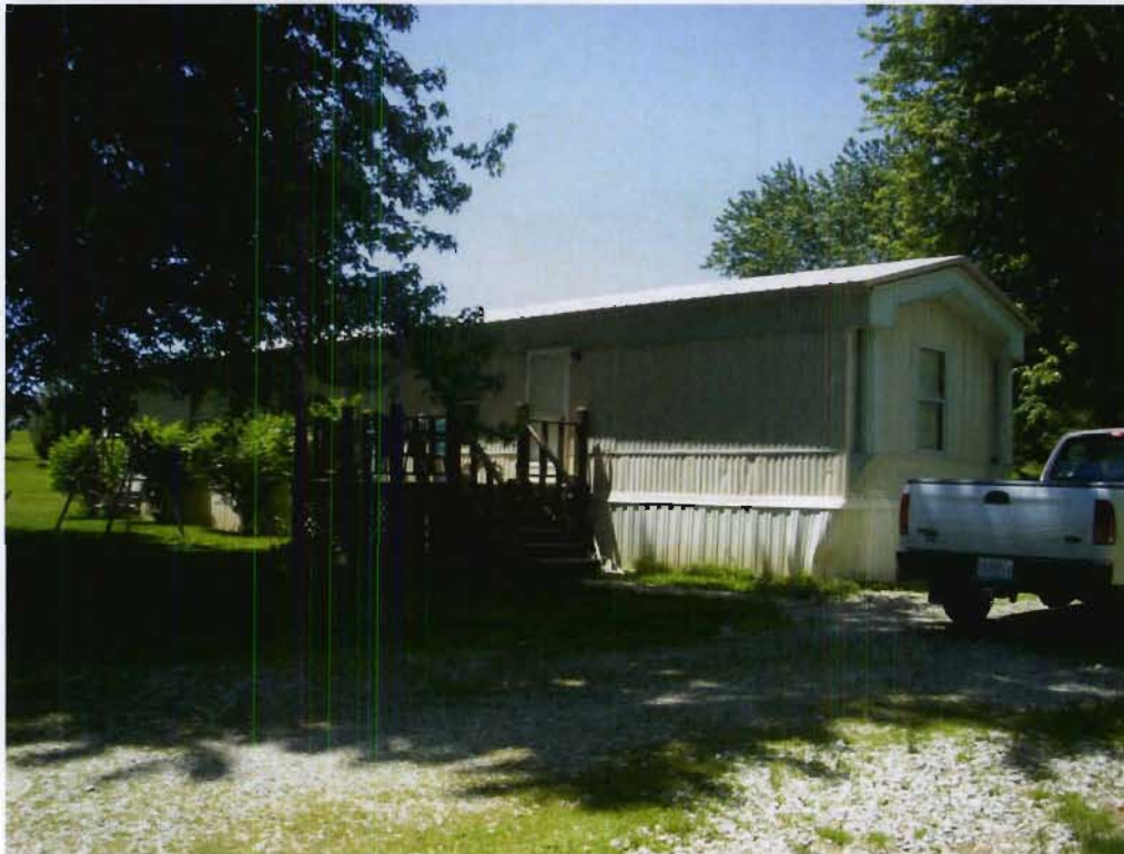
Structure 53a (Mobile home), view W
