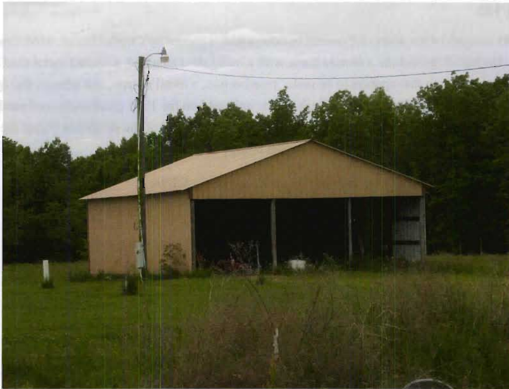
Structure 183b (Barn), view W
