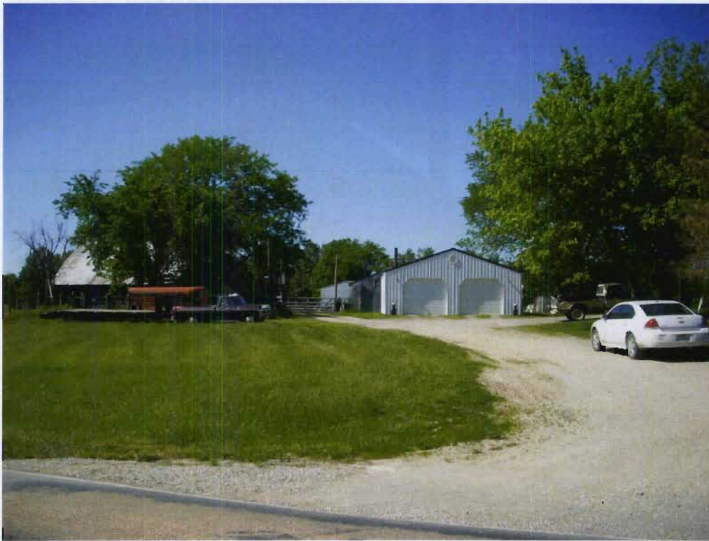
Property 104, general view NW
