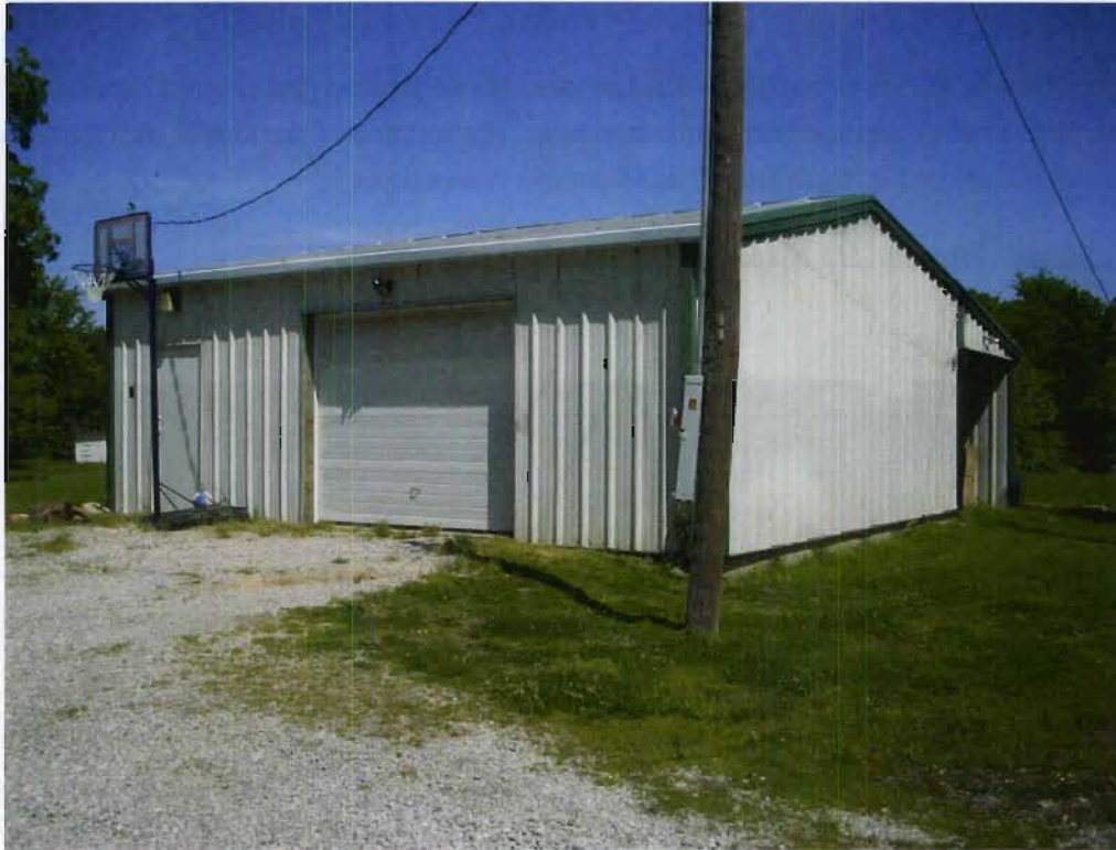
Structure 112e (Garage), view NE
