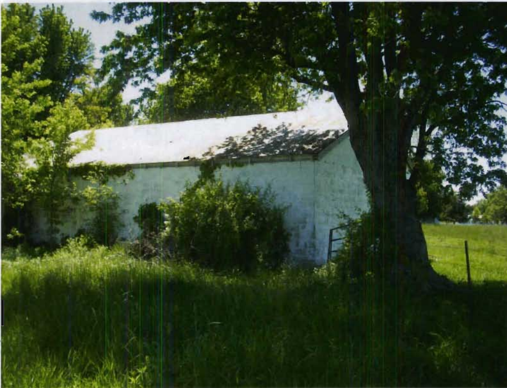
Structure 88c (Back of smaller structure), view SW
