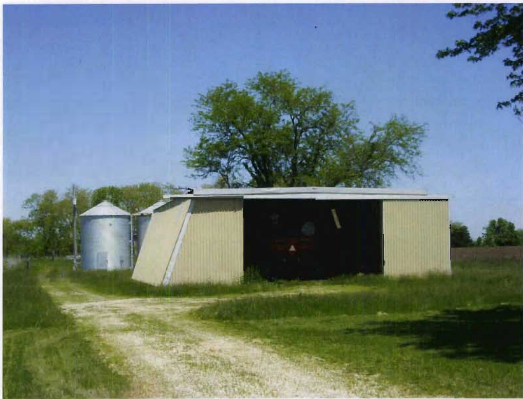
Structure 40c (yellow metal shed), view NE
