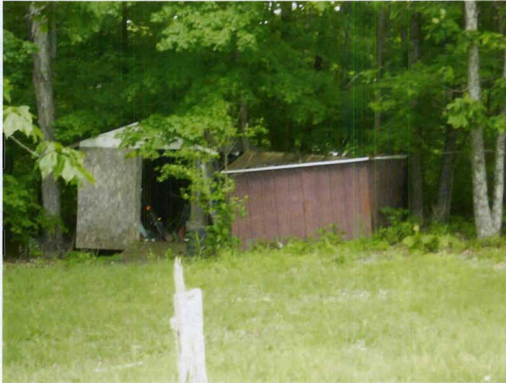
Structure 132b (Shed), view W
