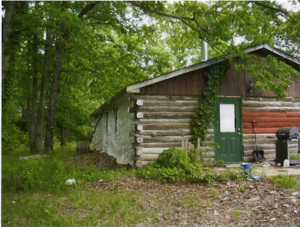
Structure 178a (House), view ESE
