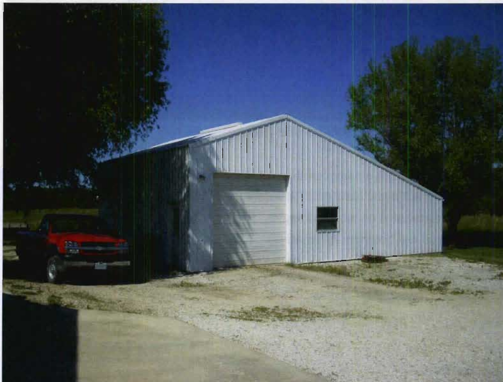
Structure 98c (Barn/shed), view NNW
