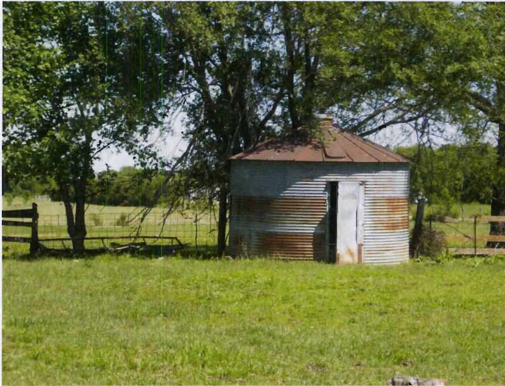
Structure 94f (Silo), view E
