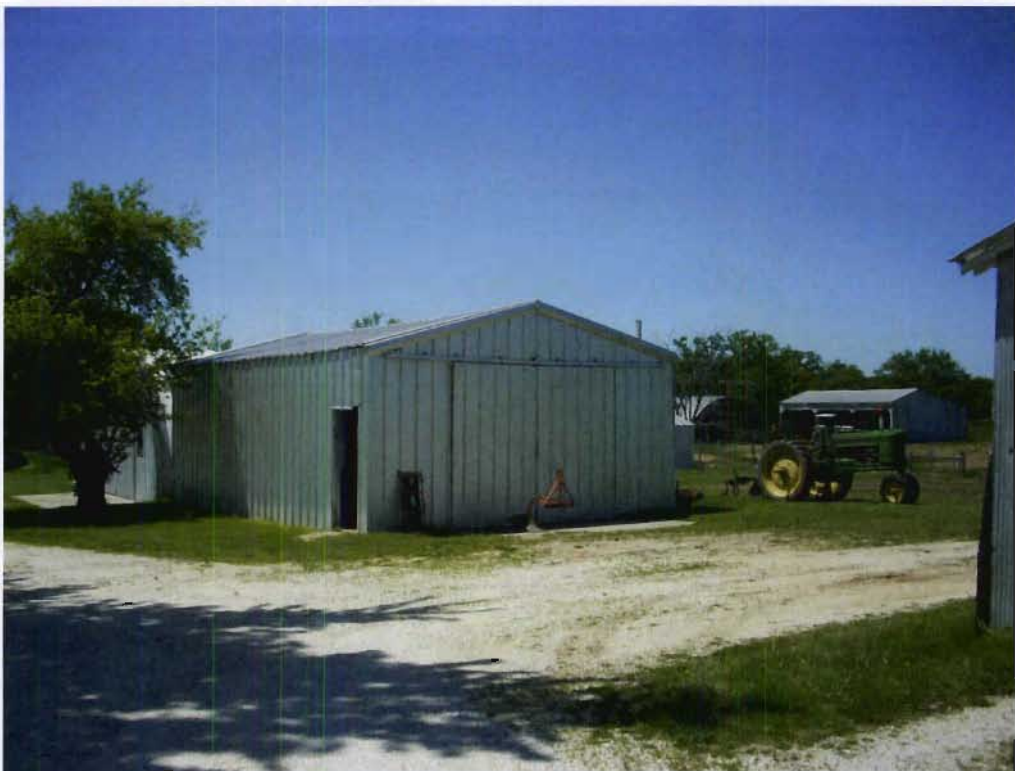
Structure 43e (Metal shed and Quonset building), view NW
