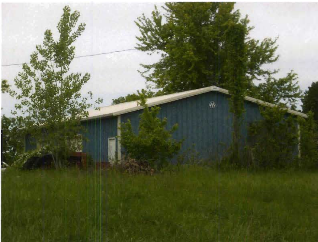
Structure 178i (Metal shed/workshop), view NE
