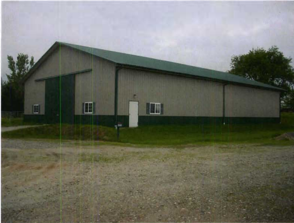
Structure 30a (Commercial building), view SSE
