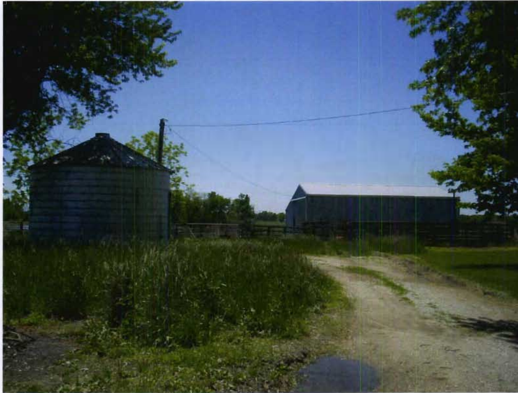
Structures 86b (Barn) and 86c (Silo), view S
