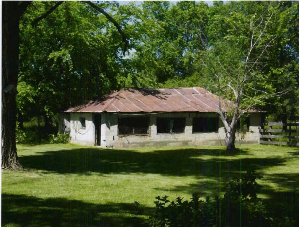
Structure 94h (Cinderblock chicken coop), view NE
