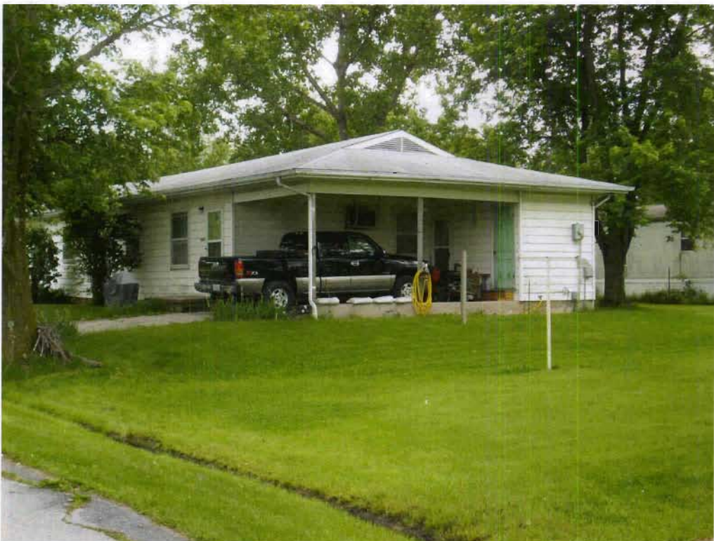
Structure 9e (Duplex), view S
