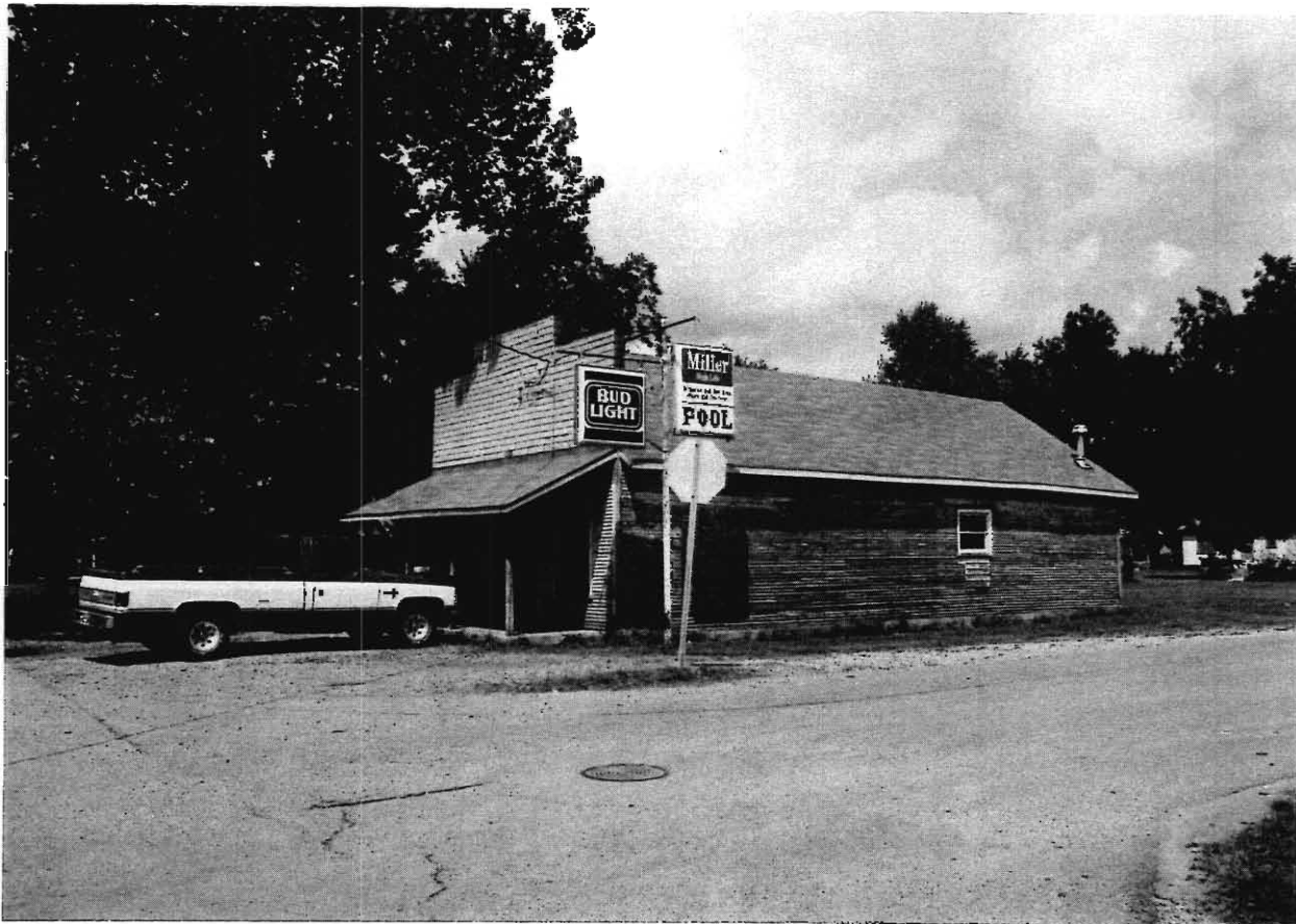
Figure 4. False front commercial building. BU-FI-1 Fisk.
