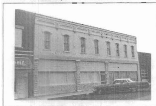
Below: Two-Part Commercial Block Form With Italianate References in Cornice and Arched Windows, 211 N. Main Street.
