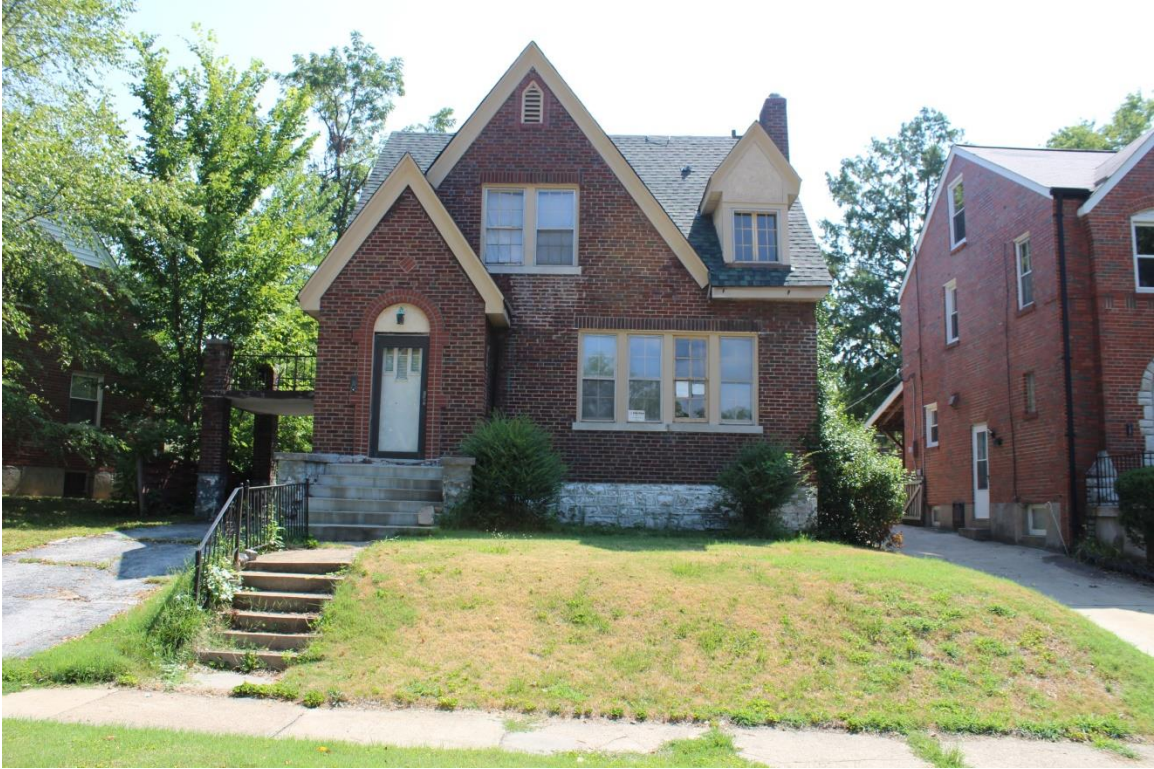
Figure 13. 3072 Arlmont Drive, view is east; photo courtesy of St. Louis County Parks.
