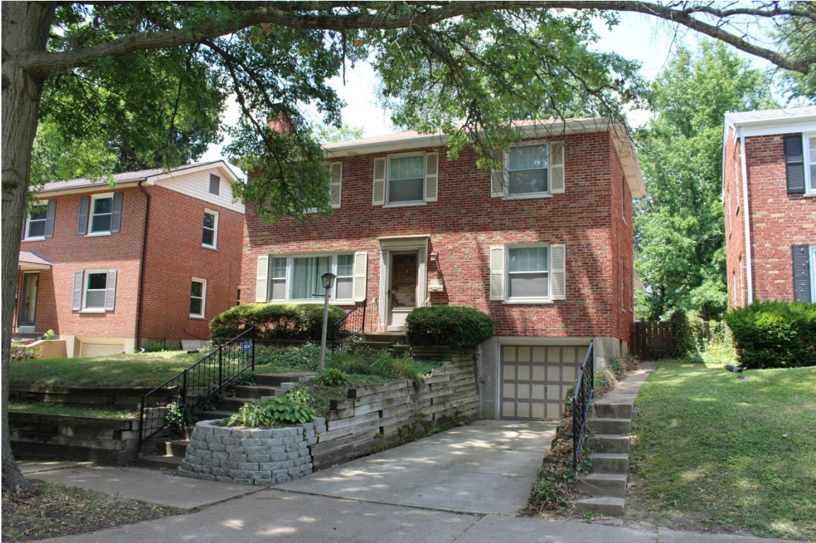
Figure 19. 2919 Delavan Drive was constructed in 1955 and has a basement level garage. Photo courtesy of St. Louis County Parks, view is northeast.
