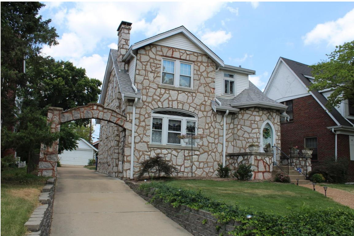
Figure 21. An Ozark (“giraffe”) pattern stone dwelling at 8017 Glen Echo Drive is a striking addition to the neighborhood’s architectural offerings. Photo courtesy of St. Louis County Parks. View is northeast.
