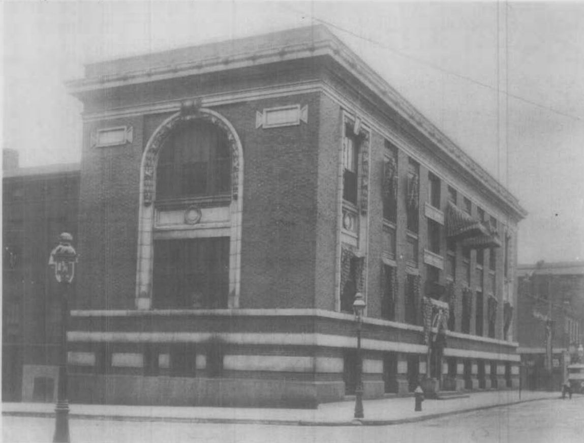
Figure 2: Beaumont Telephone Exchange. Circa 1903. Courtesy of SBC Archives and History Center, San Antonio, Texas.
