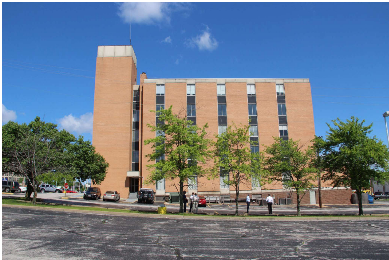
Figure 15. Strips of grass with trees and shrubs are interspersed in the parking areas near the bank. View is west. (Photo: Keenoy, 13 June 2019).
