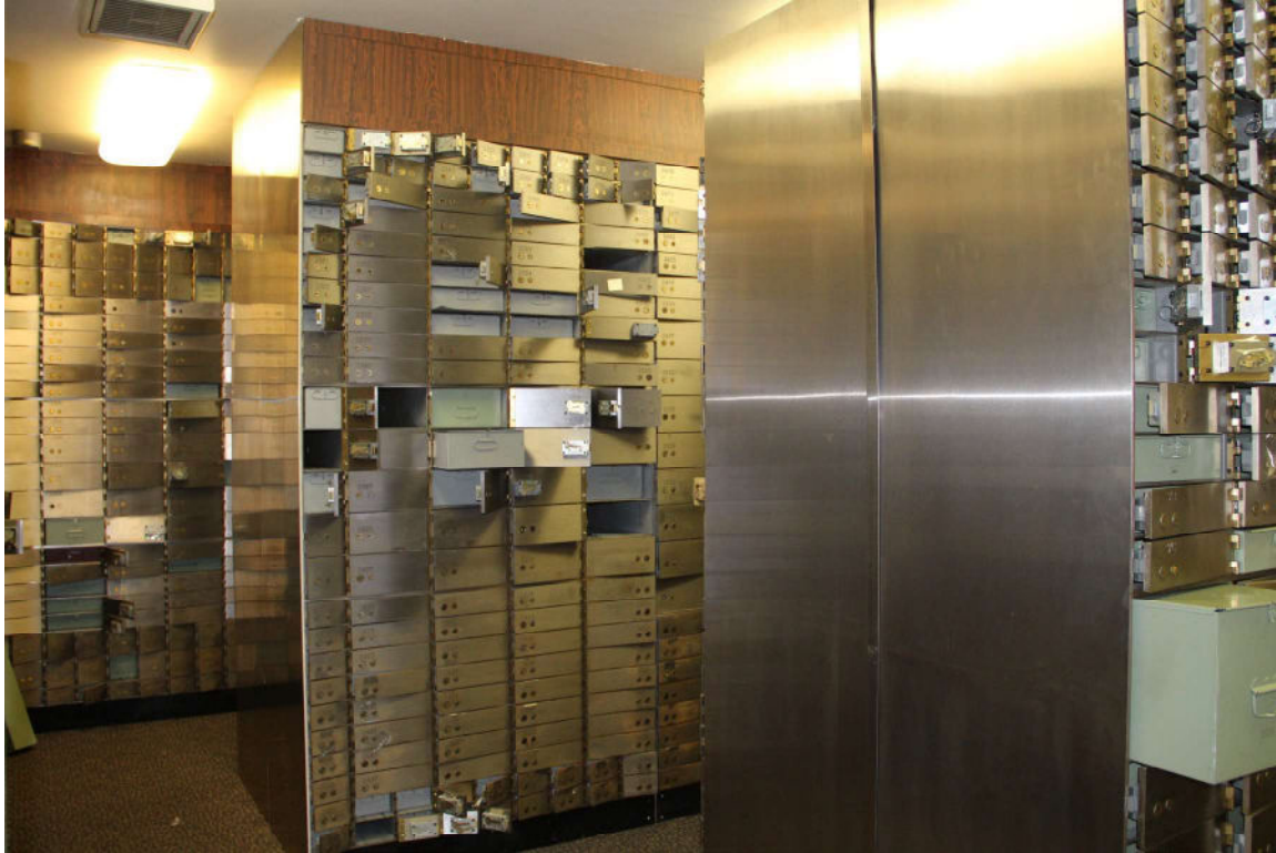
Figure 4. Safe deposit boxes inside the original bank safe (Photo: Keenoy, 13 June 2019).
