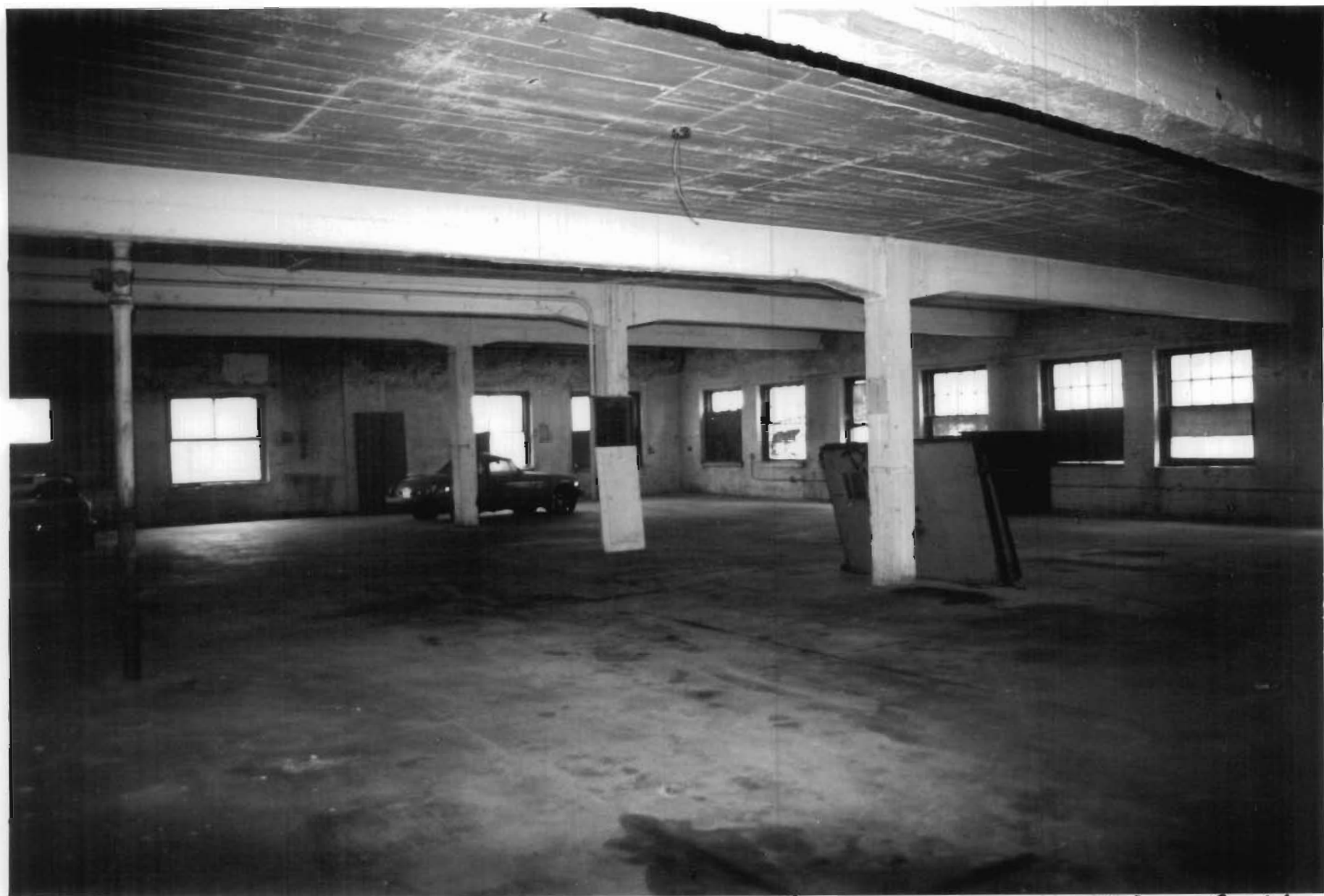
Autocar Sales and Service Building St. Louis (Independent City), Mo. Photo # 8
