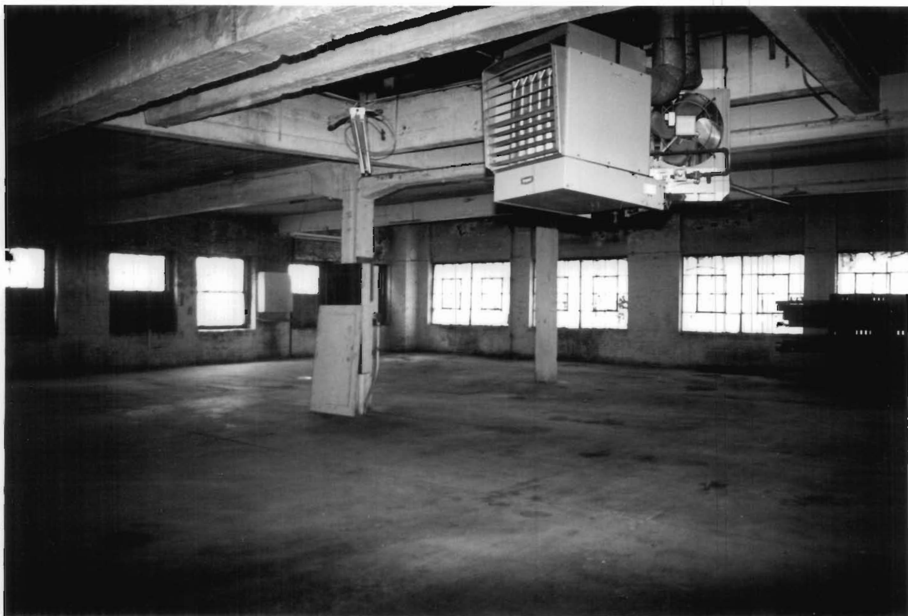
Autocar Sales and Service Building St. Louis (Independent City), MO, Photo # 9
