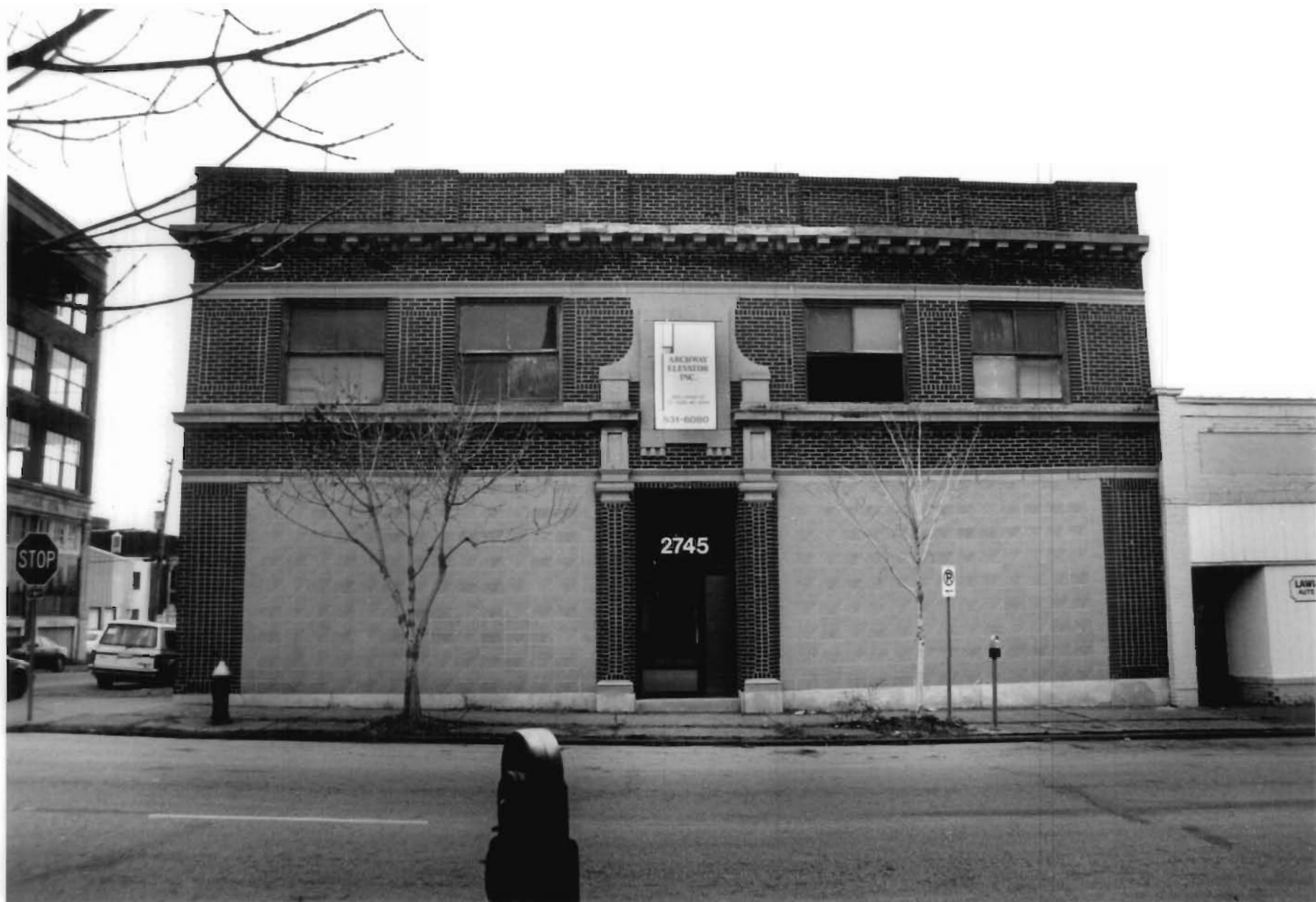
Autocar Sales and Service Building St. Louis (Independent City), MO. Photo # 1
