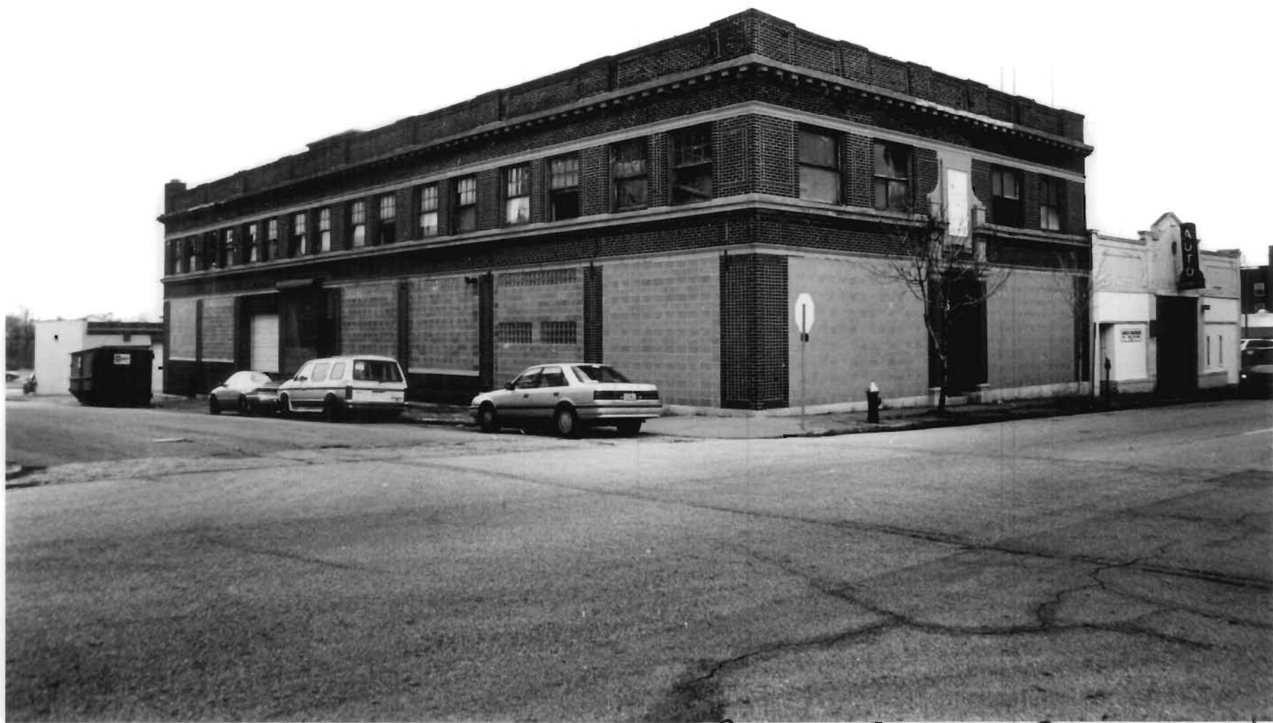
Autocar Sales and Service Building St. Louis (Independent City), MO. Photo #2
