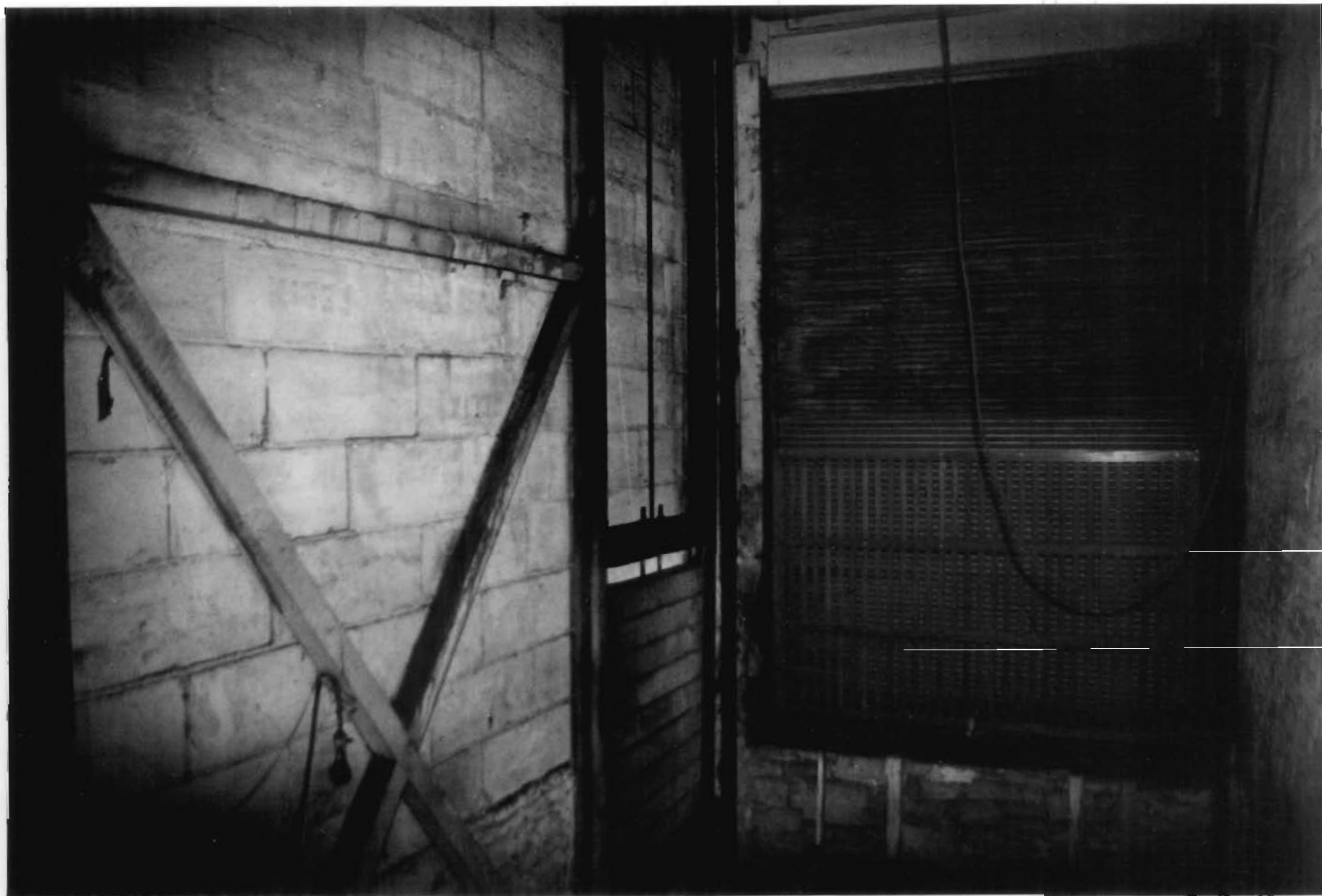
Autocar Sales and Service Building St. Louis (Independent City), MO, Photo # 6
