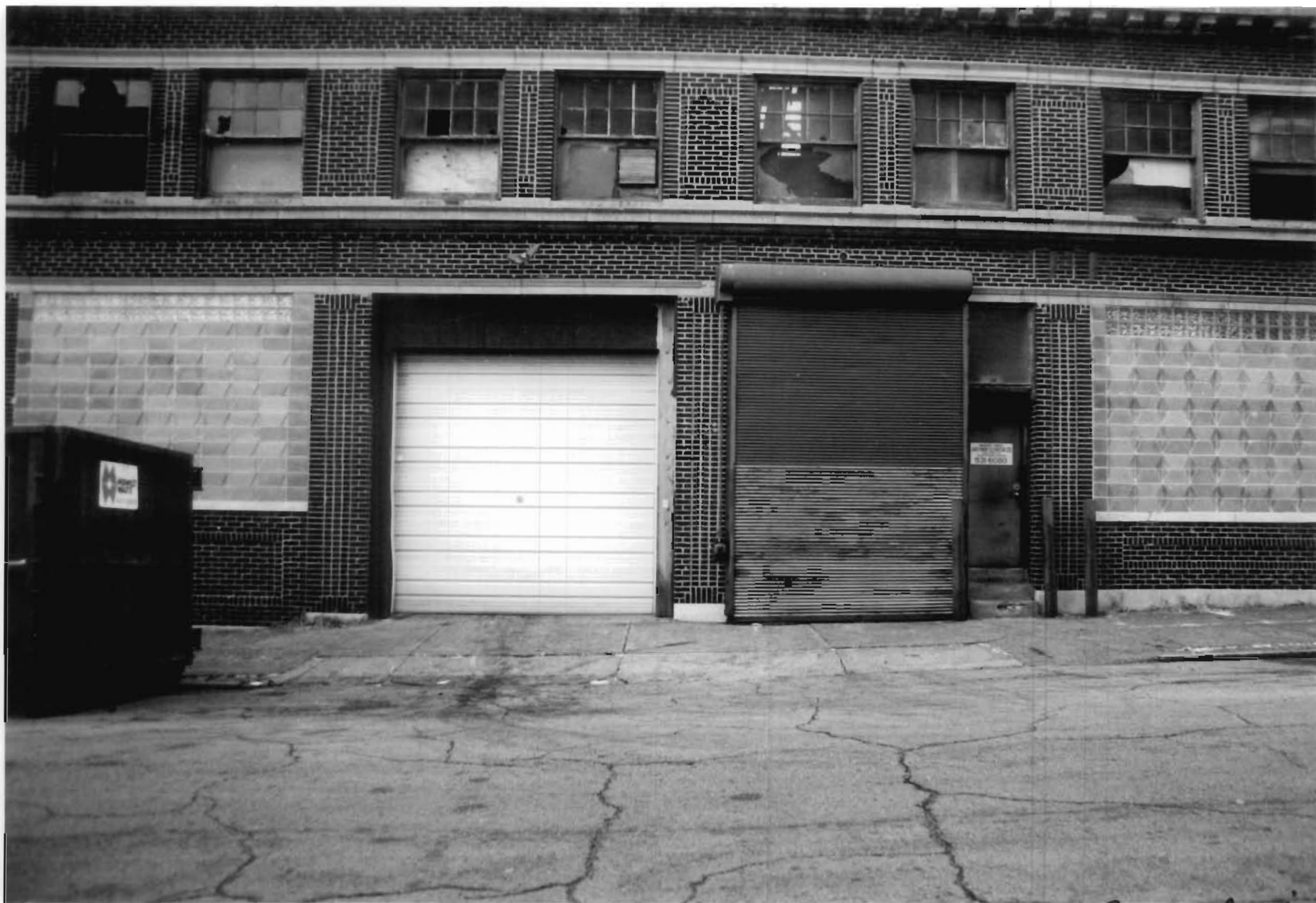
Autocar Sales and Service Building St. Louis (Independent City), MO. Photo # 4
