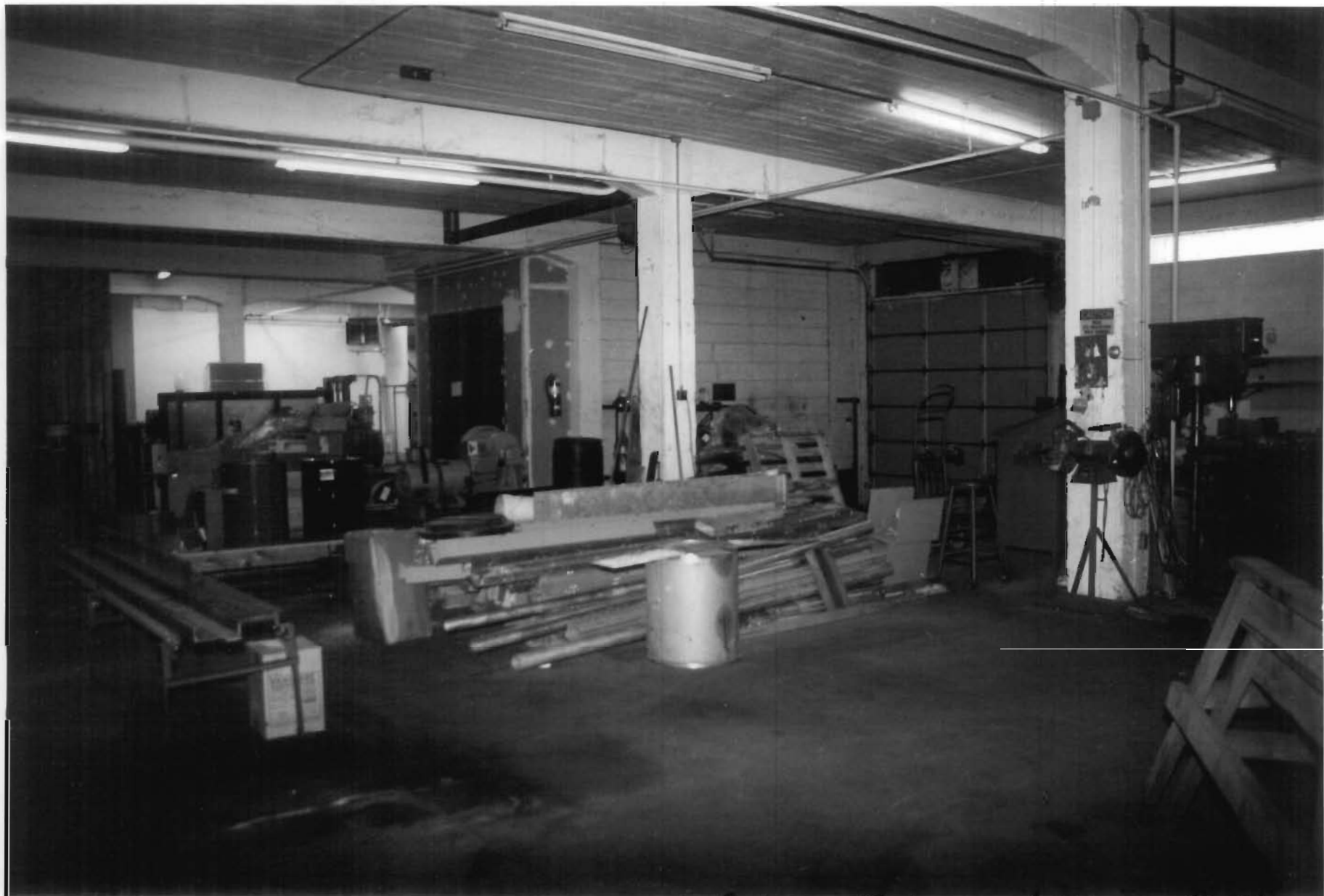
Autocar Sales and Service Building St. Louis (Independent City), MO. Photo # 5
