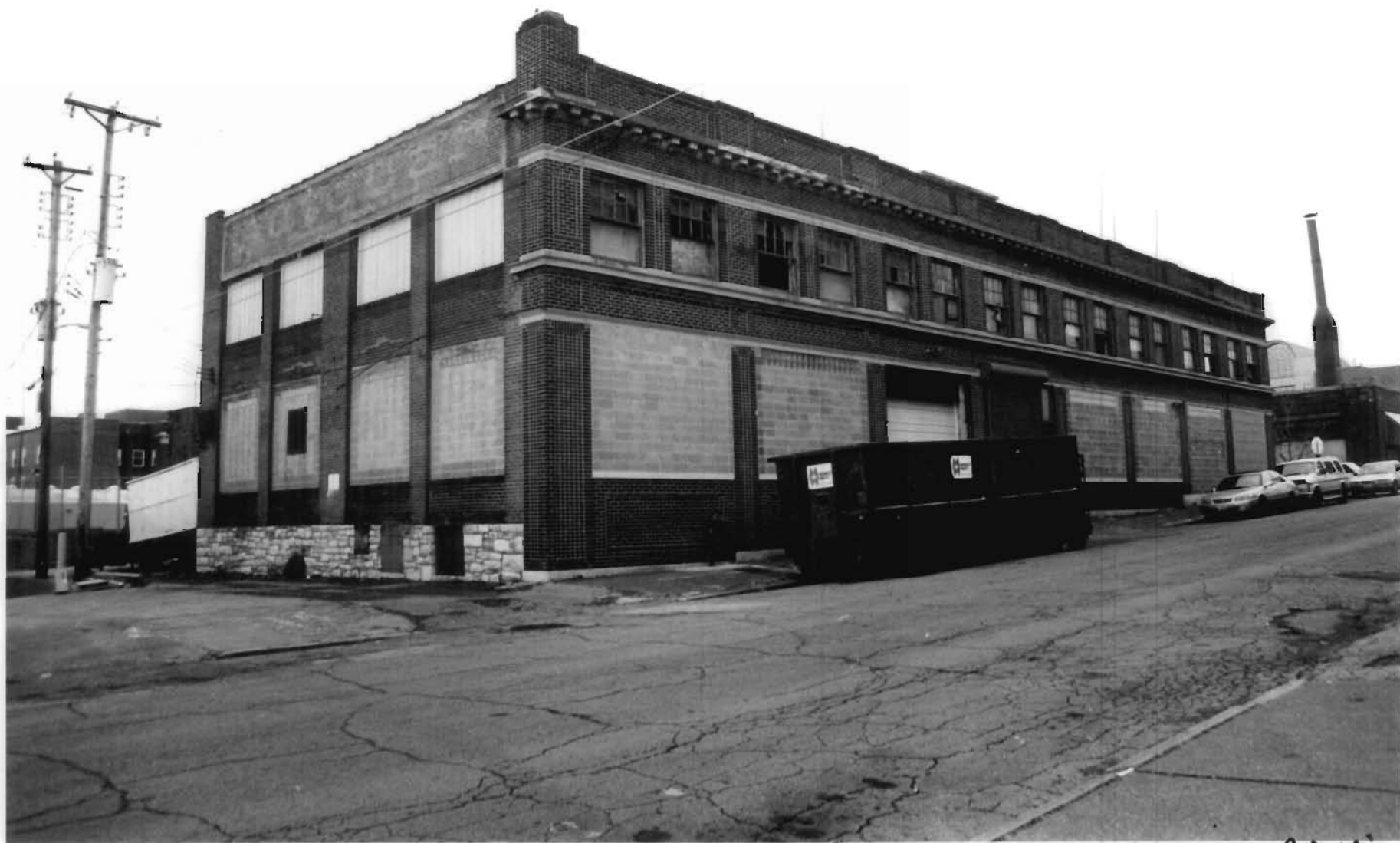
Autocar Sales and Service Building St. Louis (Independent City), MO Photo # 3
