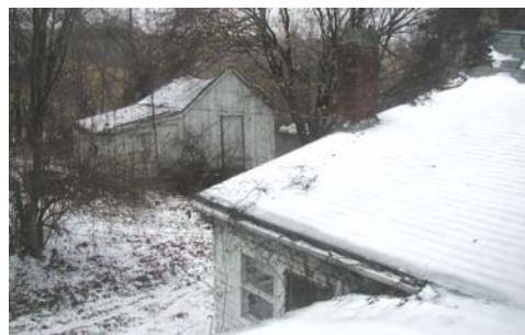
Milk House, View to the North
