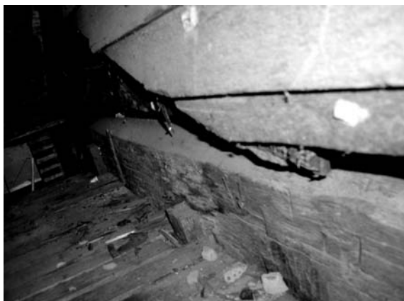
Cap Logs at Floor Level, East Attic
