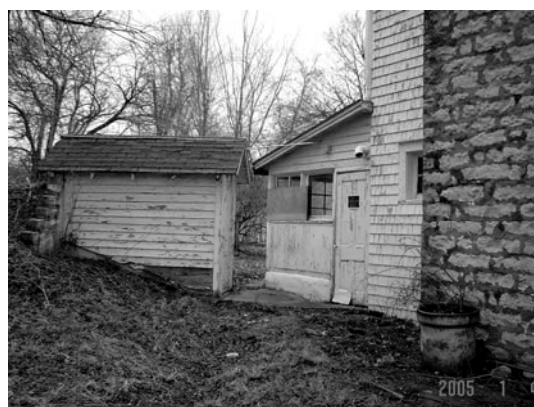
Root Cellar, South Elevation
