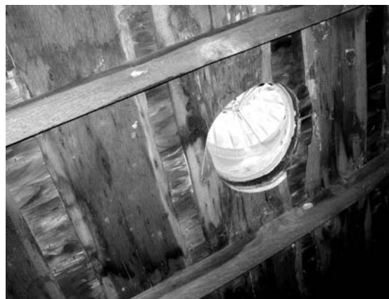
Sawn Roof Sheathing and Rafters, West Attic
