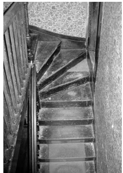
Stair Turn View to the North
