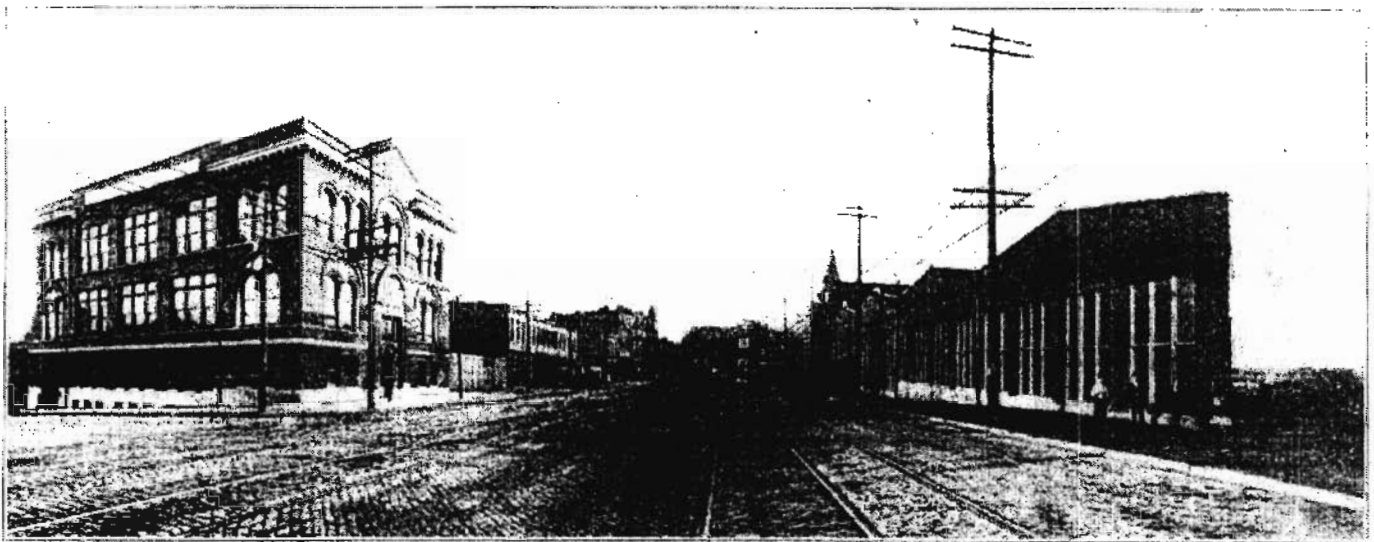
American Brake Company Offices, 1932 N. Broadway
