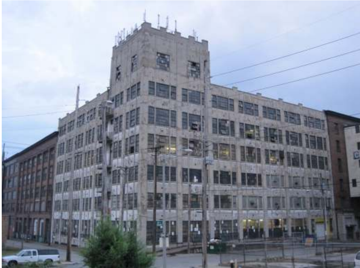
Figure 7: Crunden-Martin Building (1920, Tom P. Barnett). Photograph by the preparer.
