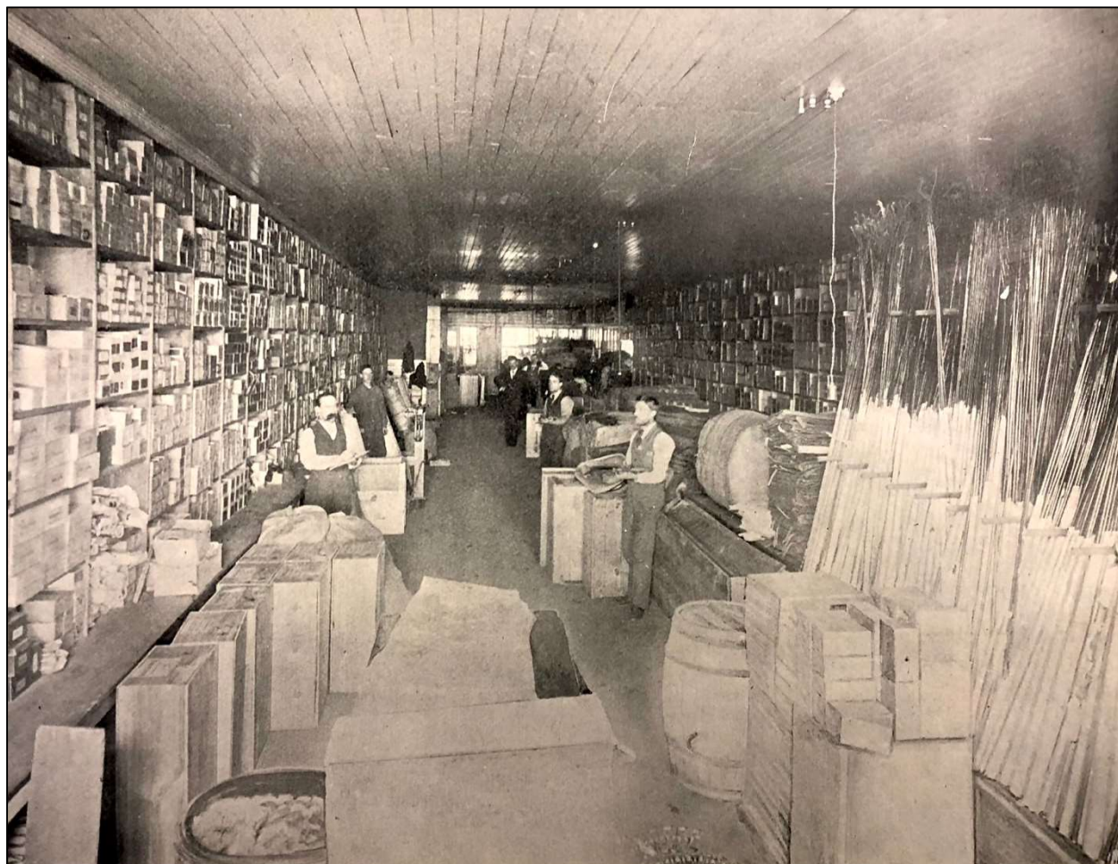
Figure 14: 1311-1315 W. 13 th Street, Interior. Saddlery Hardware Department, 1898
