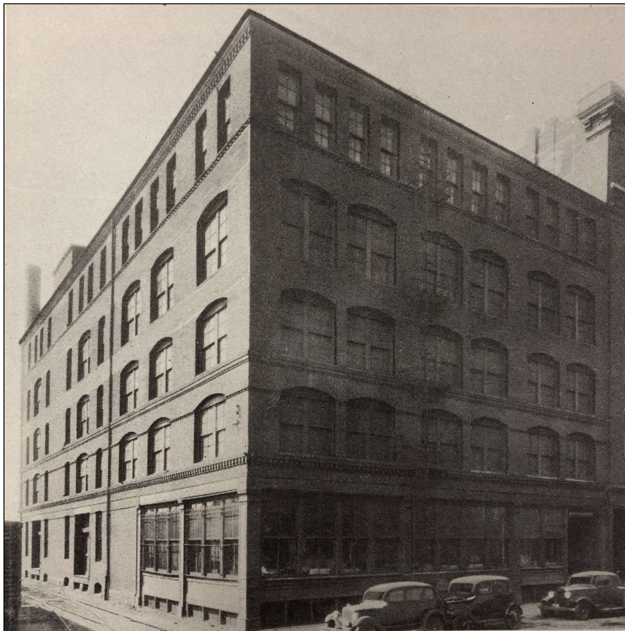
Figure 22: The Charles Francis Adams, Jr., Building as it appeared c. 1940
