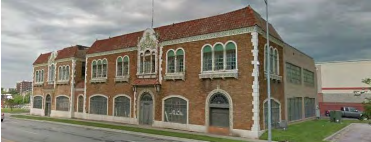
Figure 23. Luzier Cosmetics Building at 3216 Gillham Plaza completed in 1928. Source: Google maps 2016.
