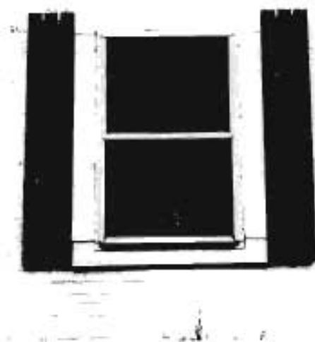
African American School Detail: window, north side
