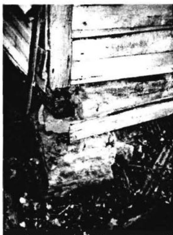
Concord/Liberty School Detail: pier, northeast corner
