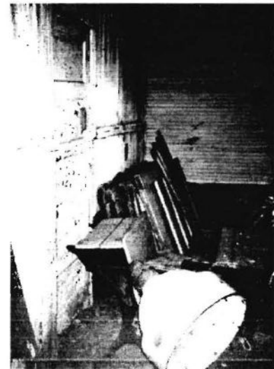
Concord/Liberty School Interior: cloak/entrance room
