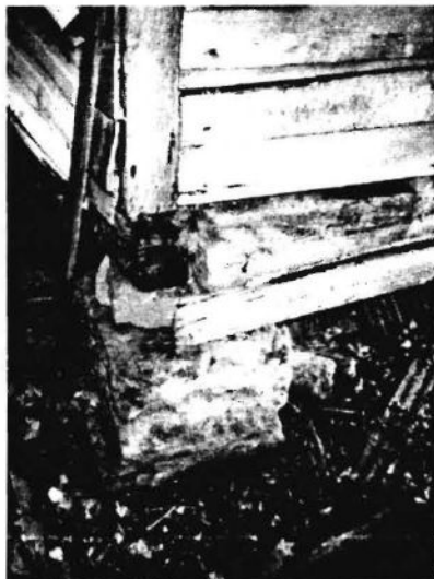
Concord/Liberty School Detail: pier, northeast corner
