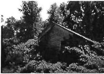
Grant School Clarksville, Mo. View from north
