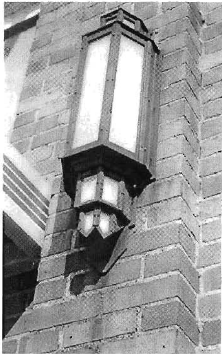
Lincoln School Period light fixture flanking entrance
