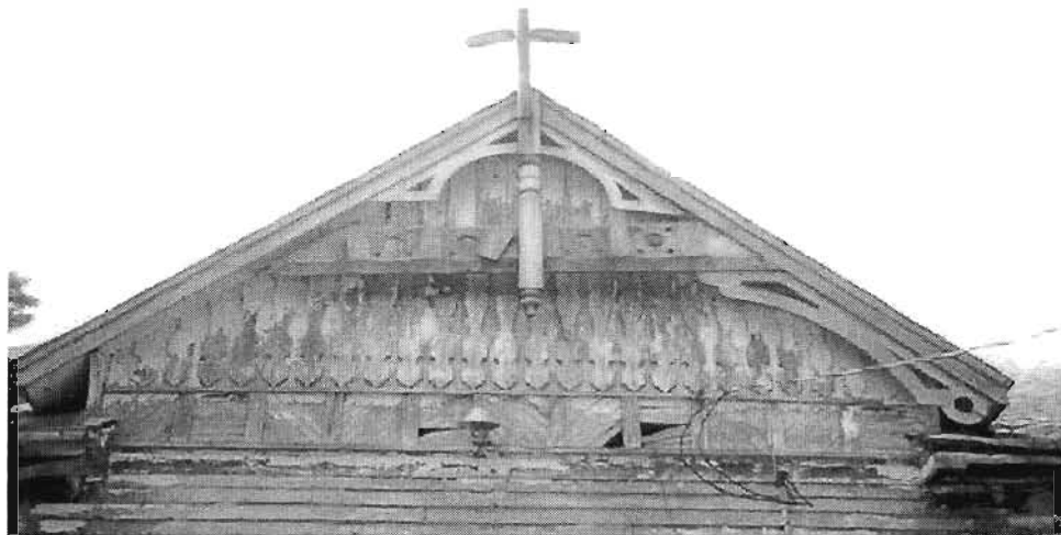
Howard School Detail of front gable
