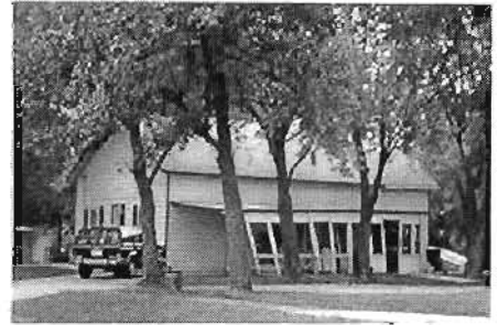
Lincoln School View from southwest
