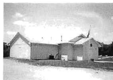
Dunbar School View from southwest
