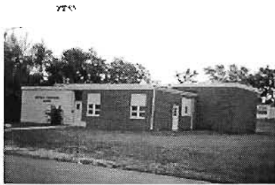
Dumas School, Macon MO. View from southwest
