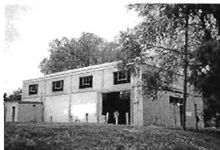
Lincoln Gymnasium Louisiana, MO. View from southwest
