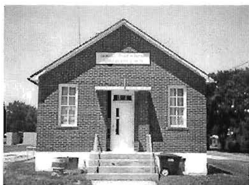
Washington School View from east: facade
