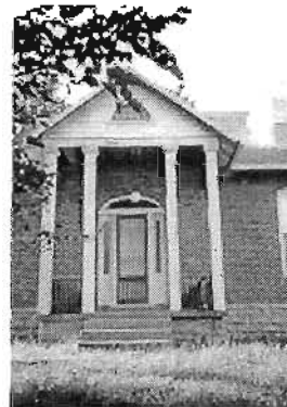
Banneker School View from south: facade
