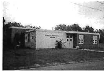
Dumas School View from northwest
