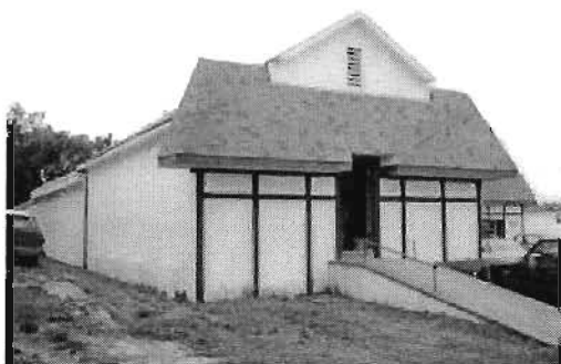
Lincoln School. Wentzville, MO. View from southwest.
