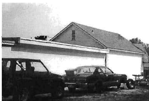
Lincoln School. Wentzville, MO. View from northwest.
