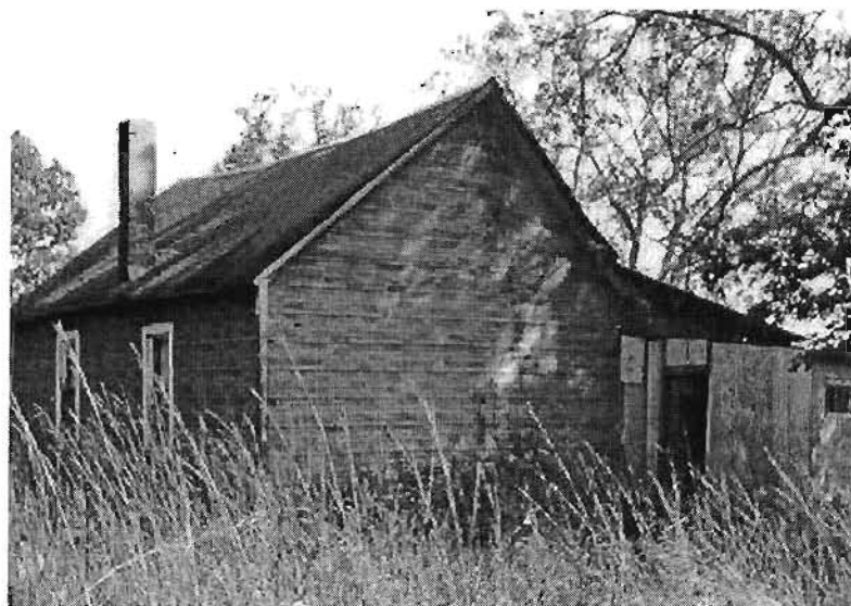
Crow's Fork Baptist Church. View from northwest.
