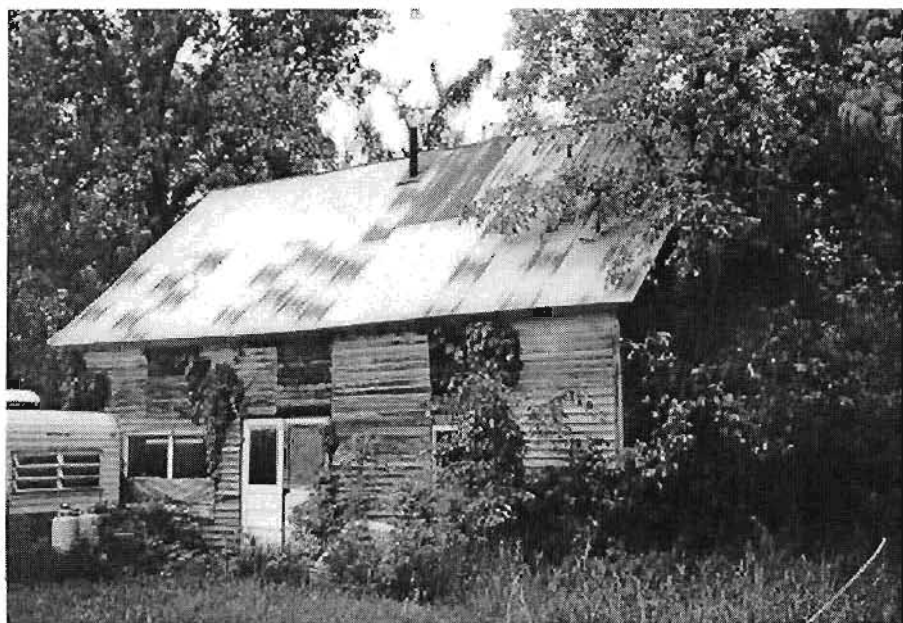
Nelson Colored School. View from northeast.
