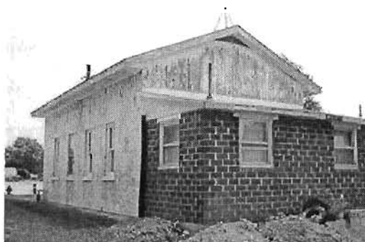
Lincoln School View from northwest.
