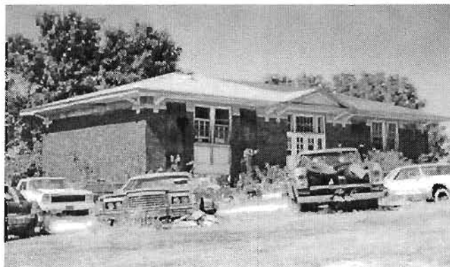
Douglass School, Higginsville, MO. View from southeast.
