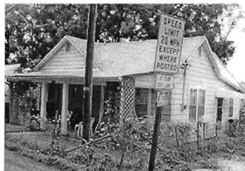
Dunbar School. View from southeast.
