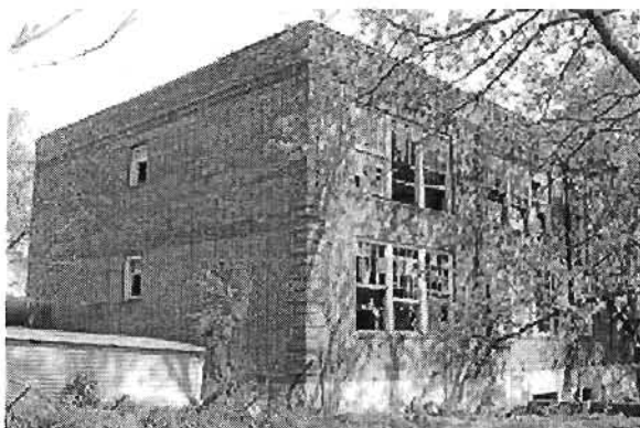
Bartlett Building. View from northwest.
