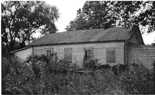
Lincoln School. View from northwest.
