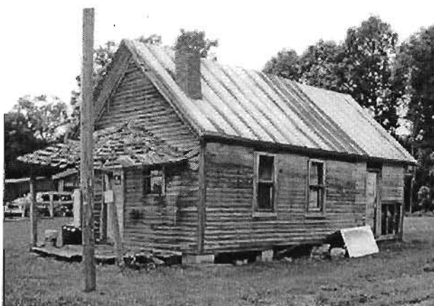
Gregory School. View from northeast.
