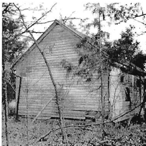
Douglass School. View from north.
