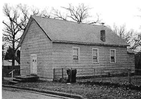
Good Hope Baptist Church. View from northwest.
