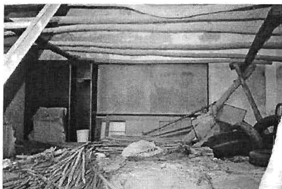
Bartlett Building. Interior: classroom.
