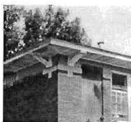
Douglass School. Detail: triangular knee braces, windows and wide eaves.
