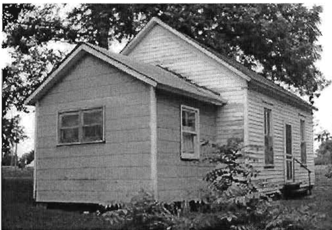
Lincoln School, Gilliam, MO. View from northeast.
