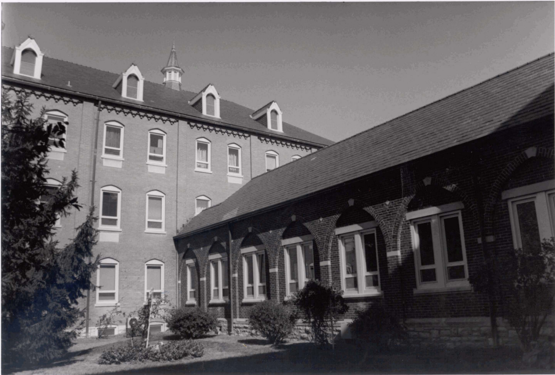
St. Mary's Institute of O'Fallon St. Charles County, MD Photo No. 8
