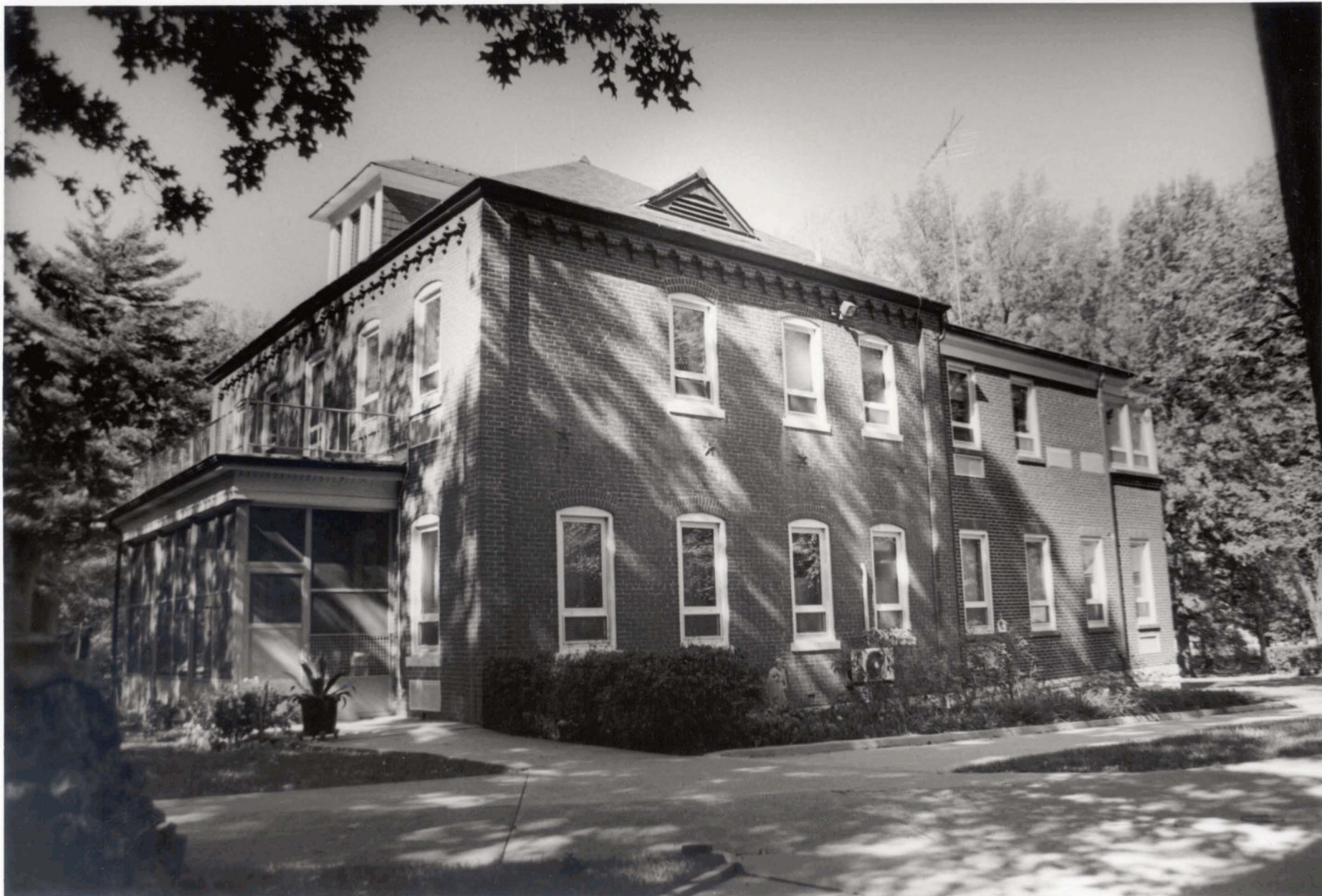
St. Mary's Institute of O'Fallon St. Charles County, MD Photo No. 15
