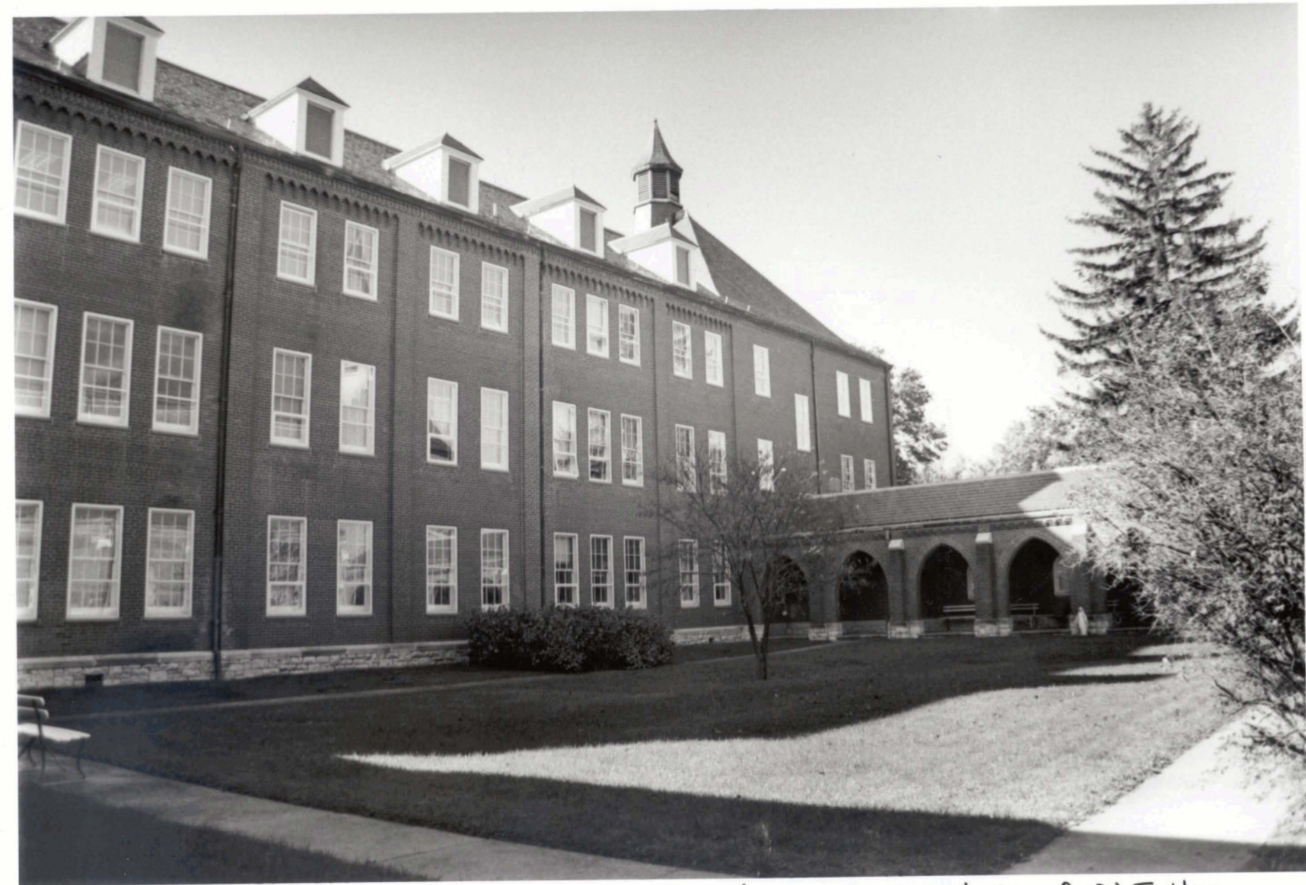
St. Mary's Institute of O'Fallon St. Charles County, MD Photo No. 12
