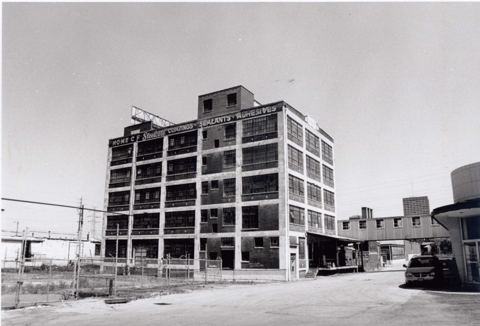
Steelcote Manufacturing Company Paint Factory St. Louis (Independent City), MO Photo # 2
