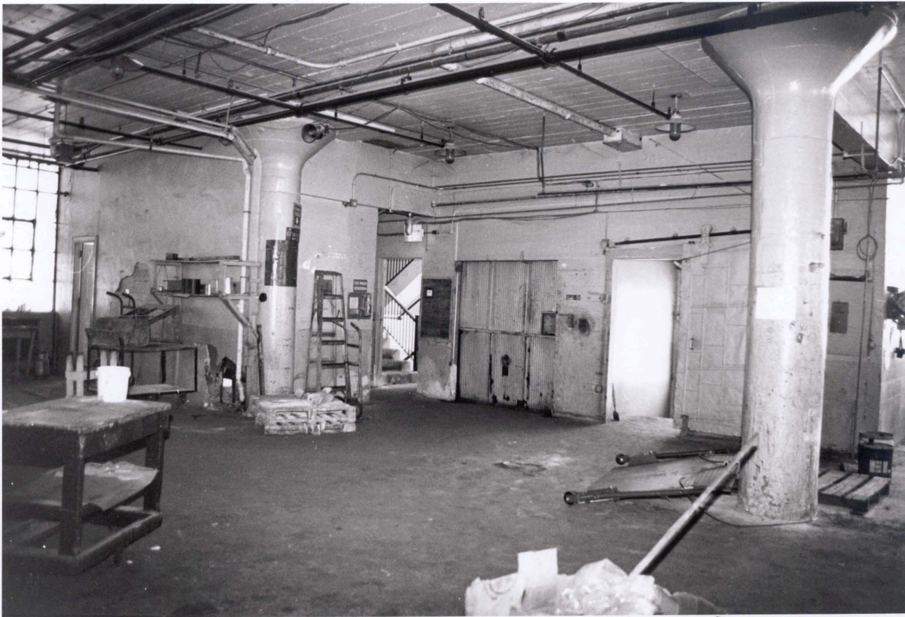
Steelcote Manufacturing Company Paint Factory St. Louis (Independent City), MO Photo # 10
