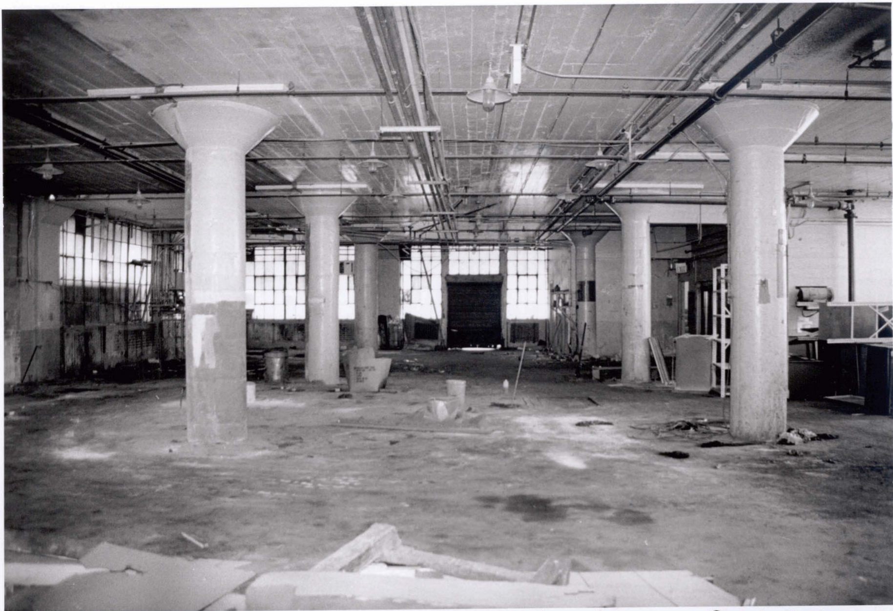
Steelcote Manufacturing Company Paint Factory St. Louis (Independent City), Mo Photo # 9
