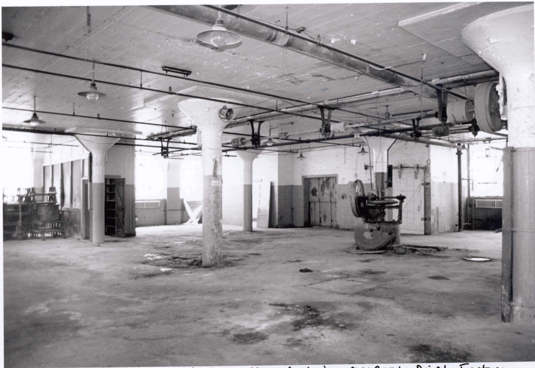
Steelcote Manufacturing Company Paint Factory St. Louis (Independent City), Mo Photo # 13
