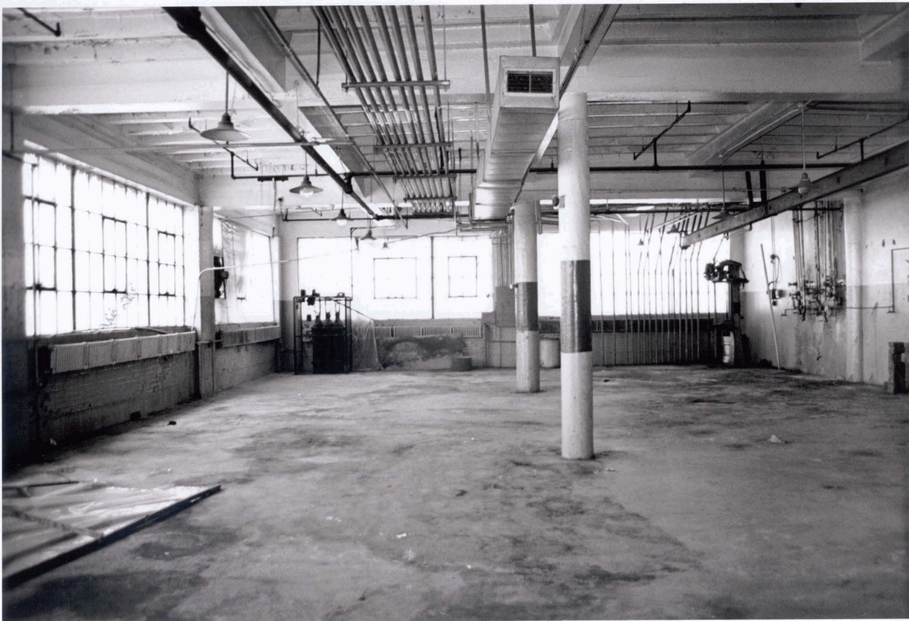
Steelcote Manufacturing Company Paint Factory St. Louis (Independent City), MO Photo # 14
