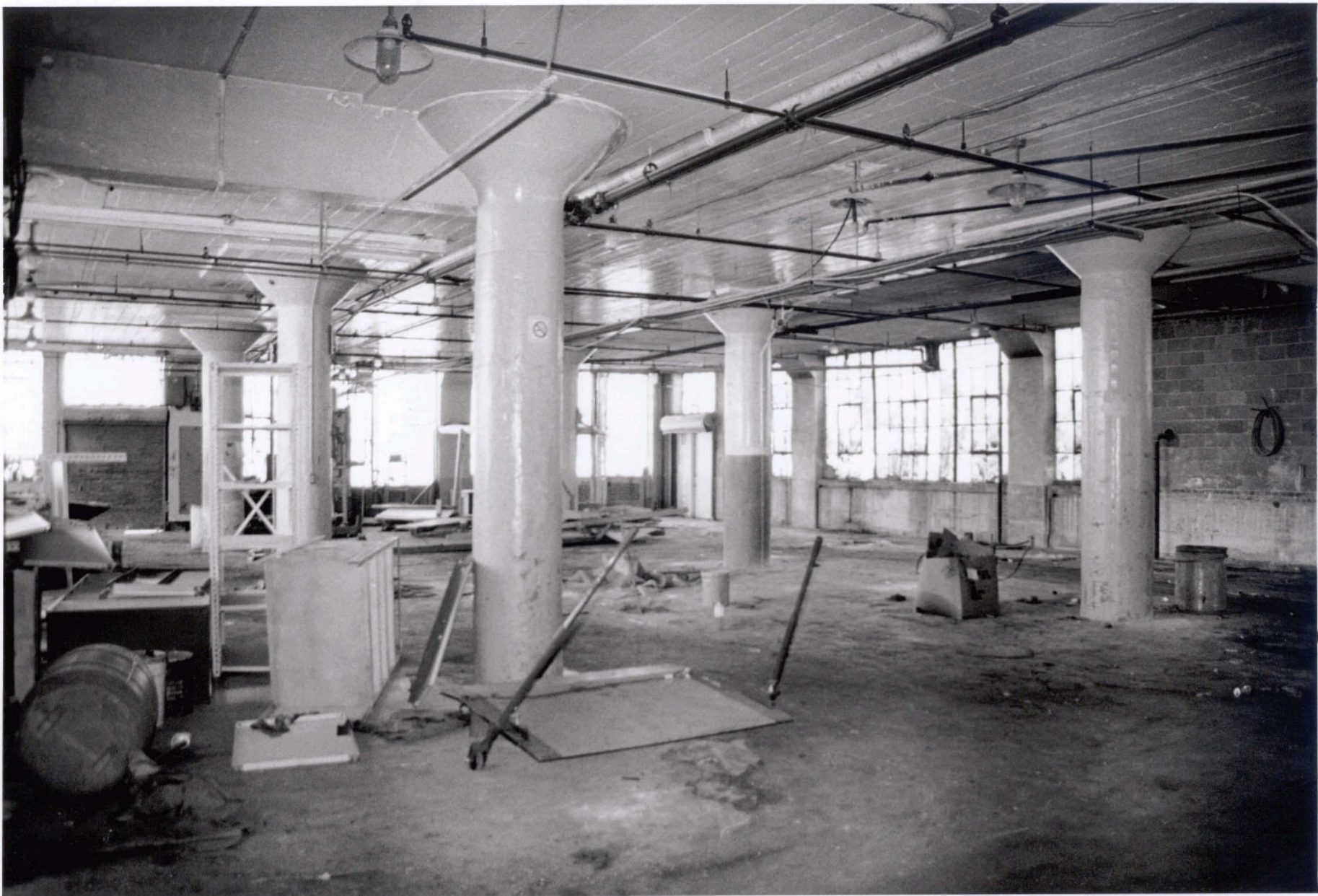
Steelcote Manufacturing Company Paint Factory St. Louis (Independent) City, MO Photo # 7
