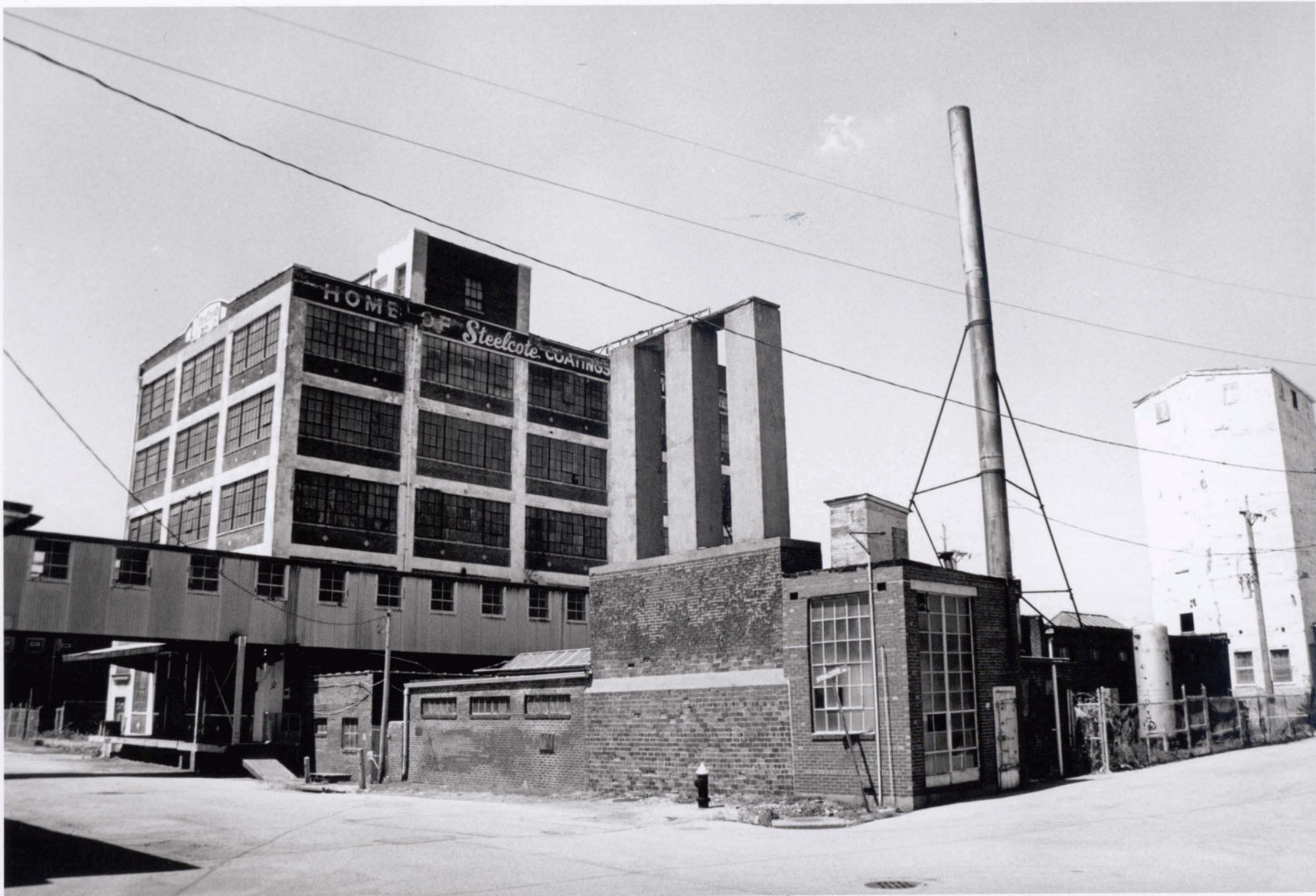
Steelcote Manufacturing Company Paint Factory St. Louis (Independent City), MO Photo # 3
