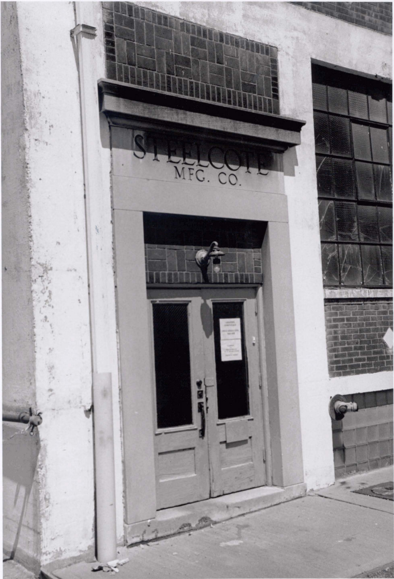
Steelcote Manufacturing Company Paint Factory St. Louis (Independent City), MO Photo # 1
