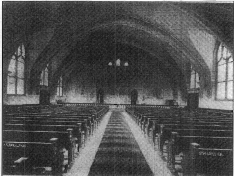
Interior of St. Mark's Church c. 1902.
