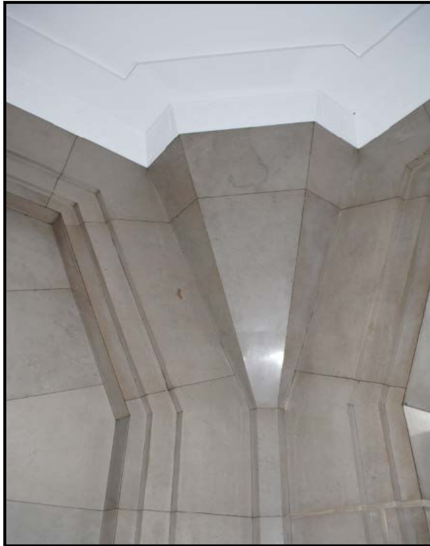
Figures 1A and B (top to bottom): Figure 1A is main lobby geometric marble wall slabs (and ceiling detail); Figure 1B is an example of the cast iron transom panels at the main entry. Source: Matt Bivens, 2014-2016.
