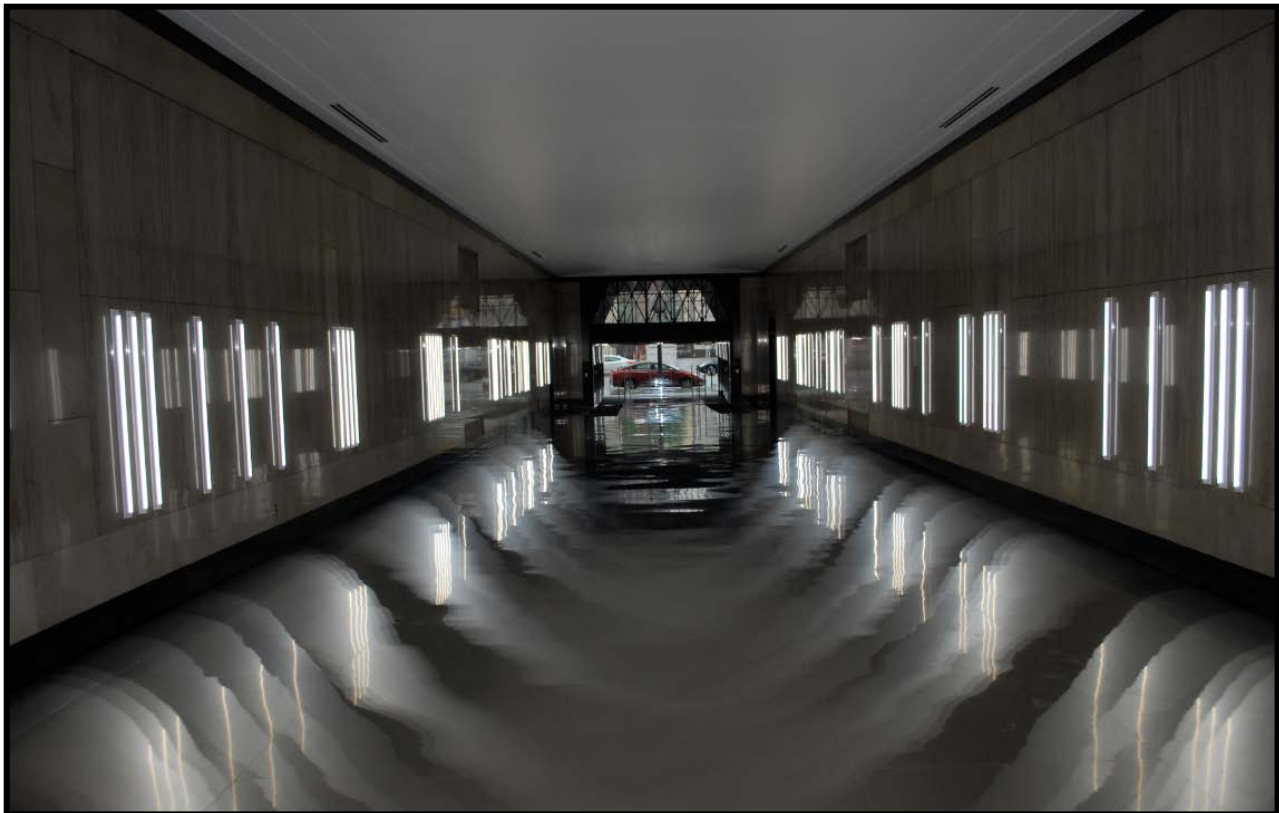
Figure 7: 1 st floor hall looking west towards North Tucker Boulevard. Original terrazzo floor is intact beneath metal floor veneer; vertical lighting is removable but provides light in an otherwise dark corridor. Source: Matt Bivens photograph, 2015.
