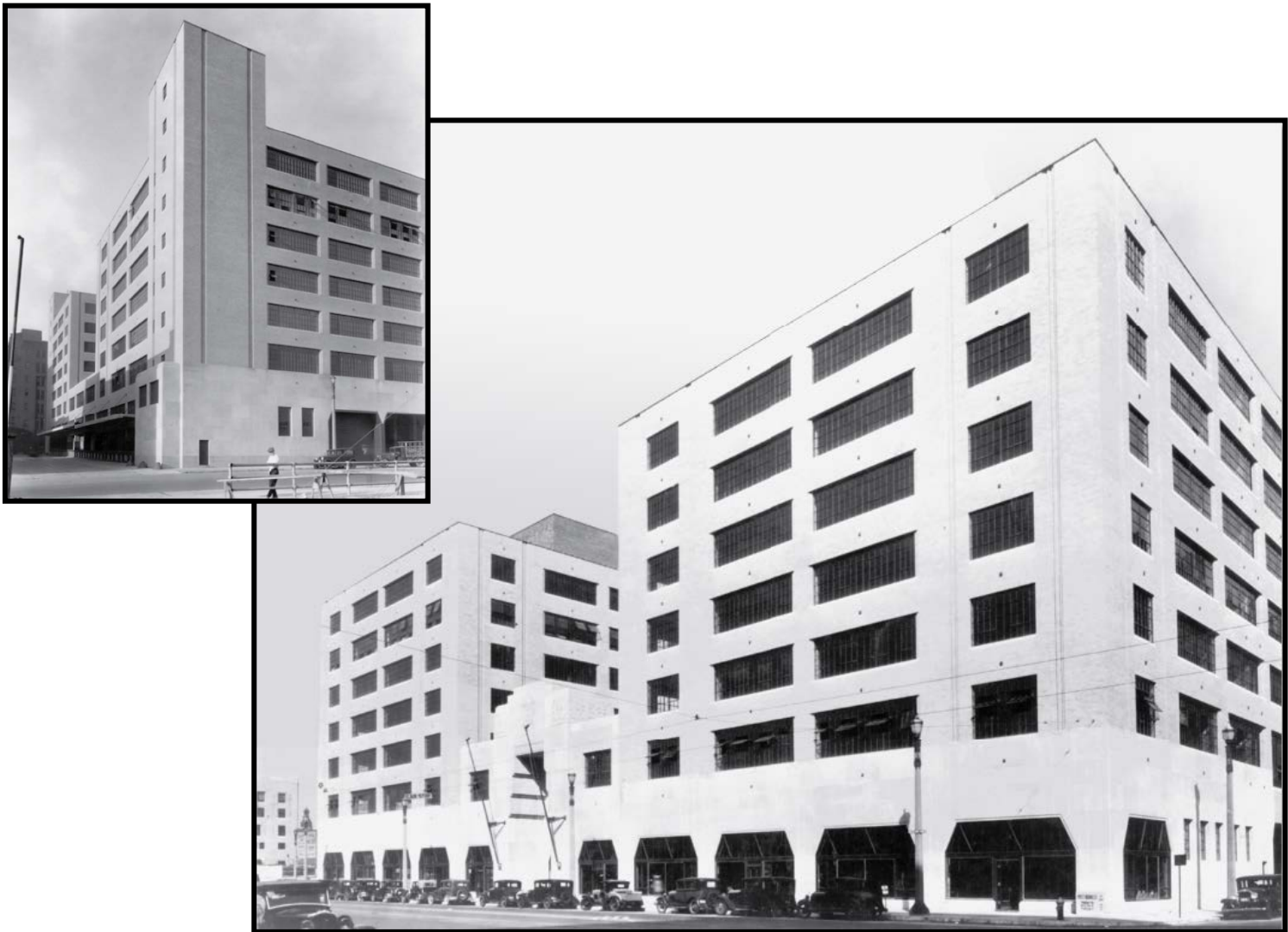
Figure 25: Photographs of completed construction, 1932. The larger image is the primary elevation; the smaller image is the rear, east elevation (left side) with a portion of the north elevation (right side). Source: Collection of Dale Jenkins, Illinois Traction Society.
