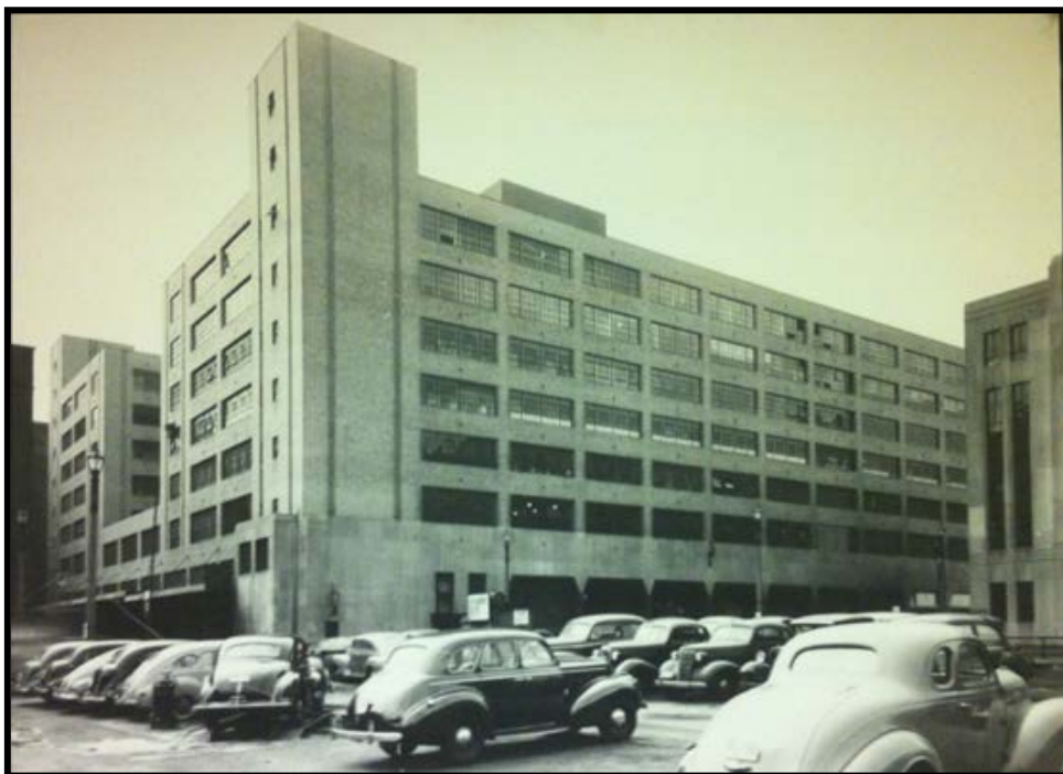
Figure 28: October 1942 photographs of the Midwest Terminal Building, view to southwest (top) and along Lucas alley (bottom) showing loading facilities (color photo is today view, Matt Bivens, 2016). Source: Aeronautical Chart Maintenance Project, St. Louis, Missouri. Exhibits B and C, 10-24-1942.
