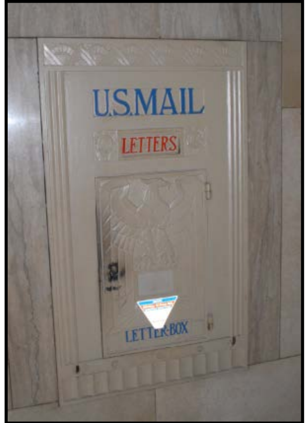
Figures 2A and B (clockwise starting at right): Figure 2A is the original U.S. mail box; and Figure 2B contains 2 examples of the ornamental metal grilles in the lobby. Source: Matt Bivens, 2014-2016.
