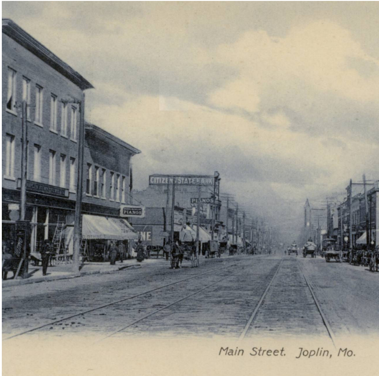
Figure 9: Postcard of Main Street (enlargement), c. 1907 shows 702-704 and the adjoining 706-708 S. Main Street. shortly after construction and occupancy by the Joplin Furniture Company. (From the collection of the Joplin Public Library).
