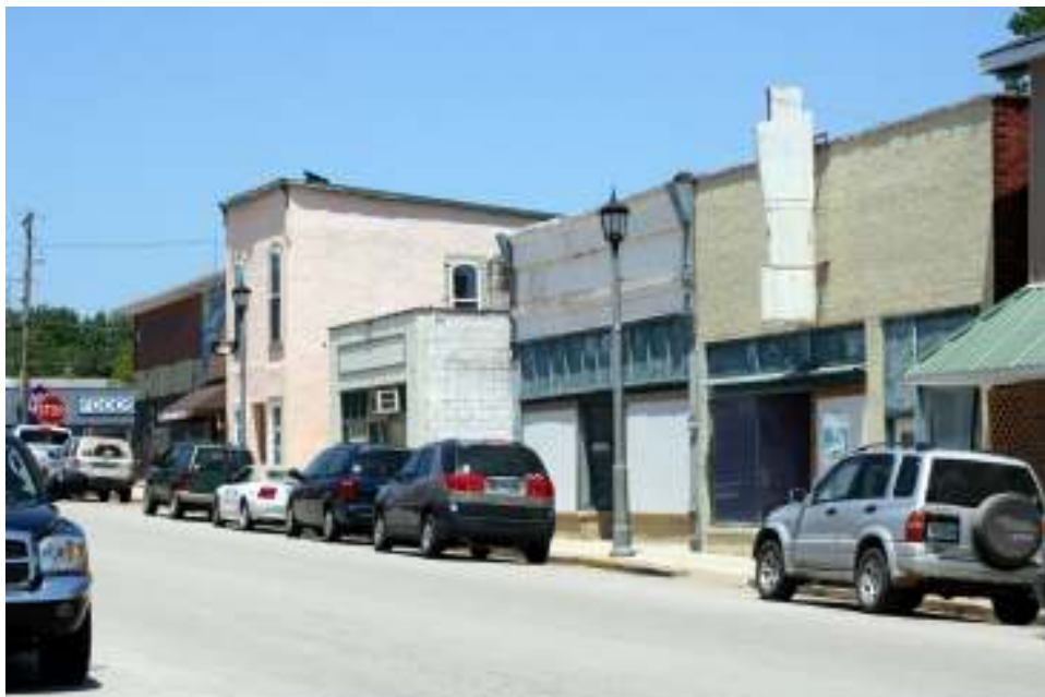
Fig. 18 Streetscape views along N. Smith Street, looking south toward Main Street, lined with examples of Property Type III-A buildings in the downtown commercial district.
