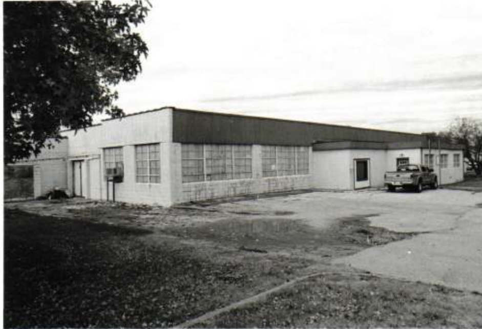
Fig. 14 Industrial variant of the Type III building [photo by Steven E. Mitchell and Mary Aue Mitchell [from 2007 Historic Resource Survey Report ]
