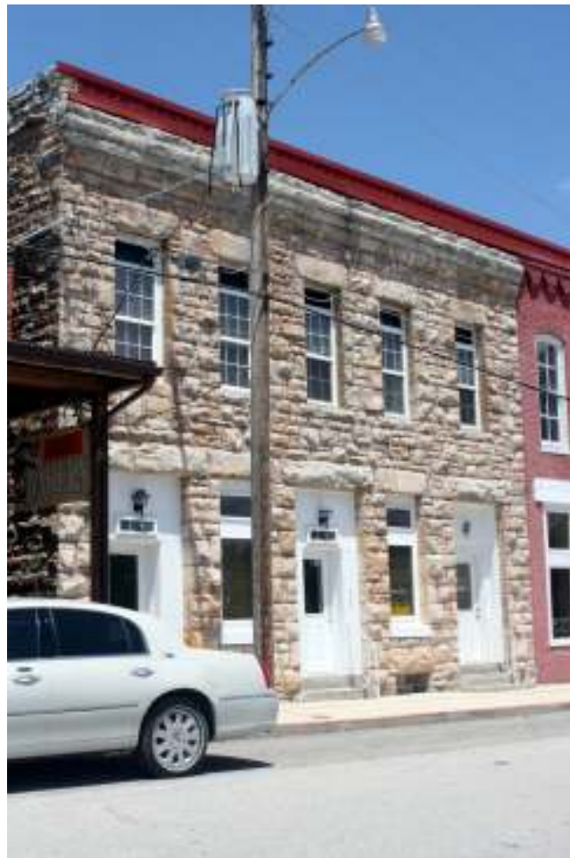
Fig. 13 The 1897 Hotel Grand, an example of a Property Type III building, in this case finished in stone with a metal cornice.
