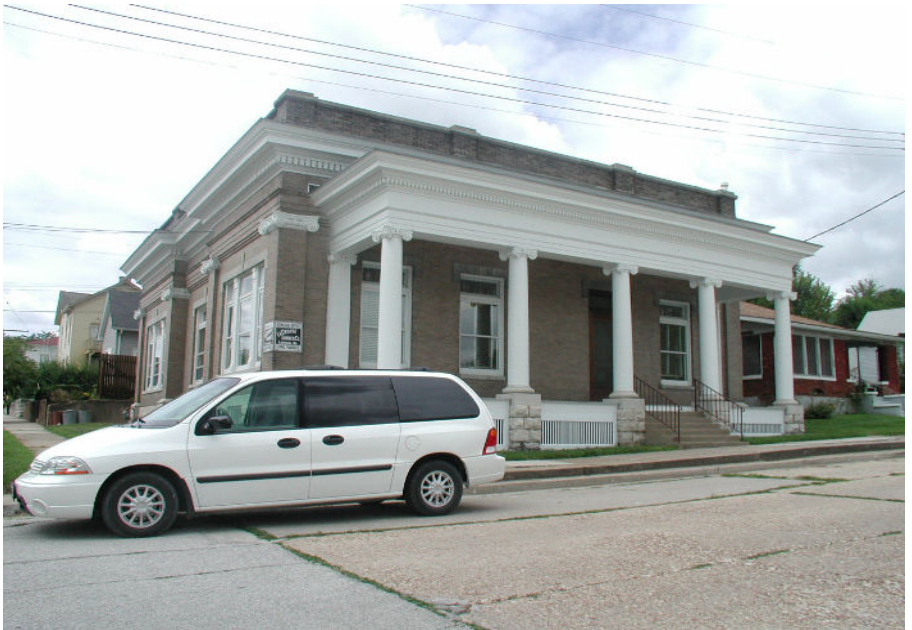
Figure Eighteen. LaCrosse Lumber Company General Offices, 2004.
