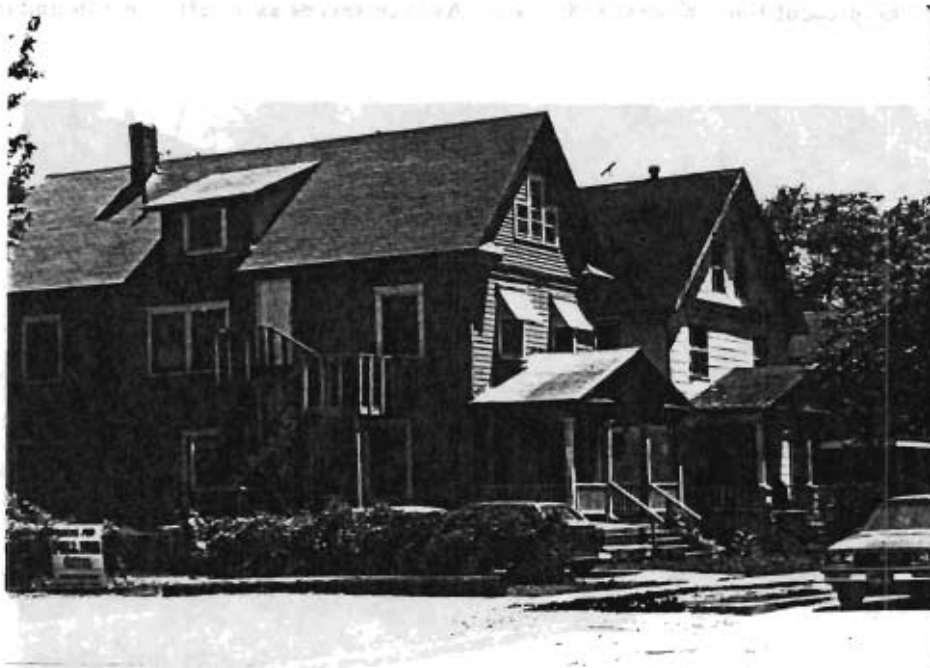
Although the building on the right has false siding and is in poor condition, its retains key design features which contribute to the visual continuity of the potential historic district.
