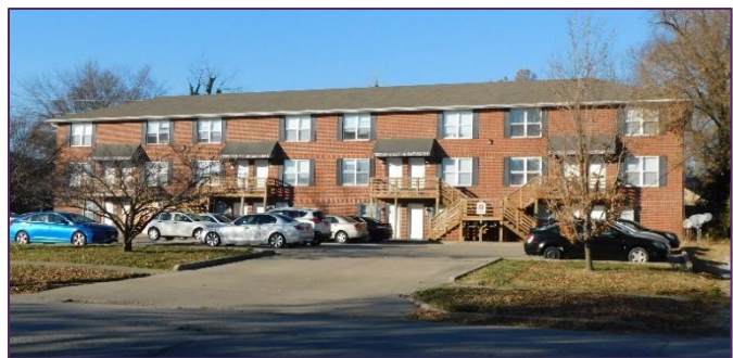
Figure 24: 411 Broad St. - Multifamily
