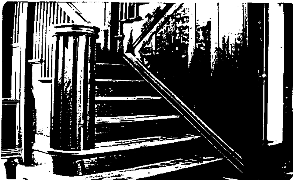
Figure 2: Historic Photograph - Original Central Stairway (Photo - circa 1930s, Patricia Hilkemeyer, Westphalia, MO)
