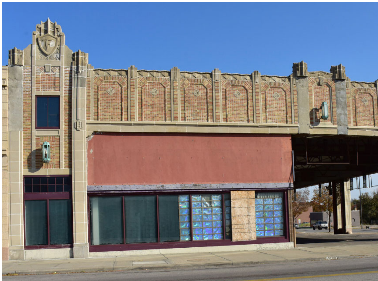
Figure 11. West elevation, showing non-historic windows. Note the light fixtures, added after 1930; they have been removed as of December 2020. Source: Brad Finch, November 2019.
